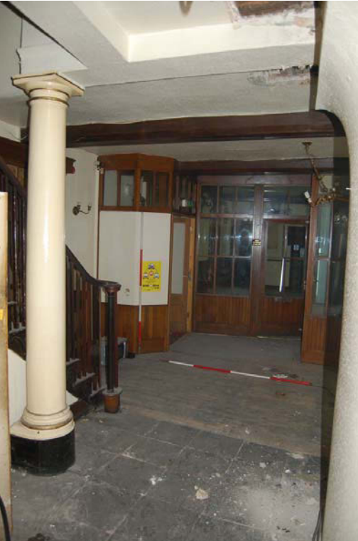
Plate 26: Room G5 looking north.
