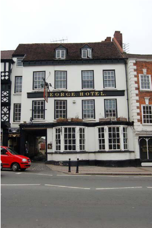
Plate 4: Street Elevation, No. 63 Load St.
