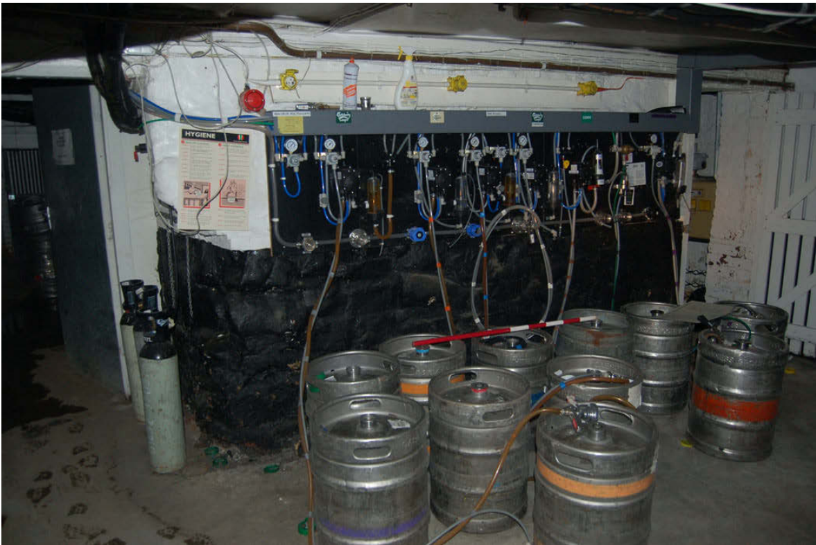
Plate 16: Basement room B1 looking south; red sandstone stack footing.
