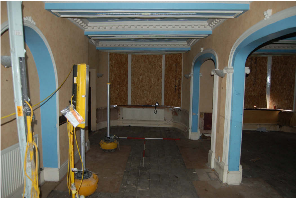
Plate 18: Room G1 (east), looking south.
