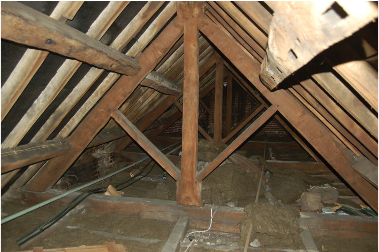
Plate 76: Room F19 King-post roof structure looking south. Note re-used timbers.
