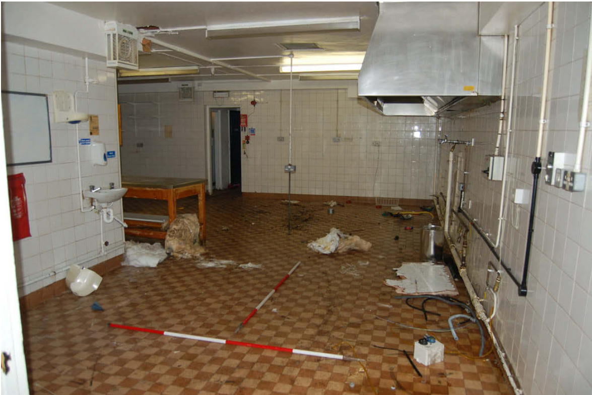
Plate 32: Room G12 (Kitchen) looking north.
