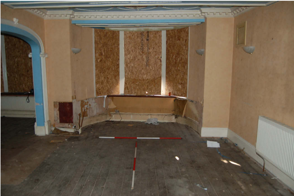
Plate 17: Room G1 (west), looking south.
