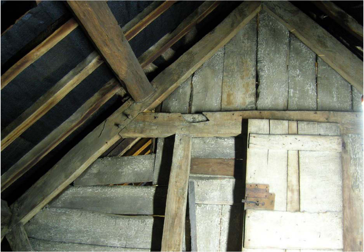
Plate 69: Truss 3, taken from the north, note reused collar. (Photo: Nottingham Tree Ring Dating Laboratory).
