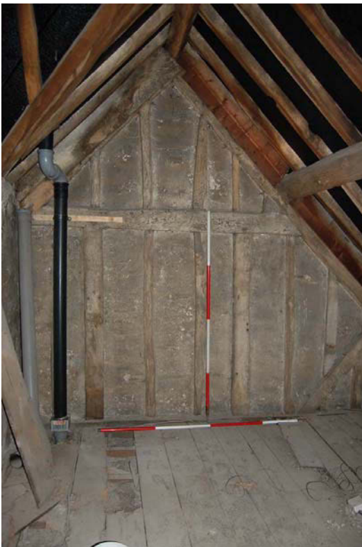
Plate 67: Room T9, east wall. head/cill.
