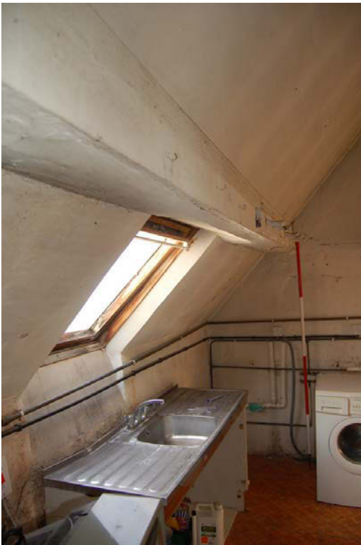
Plate 57: Room S17 looking north.
