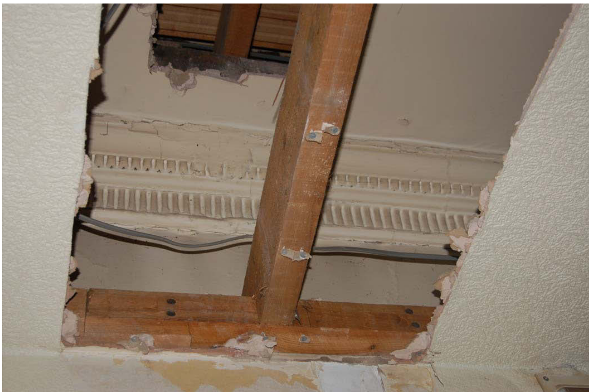
Plate 31: Room G11; former cornice detail above inserted ceiling.
