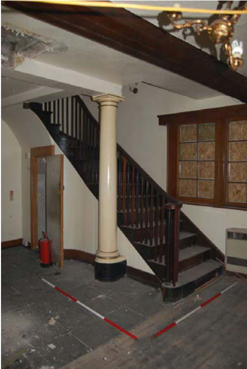
Plate 27: Room G5 base of stair B.
