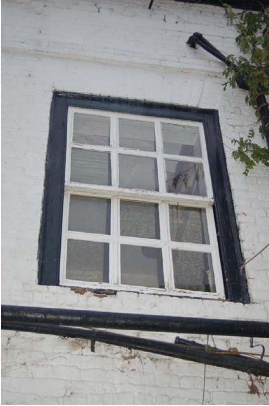
Plate 8: Exposed sash-box / broad glazing bars to primary window Room F.xx
