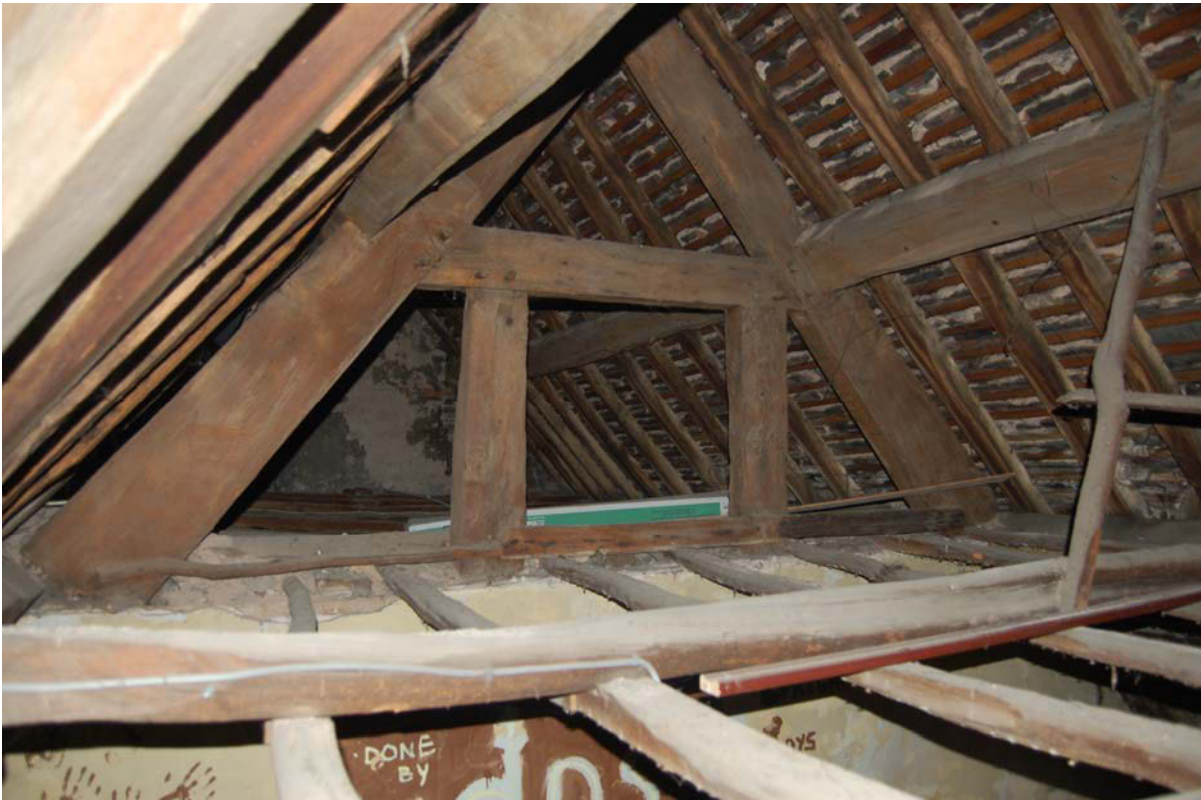
Plate 59 Truss 2, taken from the west.
