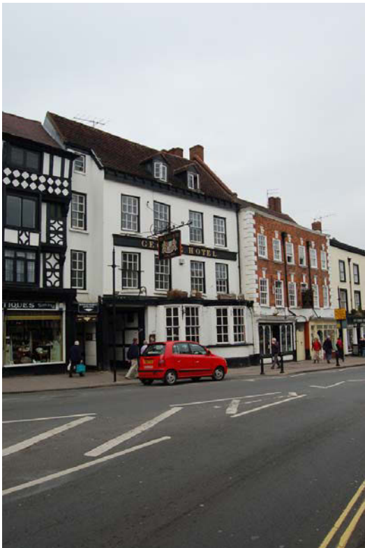
Plate 2: Street elevation from south-west.
