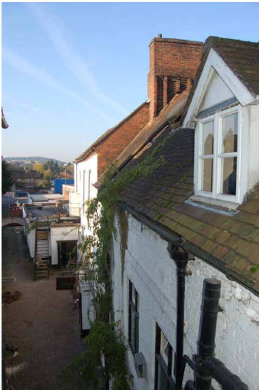
Plate 7: No.63, rear ranges looking north.
