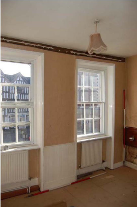
Plate 44: Room F9 looking south-west.
