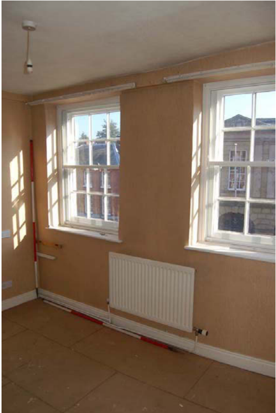
Plate 54: Room S5 looking north-west.
