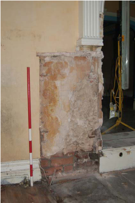
Plate 21: Room G1, change in brickwork.
