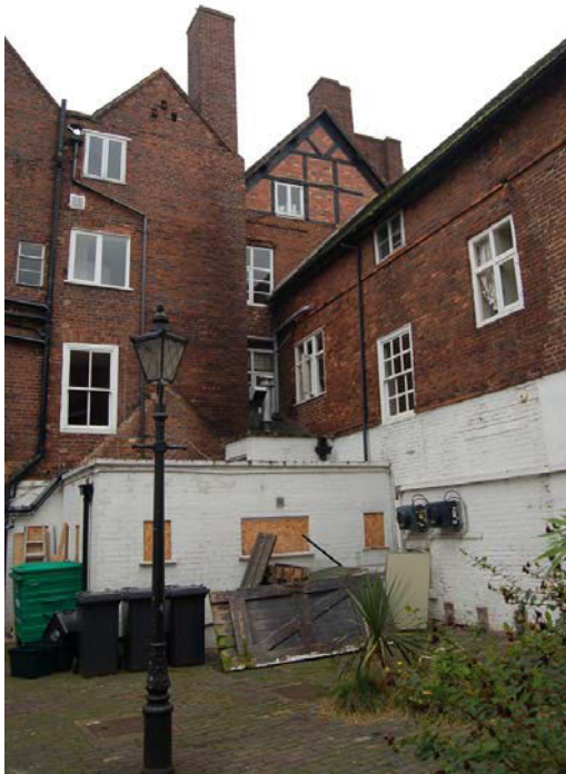
Plate 11: No.63/64; rear (north) elevation and east No. 63 rear range (right). (right).
