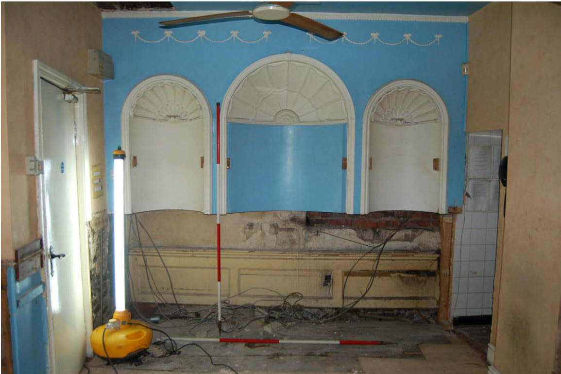
Plate 19: Room G1 north wall, note former dado panel.
