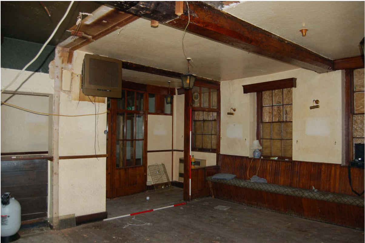
Plate 28: Room G10 looking south-west. Note stop chamfered beam.
