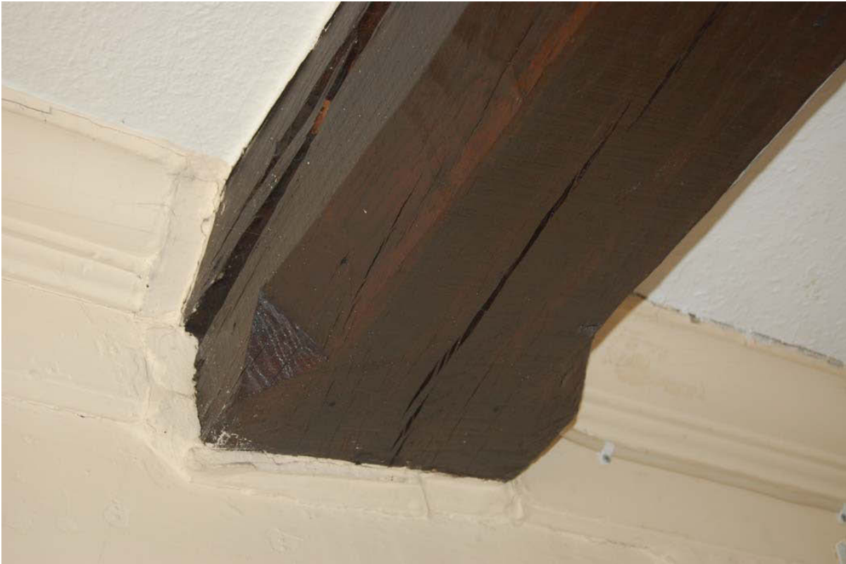
Plate 43: Room F6, detail of stop-chamfered ceiling beam.
