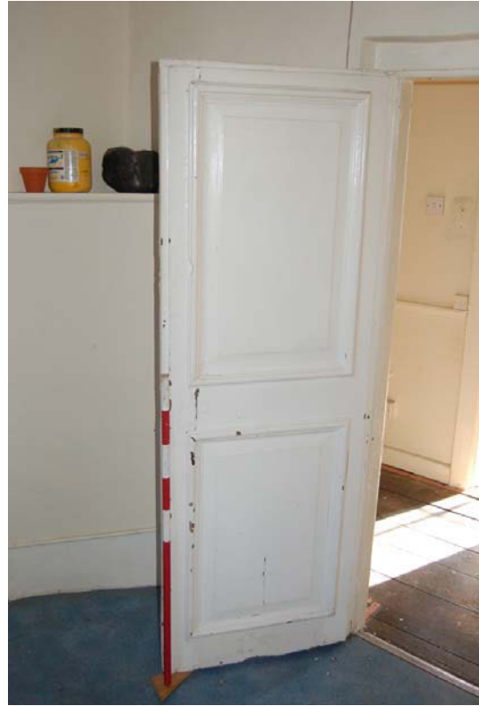
Plate 39: Room F5 bolection panelled door.
