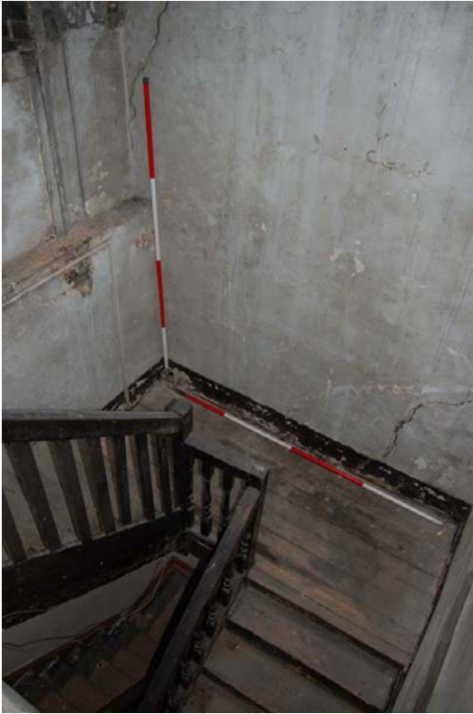
Plate 65 Stair A (2 nd - 3 rd floor).
