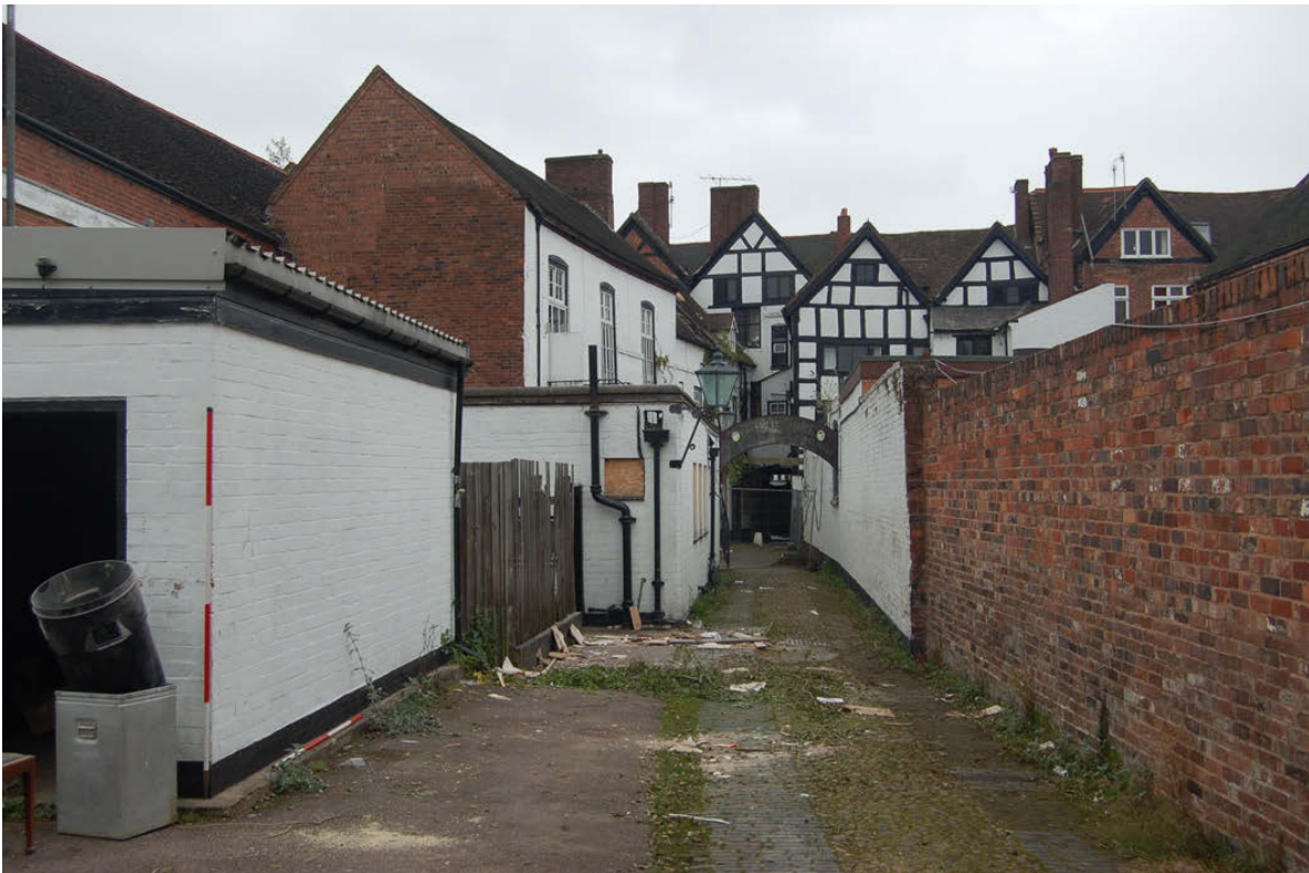
Plate 10: Modern garages (left) to north of Assembly Room (note rebuild in Assembly Room gable).
