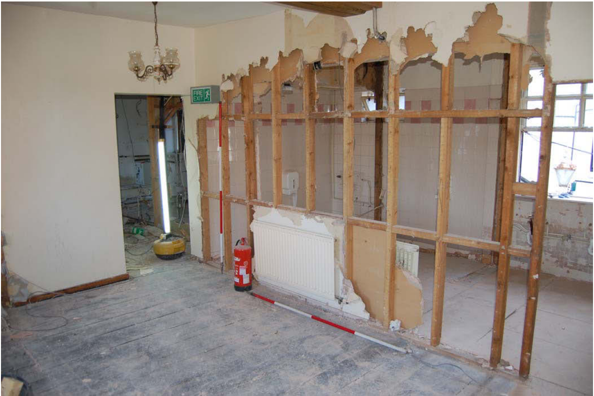
Plate 47: Room F14/ 15/16 - 1960s studwork partitions during removal.
