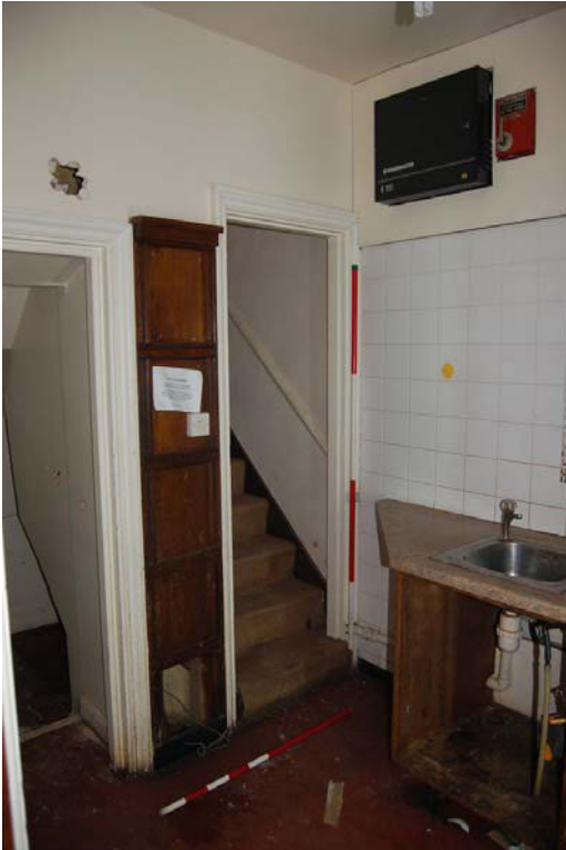
Plate 25: Room G3; base of stair A.
