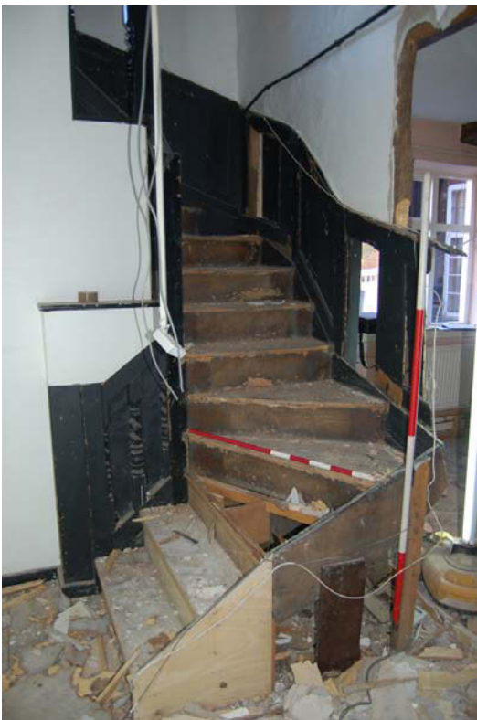
Plate 48: Late C17th open-well stair (C) with twisted balusters.
