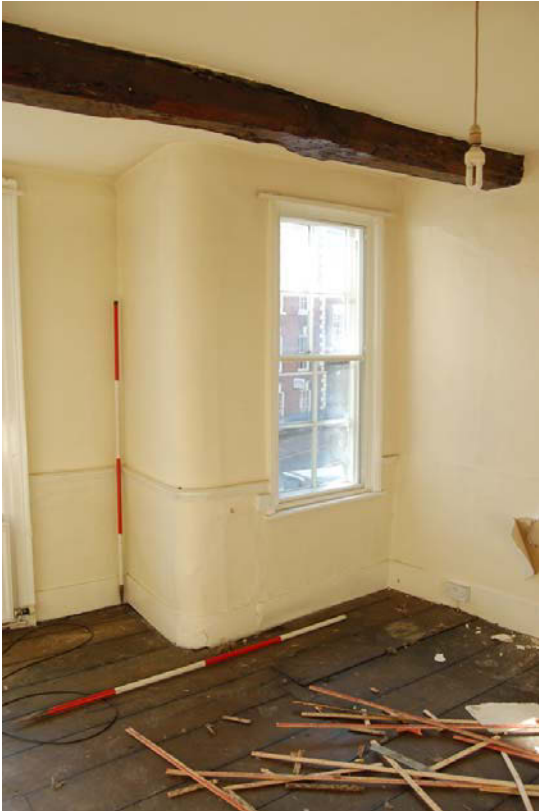
Plate 34: Room F1 looking south-west.
