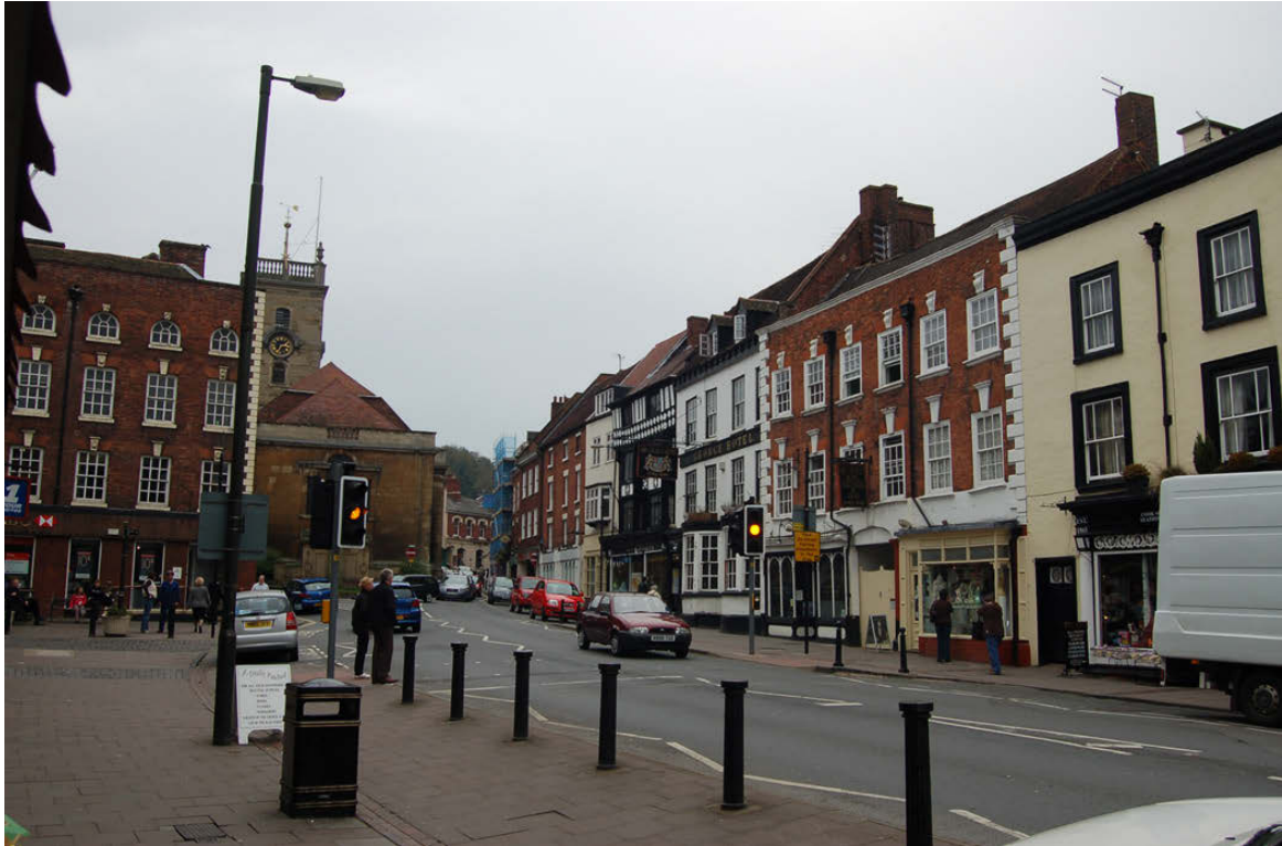
Plate 1: Load Street streetscape; view from south-east, George Hotel to centre right of photo.
