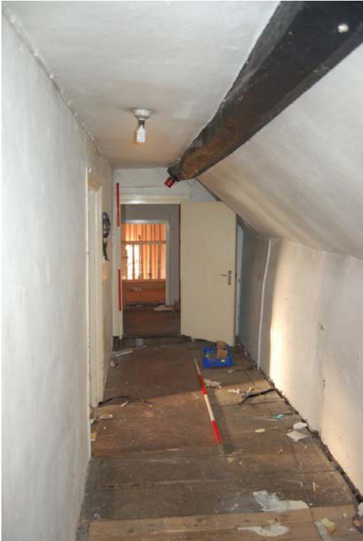
Plate 56: Room S16 looking north.
