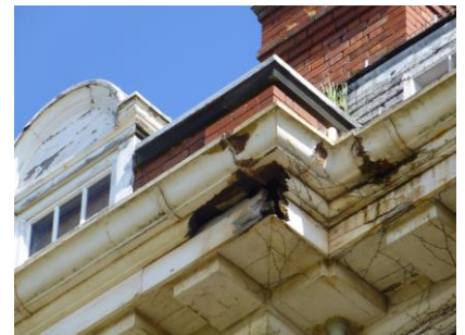
Neville House: cornice detailing in timber
