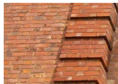
The two types of brick used on Neville House are subtly different. The quoins are in a slightly smoother and more regular brick.
