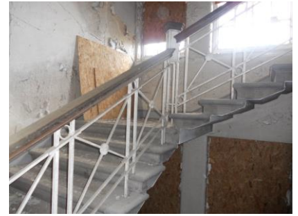
Neville House: the elegant cantilevered stone staircase is to be retained in the current proposals.
