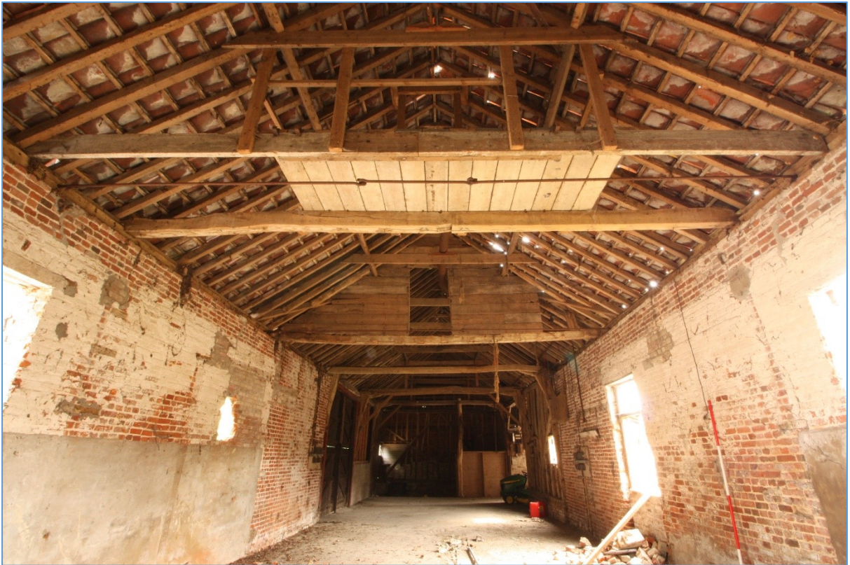
Plate 32. Interior view of Barn 2, looking north, showing the tie beams and raised platforms in the roof space.
