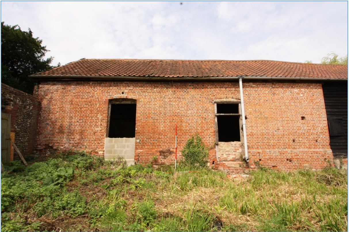
Plate 24. Barn 2's eastern elevation, showing the two partially blocked doorways and the junction with Barn 1..
