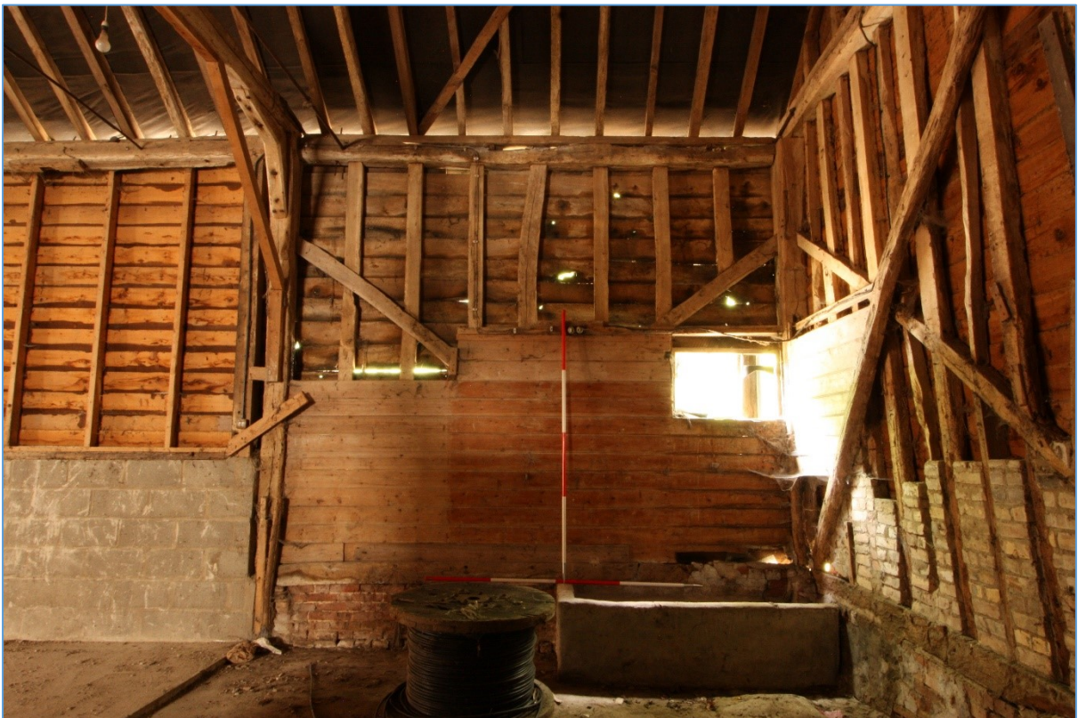
Plate 8. Interior view of the northern bay of Barn 1's western elevation, showing the remaining panel of studwork.
