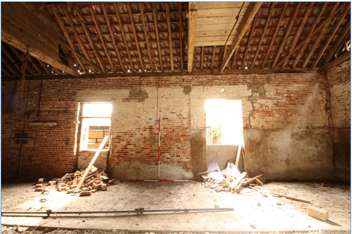
Plate 25. Interior view of Barn 2's eastern elevation, showing the two partially blocked doorways.
