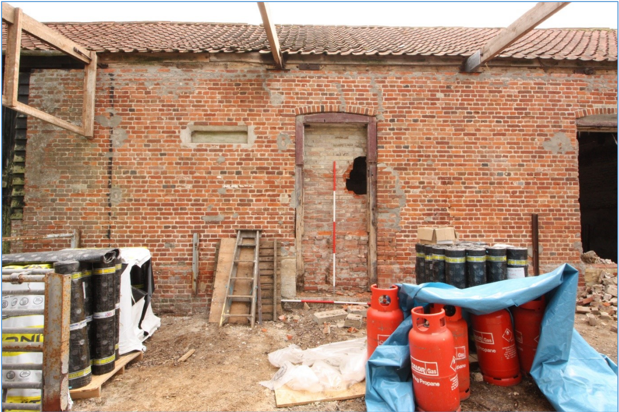
Plate 30. Barn 2's western elevation, central section, showing the partially unblocked northern doorway and associated blocked window.
