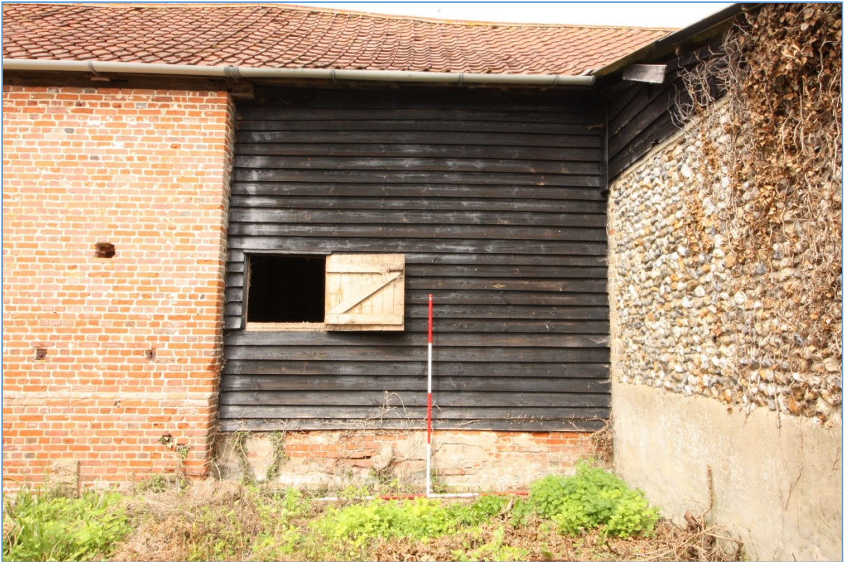
Plate 13. The southern bay of Barn 1's eastern elevation, showing the outward-opening hatch.
