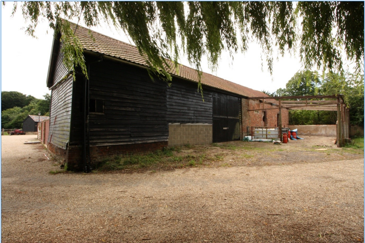
Plate 3. General view of the barn from the north-west, showing the weatherboarded northern end (Barn 1) and the brick-built southern end of the structure (Barn 2).
