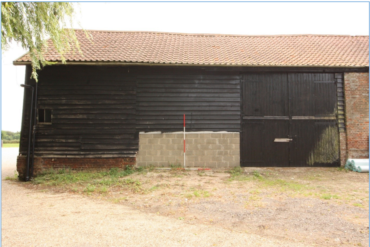
Plate 6. Barn 1's western elevation, showing the blocked-up location of the former western doorway and its modern replacement.
