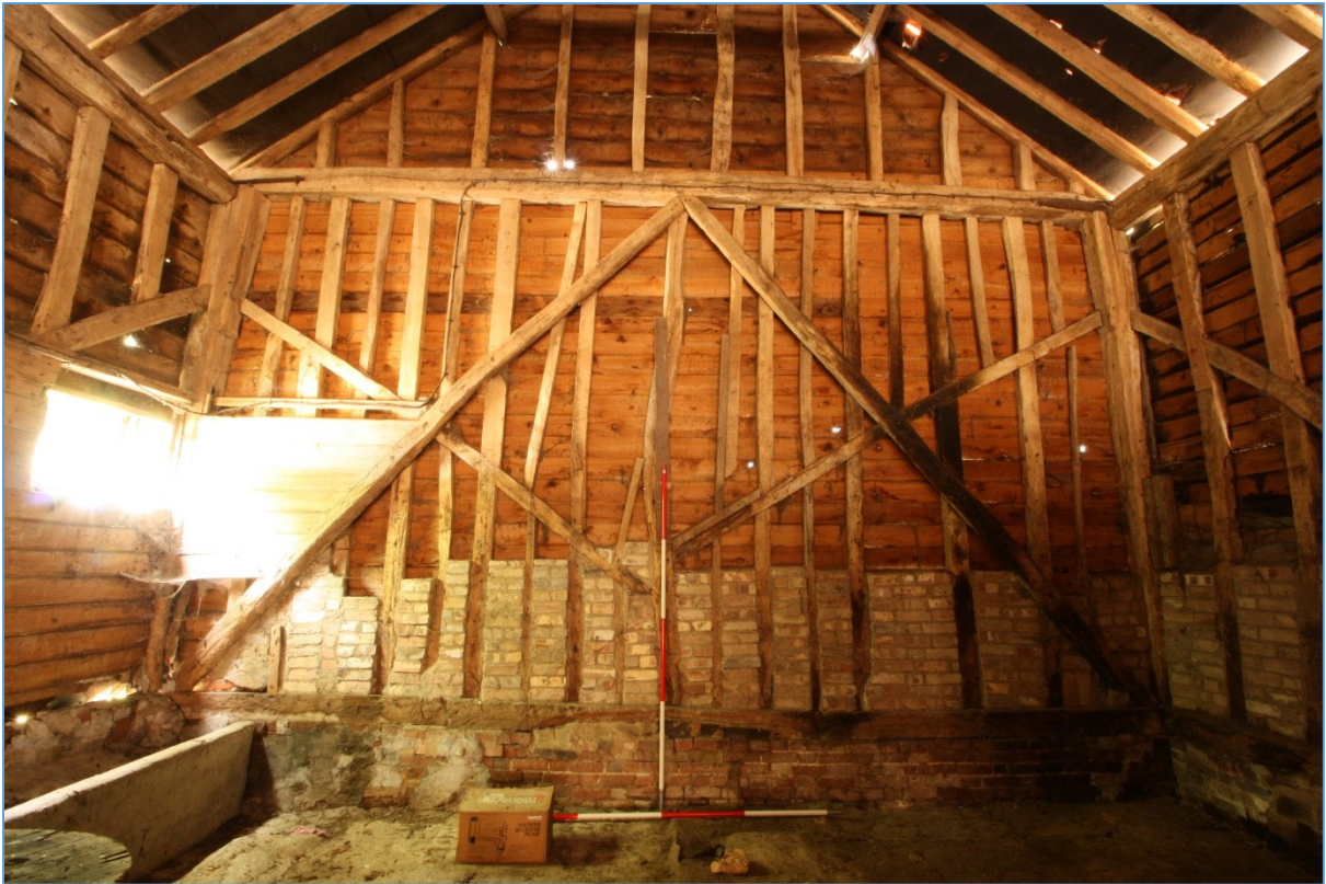
Plate 10. Interior view of Barn 1's northern elevation, showing the remaining panel of timber studwork.
