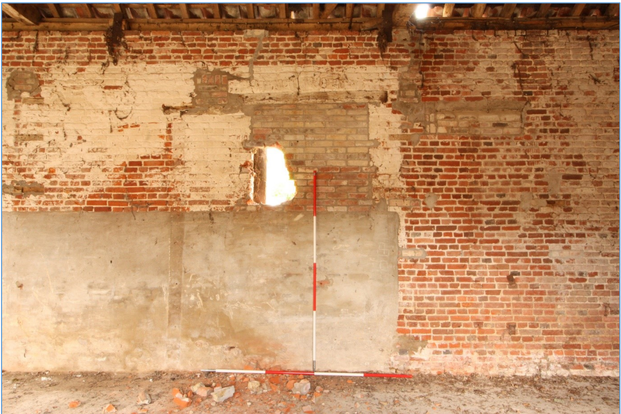
Plate 31. Interior view of Barn 2's western elevation, central section, showing the partially unblocked northern doorway and associated blocked window.
