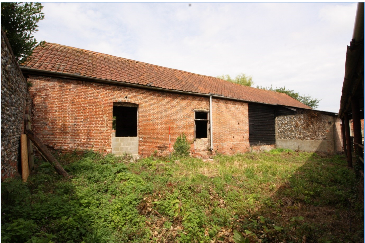
Plate 4. General view of the barn from the south-east, showing the brick-built southern end of the building (Barn 2) with the weatherboarding and brick-and-flint outshot extension of Barn 1 beyond.
