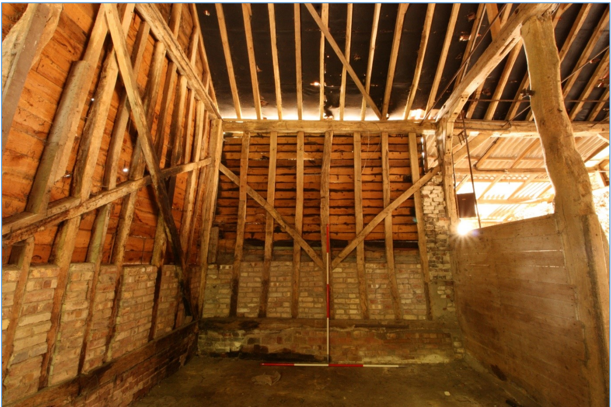
Plate 12. Interior view of the northern bay of Barn 1's eastern elevation, showing the remaining panel of studwork.
