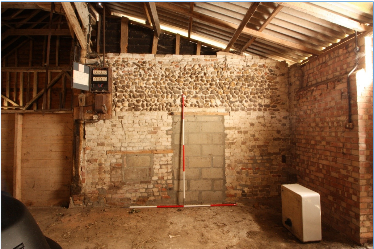
Plate 16. Interior view of the northern elevation of the outshot extension, showing the blocked doorway.
