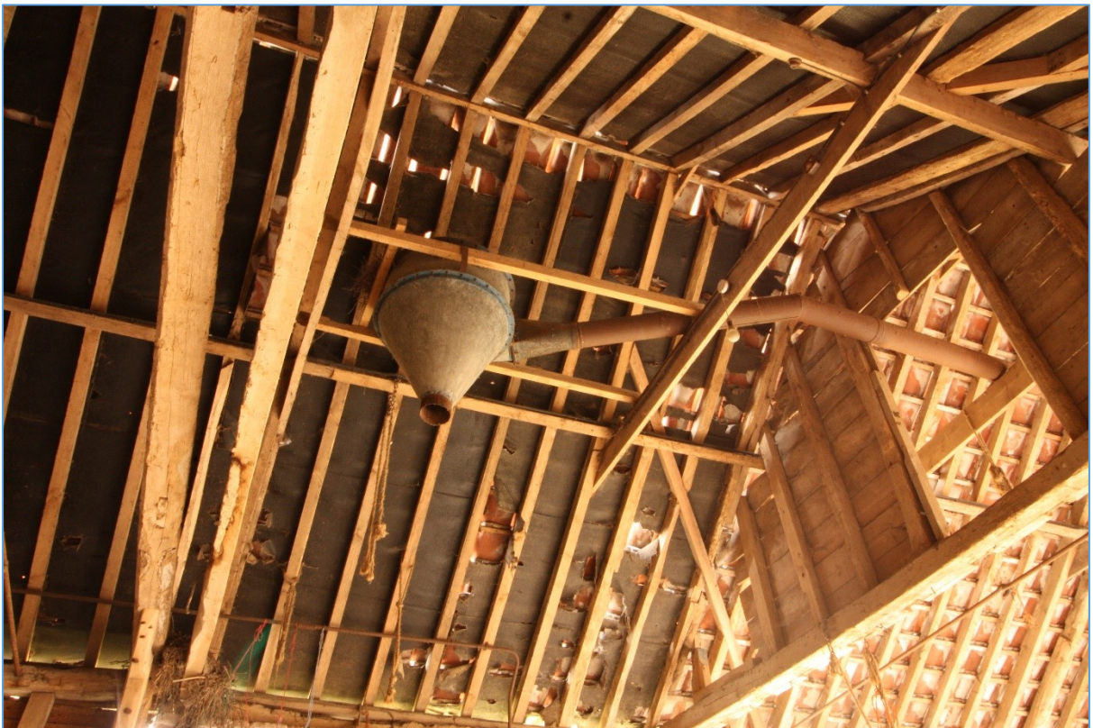
Plate 33. Detail of the silo-related pipework and funnelling still present in the roof space of Barn 2.
