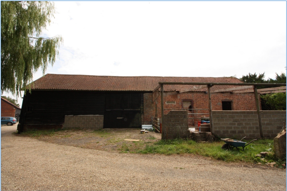
Plate 5. General view of the western elevation of the barn, showing the clear division between the construction of Barn 1 and Barn 2 and the single pantiled roof of the building.
