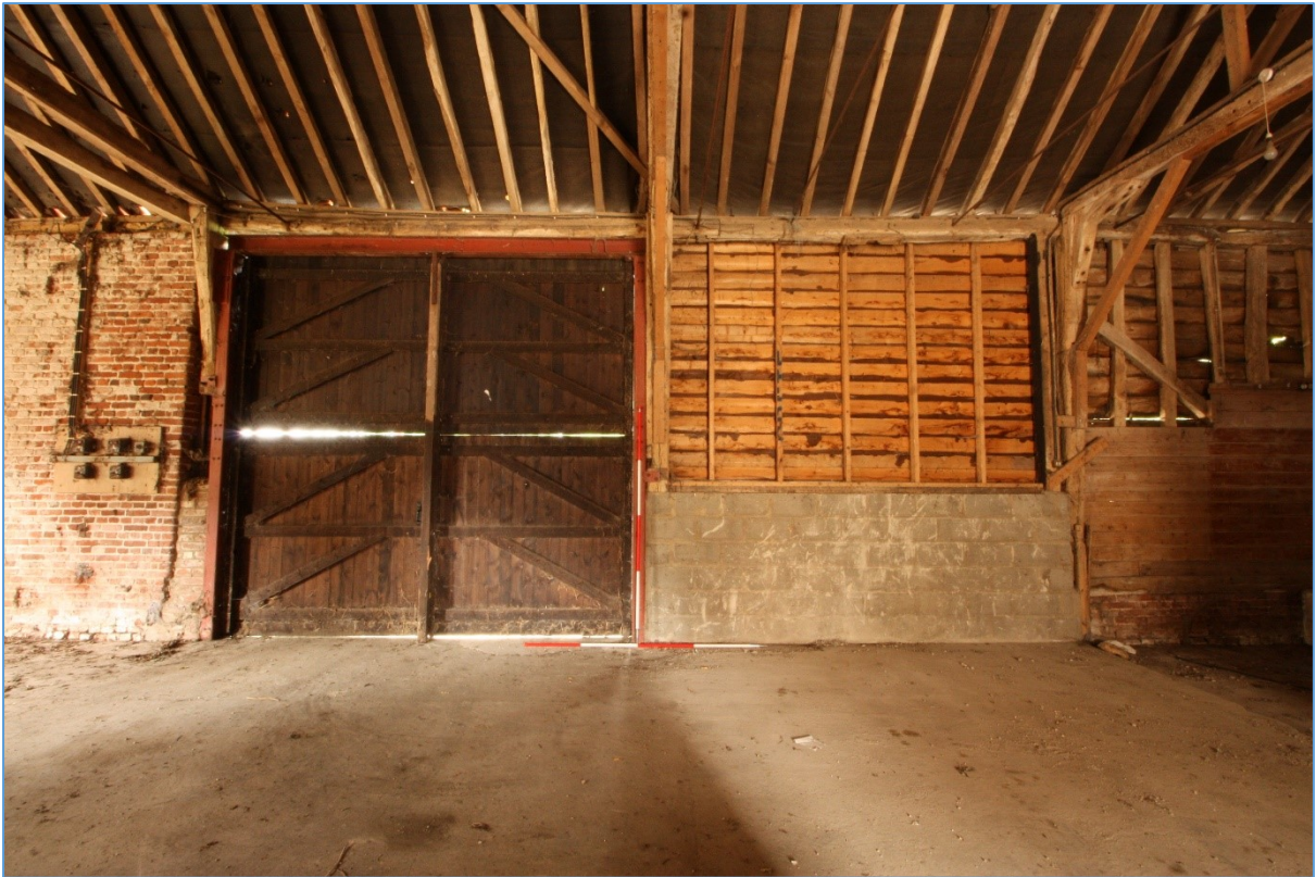
Plate 7. Interior view of the Barn 1's western elevation, showing the blocked-up location of the former western doorway and its modern replacement.
