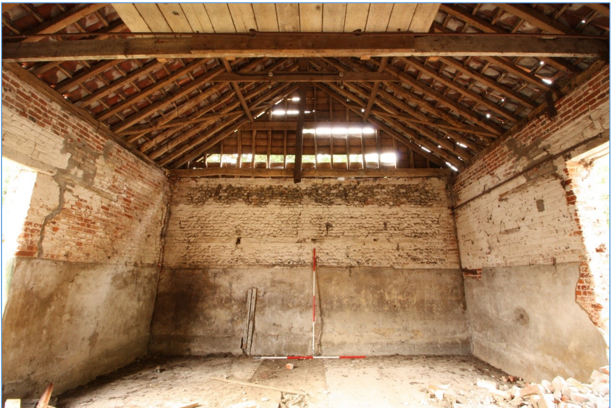
Plate 27. Interior view of Barn 2's southern elevation, showing the extent of the protective render.
