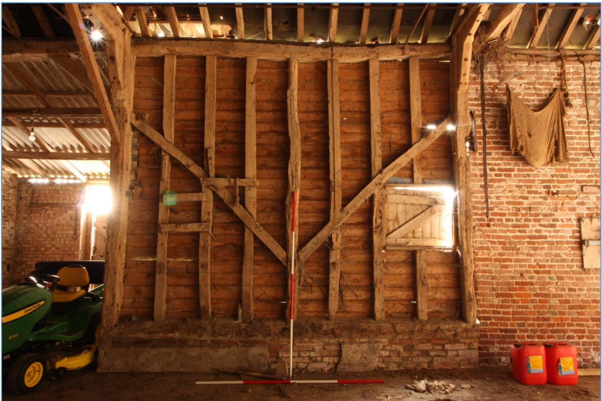
Plate 14. Interior view of the southern bay of Barn 1's eastern elevation, showing the remaining panel of studwork.
