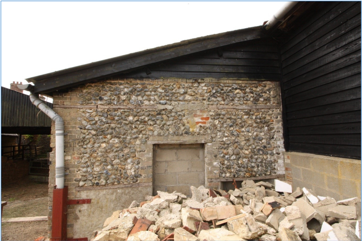
Plate 15. The northern elevation of the outshot extension, showing the blocked doorway.
