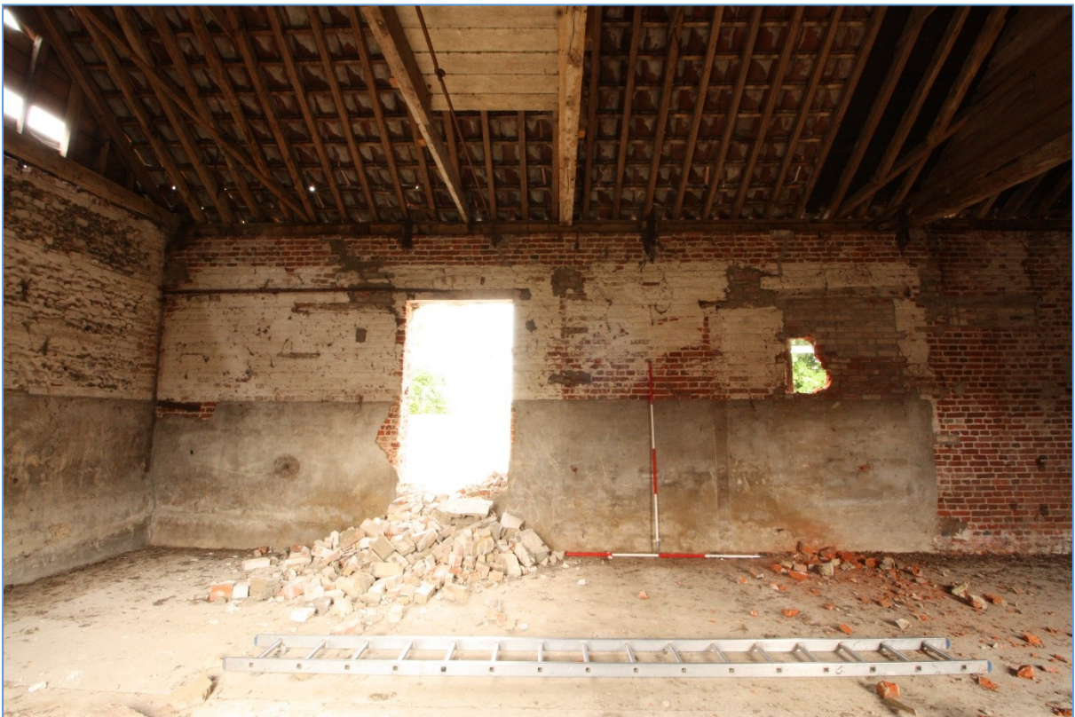
Plate 29. Interior view of Barn 2's western elevation, showing the reopened southern doorway and partially unblocked northern doorway.
