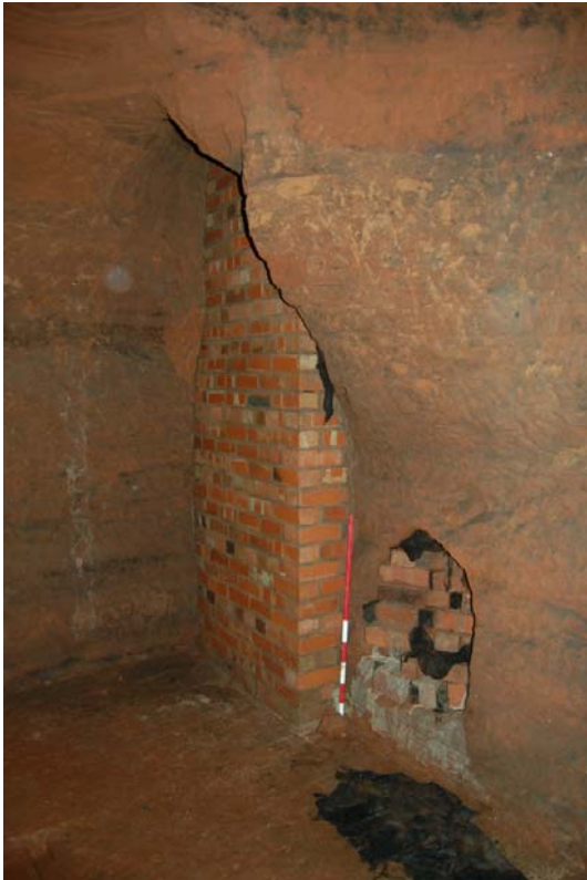
Plate 56: N2, 'Utopia' brick pier at NE angle.
