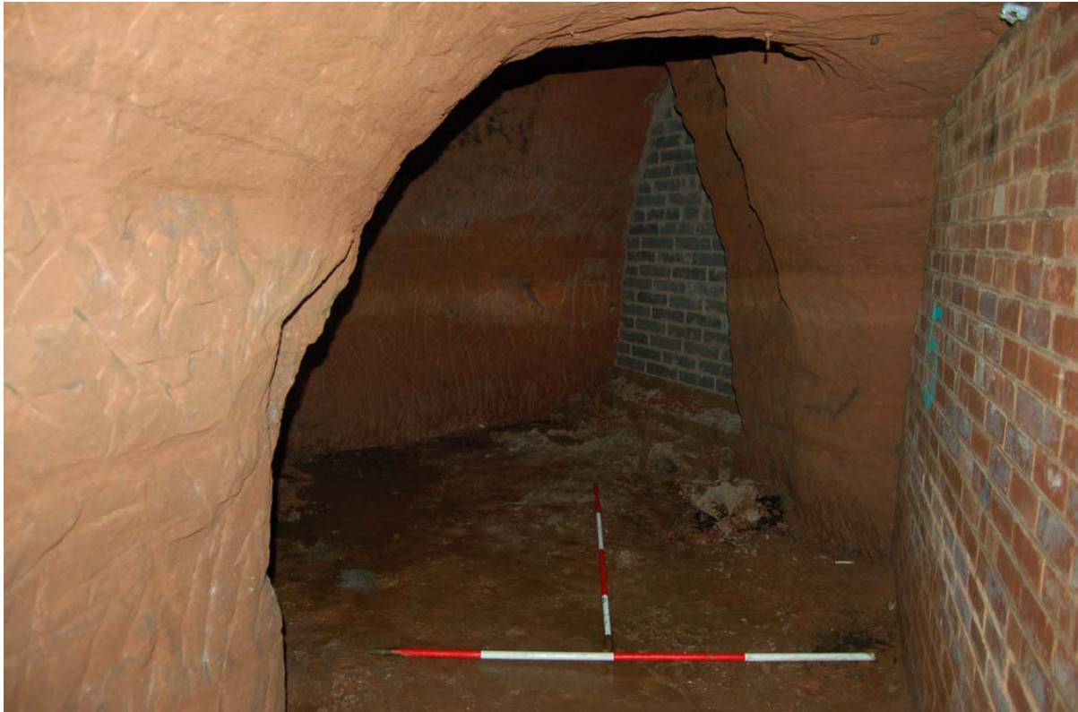
Plate 25: Secondary tunnel between S2 and S1, WW2 brickwork wall to right.
