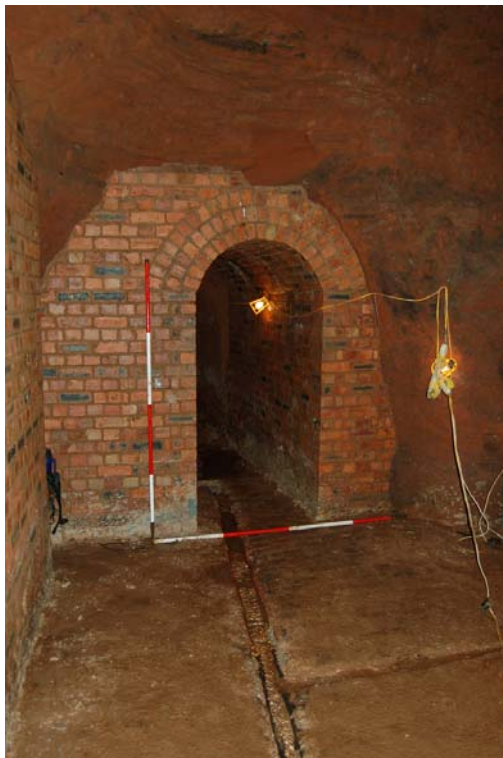
Plate 5: WW2 brickwork at west entrance, arch to entrance tunnel (→E).
