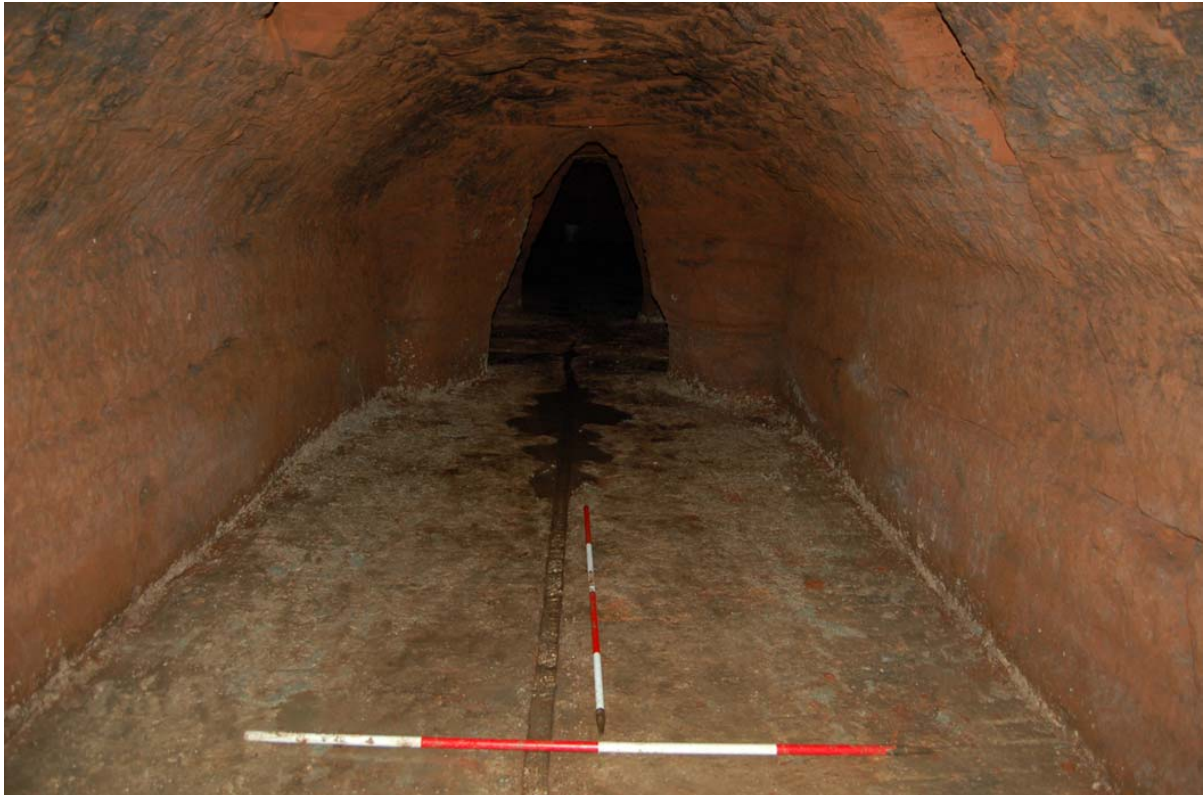
Plate 61: Chamber N4, looking south.
