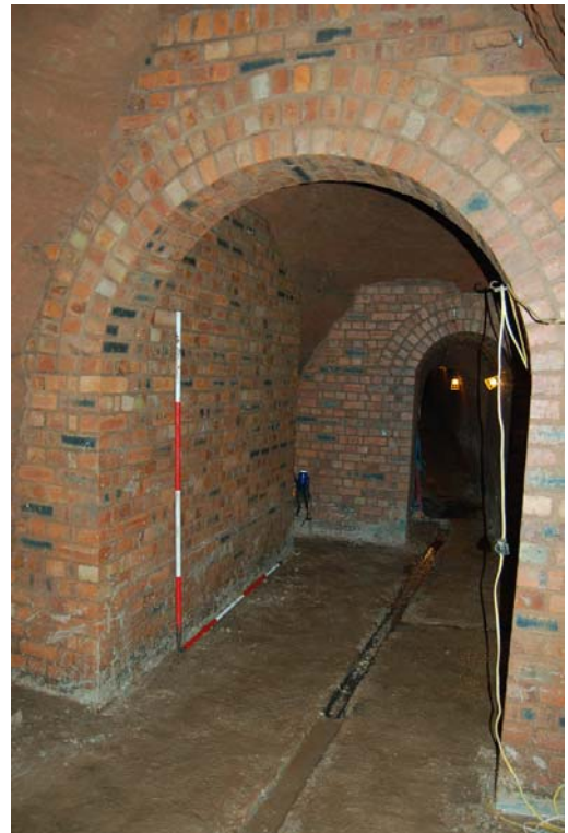
Plate 6: WW2 brickwork at west entrance, arch to Main Gallery (→E).
