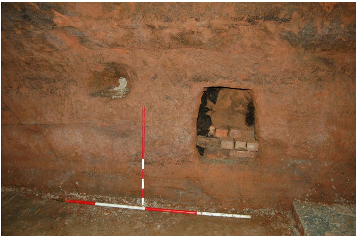
Plate 62: Chamber N4, west wall: side tunnel formerly connecting to Chamber N3.
