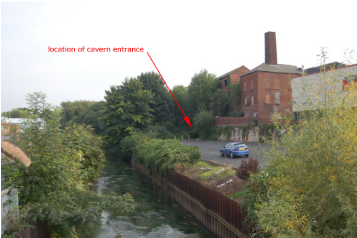
Plate 1: Location of main cavern complex entrance from the north.
