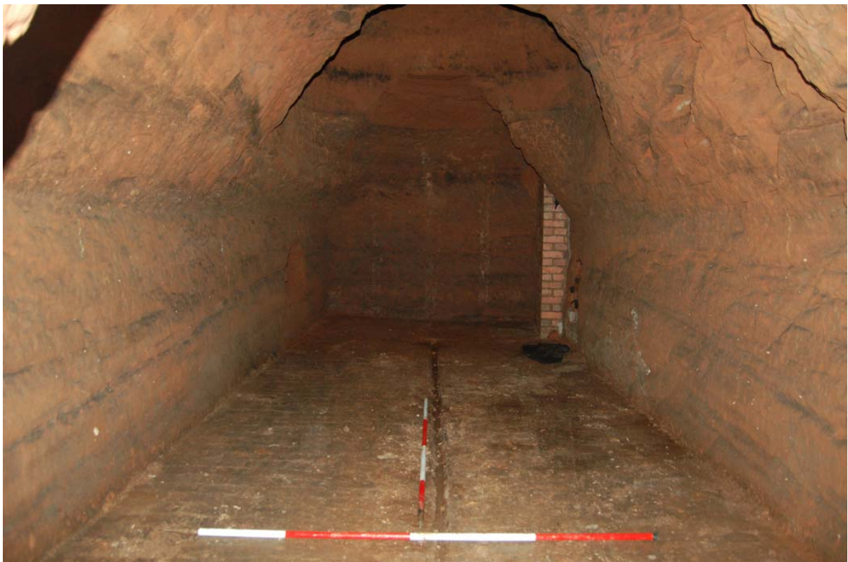
Plate 55: Chamber N2, looking south, note vertical scars in end wall.
