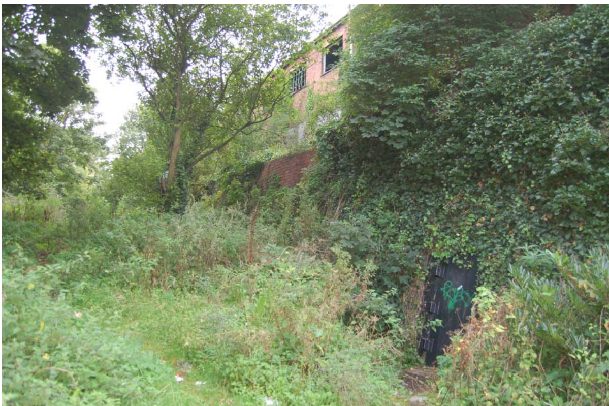
Plate 2: Cavern complex entrance within retaining wall of 'The Cliff'.
