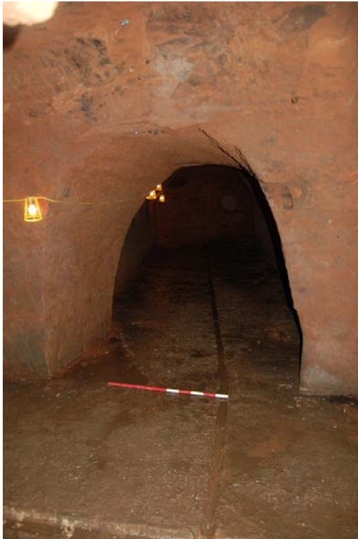
Plate 13: Main Gallery; doorway to S1.
