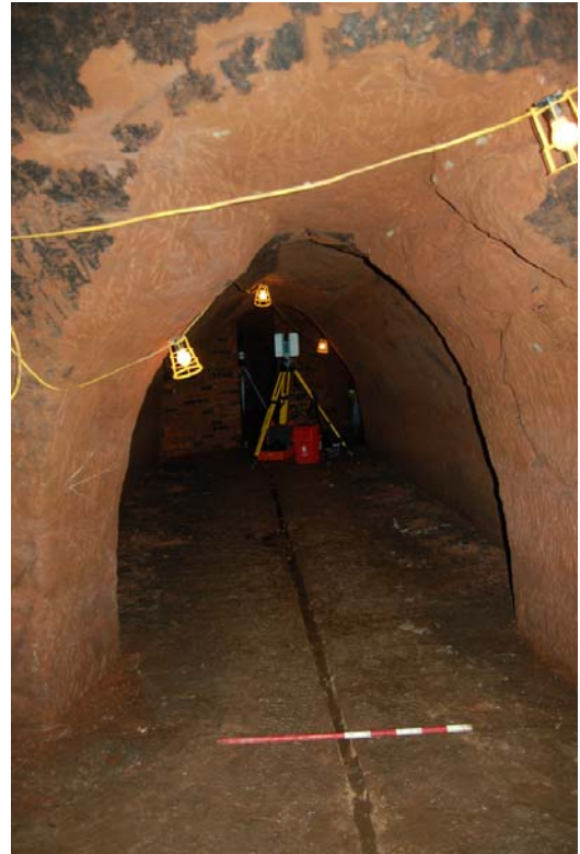
Plate 14: Main Gallery; doorway to S2.
