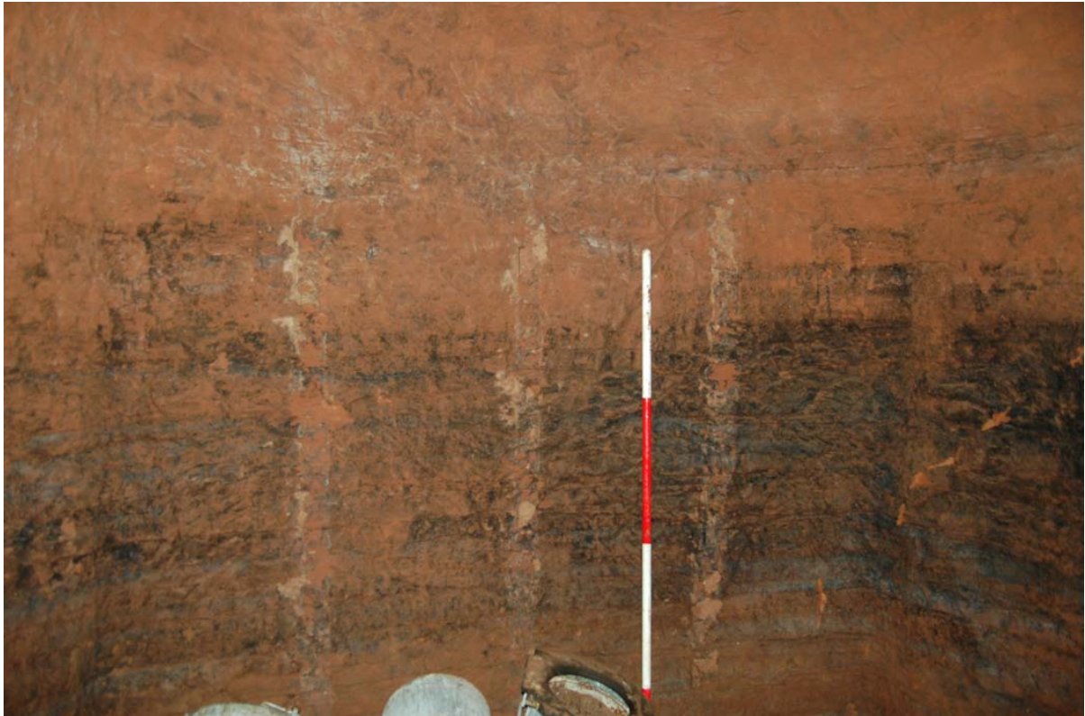
Plate 54: Chamber N1, north end: scars of former toilet partitions.
