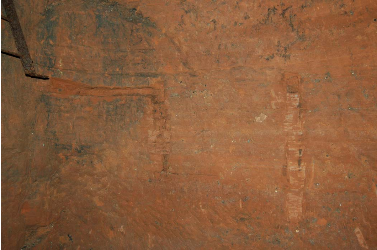
Plate 45: Chamber S5 south end; vertical scars in end wall.
