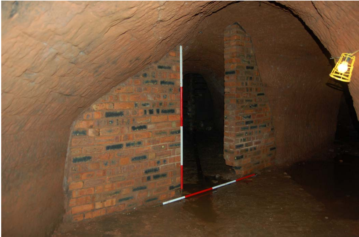
Plate 30: Chamber S2; inserted angled brick wall, note secondary tunnel (r.) to S1 (see Pl.14).
