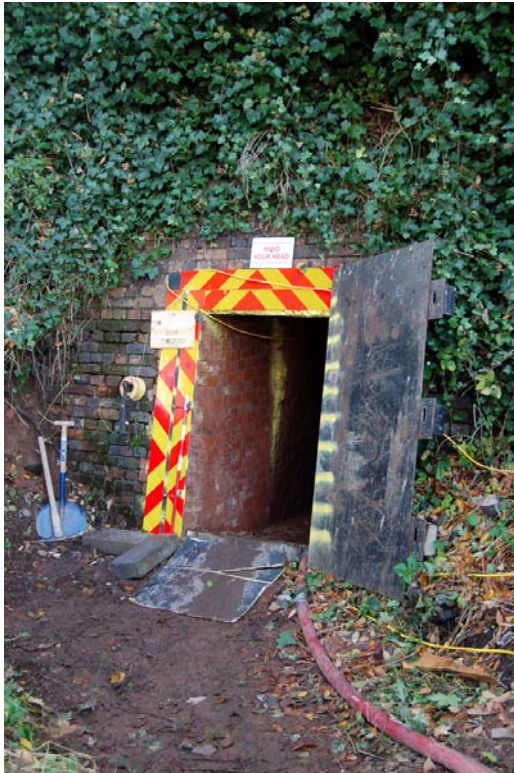
Plate 3: Eastern entrance doorway.
