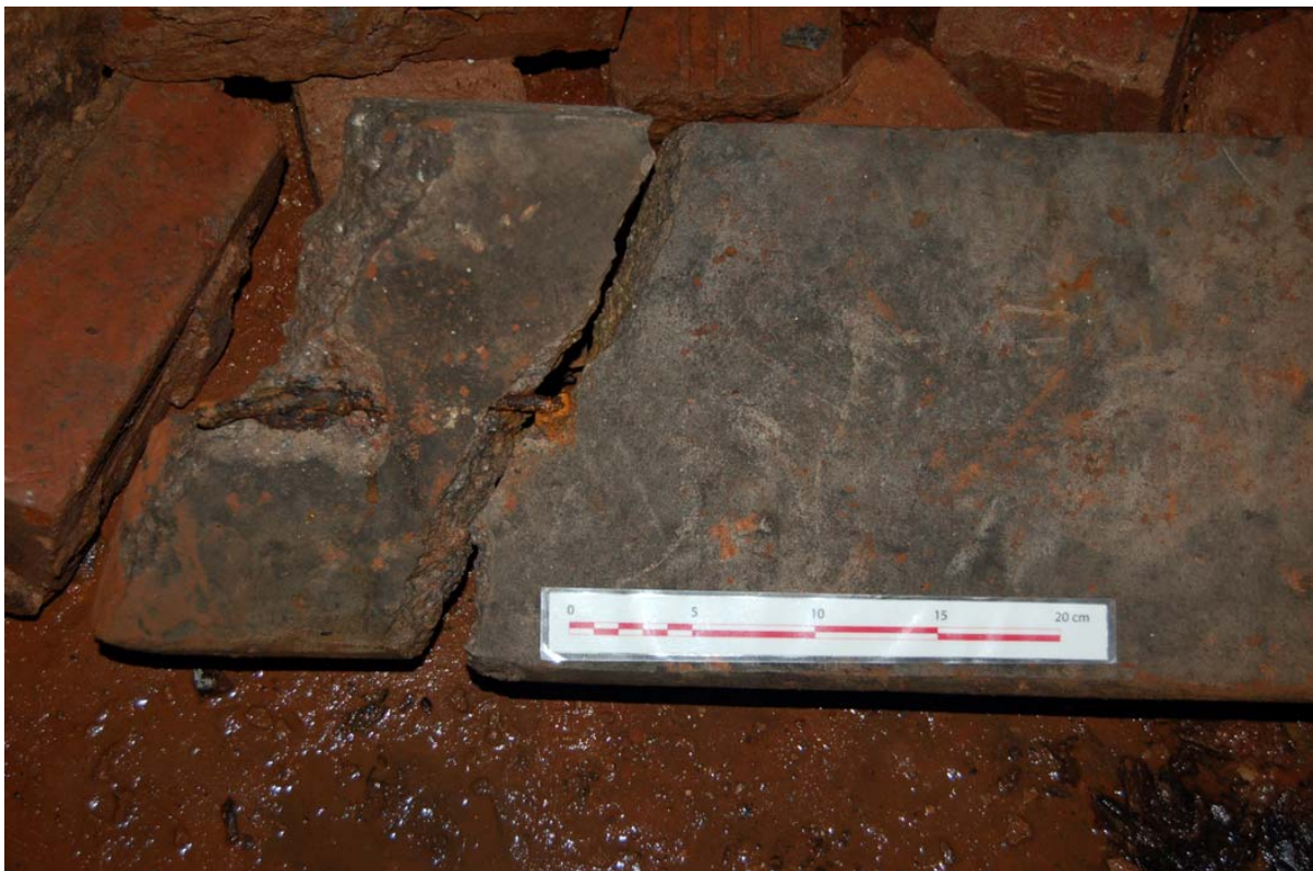
Plate 51: Chamber N1: detail of reinforced concrete bench slab.
