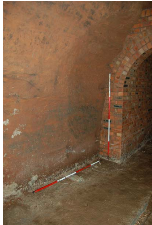
Plate 9: North jamb of wide brick arch.
