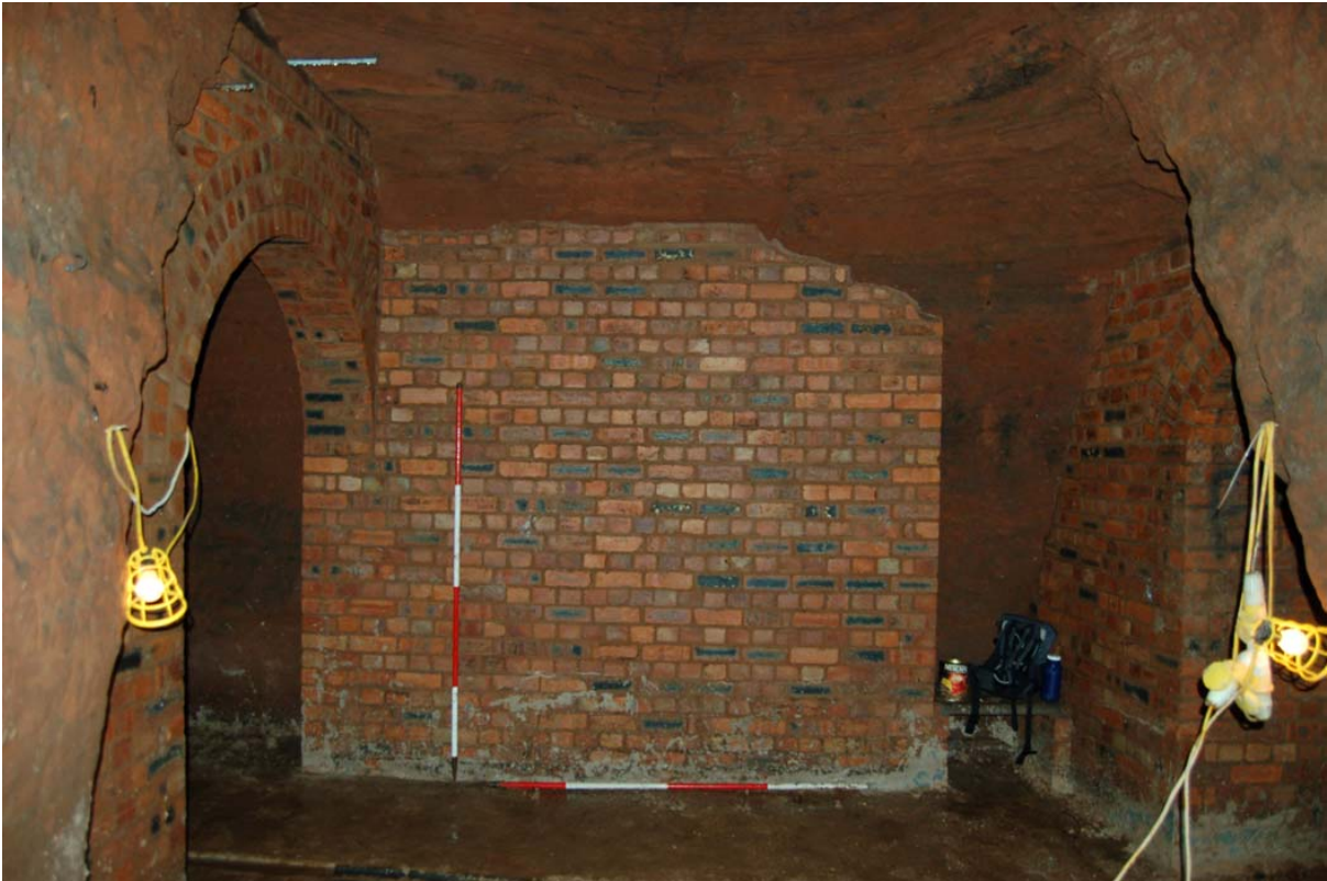
Plate 7: 'Utopia' brickwork against Main Gallery north wall at entrance (→N), note bench to right.
