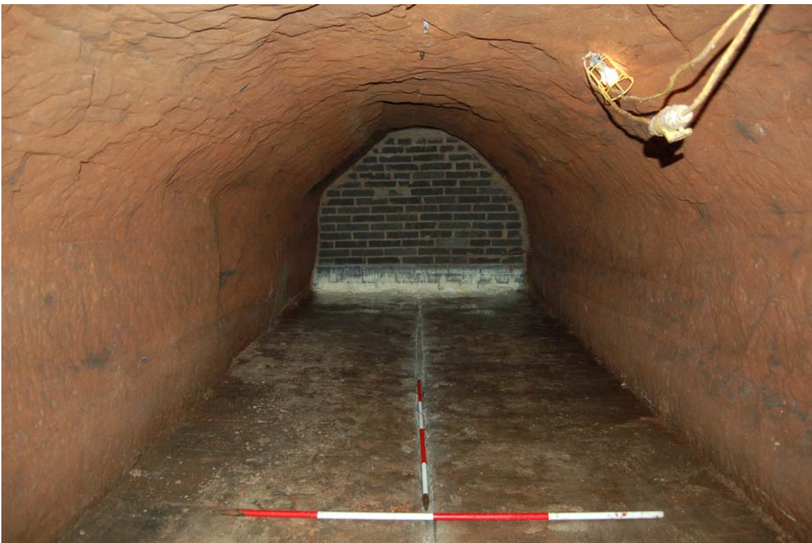
Plate 34: Chamber S3 looking south.
