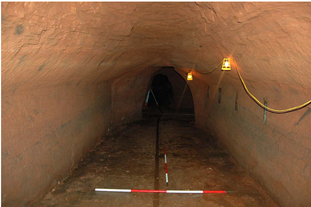
Plate 22: Chamber S1 looking north note brackets on east wall (r.).
