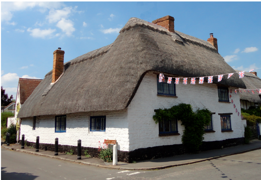
Fig. 1. View from the south
