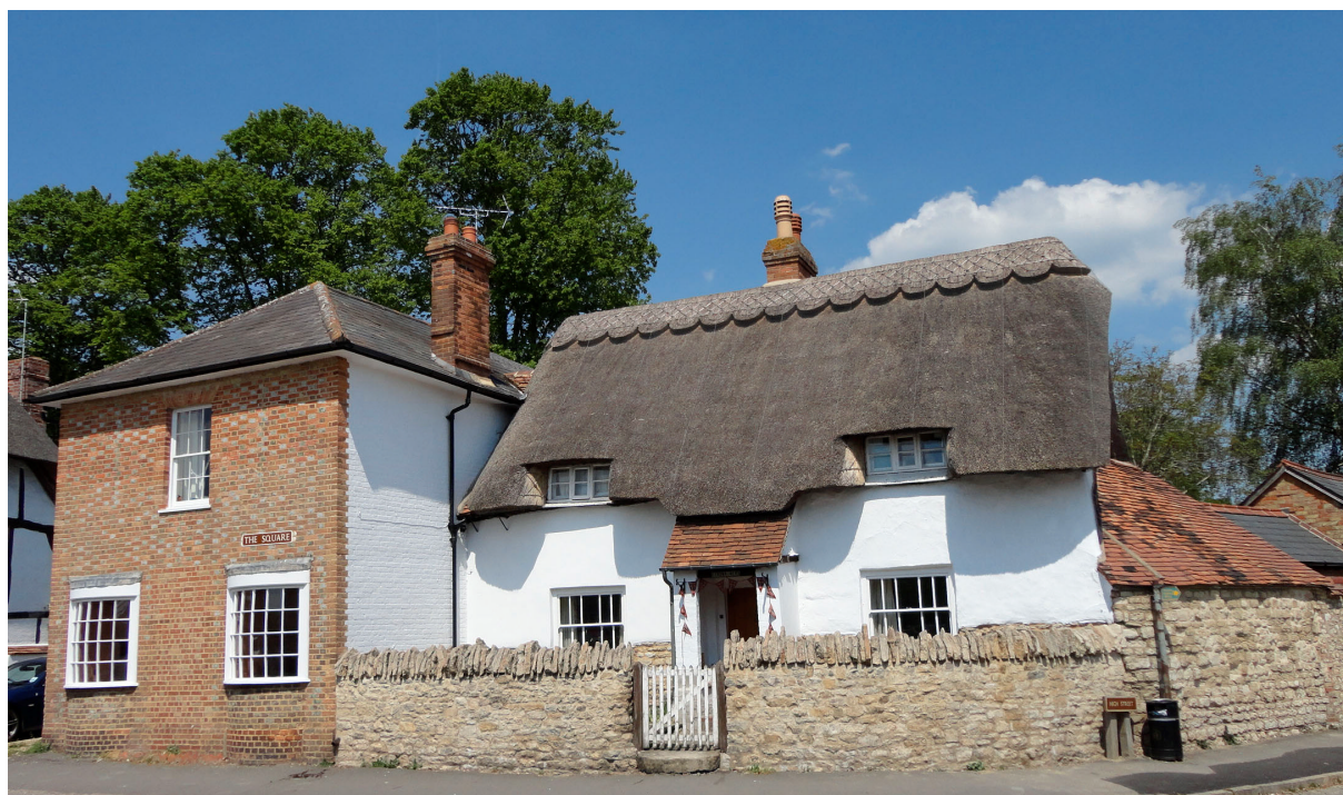
Fig. 1. View of Cordwainers from the south.
