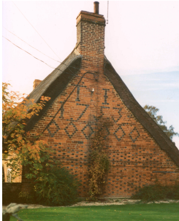
Fig. 2. View of the east gable.
