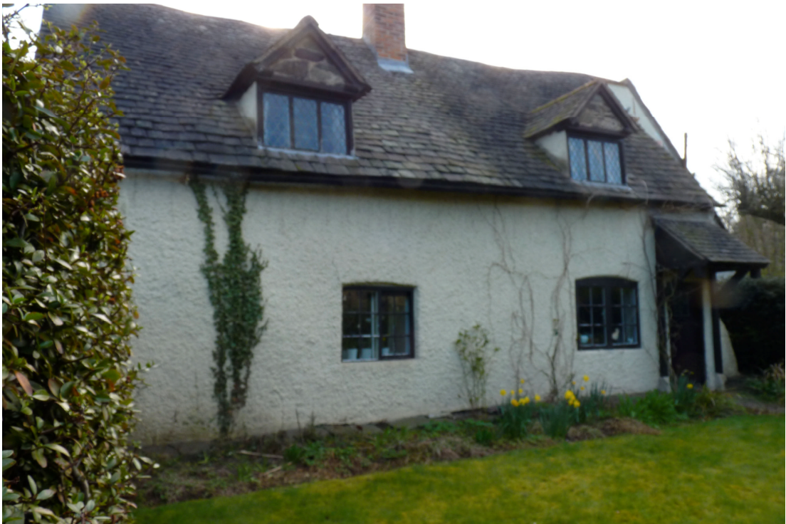
Fig. 1. Old Post Office, Woodhouse, from the north
