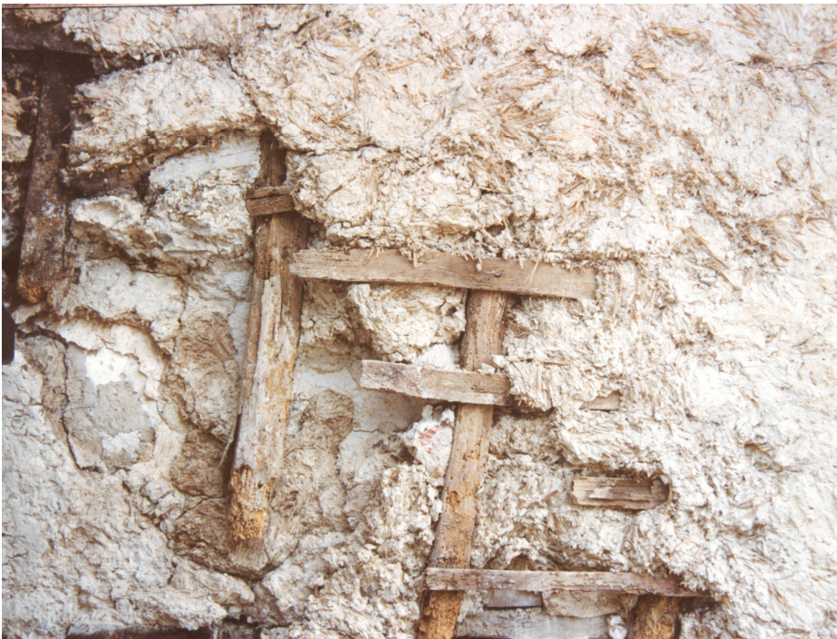
Fig. 8. Original stave and daub infill.
