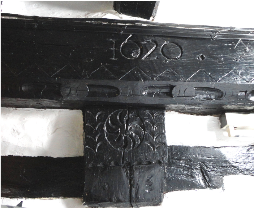
Fig. 10. Beam and bracket in the 1620 block.
