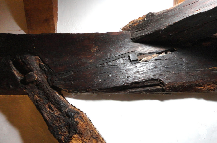
Fig. 7. Wall plate scarf in the chamber block.
