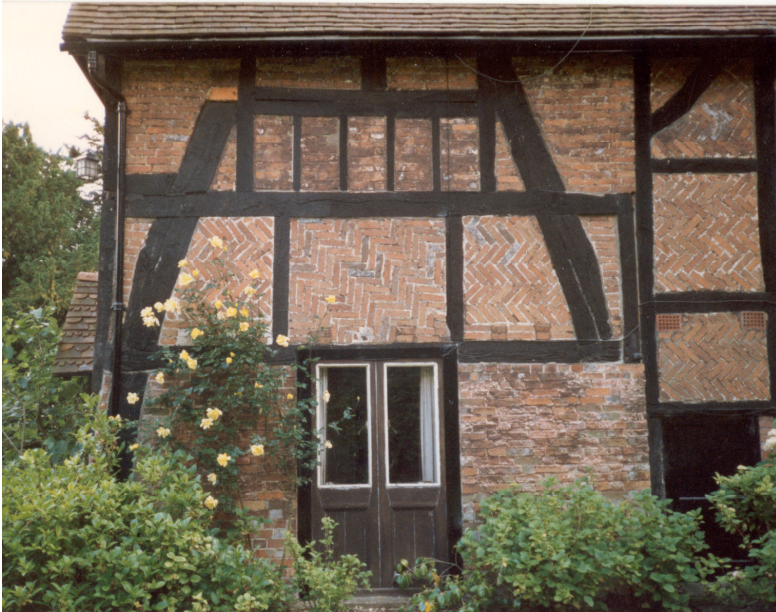
Fig. 2. View from the east, showing cruck T1 incorporated into the later wing.
