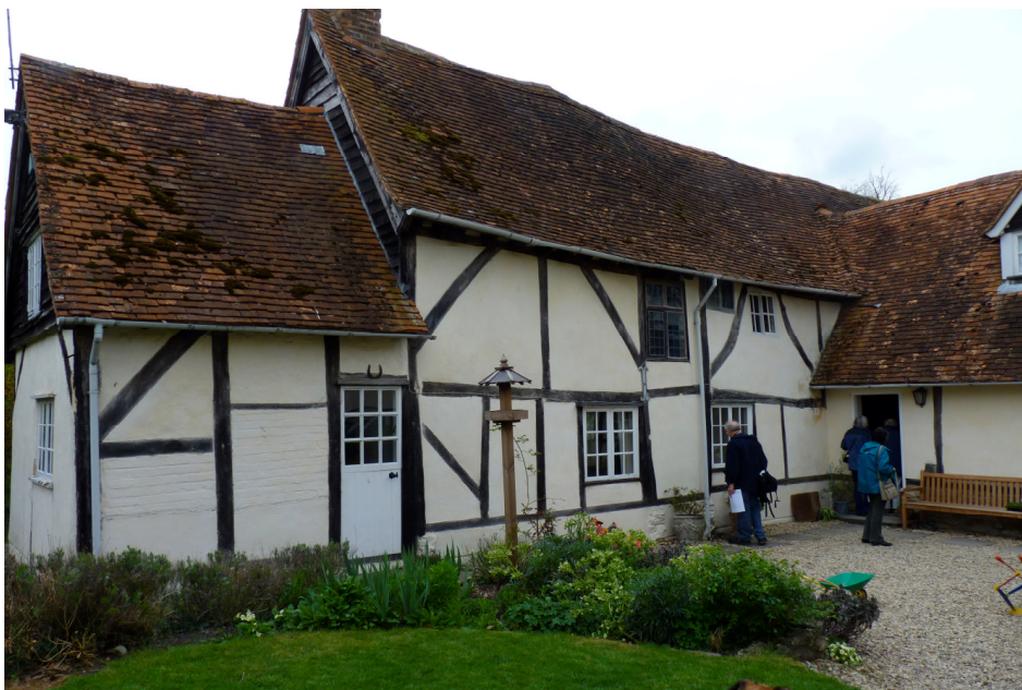
Fig. 2. View from south-east, showing part of the cruck range (right), the end of the original crosswing (centre), the kitchen (centre left) and the low seventeenth-century bay (far left)
