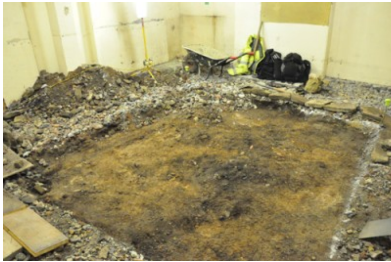
The trench in the cellar.
