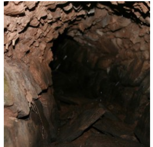
Showing the construction of the drain outlet
