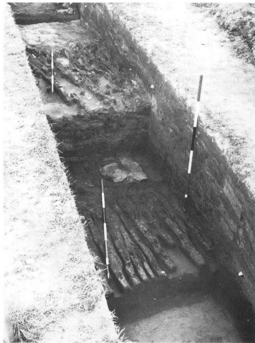
PL. VII B. The Flavian rampart partly cut back, with the Antonine I addition in front resting on remains of timber strapping (p. 17). Scales in feet.
