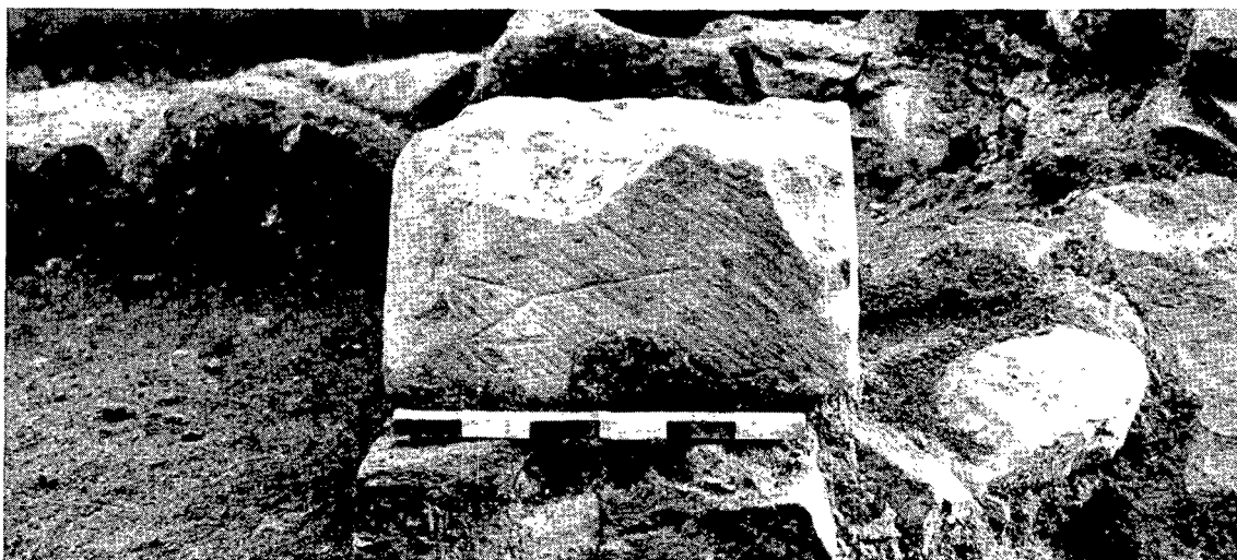
ILL 10 : Aberdeen, 12 Martin's Lane. Trench 4. Mason's mark on a stone used in construction of Building 1
