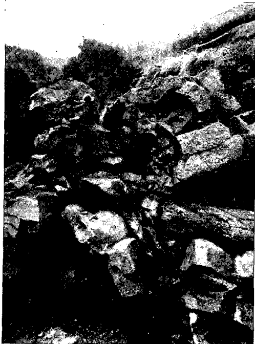
Fig. 6. Elevation of Wall, showing Vitrification.
