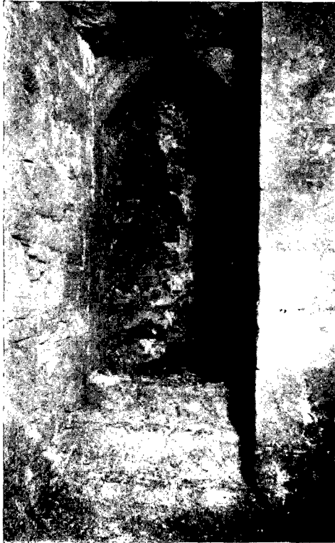
Fig. 14. Doorway on north side of Entrance Hall.
