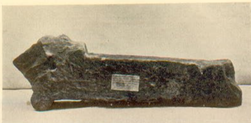
Fig. 33. Moulded Stone Rybate, apparently from oriel window.
