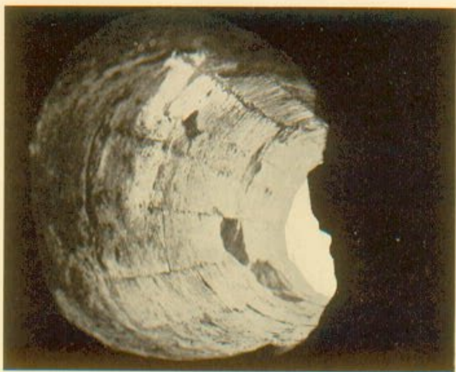
Fig. 17. Tapered Loop-hole of Battery.
