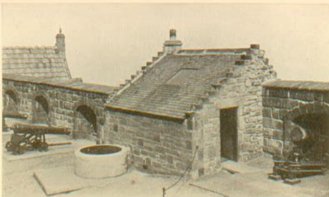
Fig. 34. View showing new Well-head to ancient Well.
