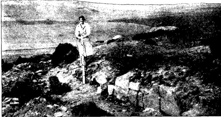
Fig. 8. West Fort: Revetment of Middle Bank in Section IIIA.
