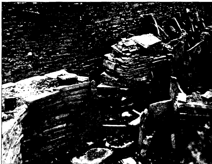
Fig. 20. Midhowe Broch: East end of south wall of chamber H, showing late doorway slapped in wall and entrance to compartment H3 in front.
