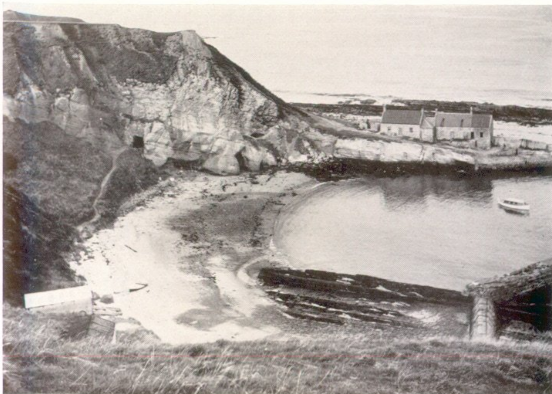
1. General view showing mouth of tunnel
