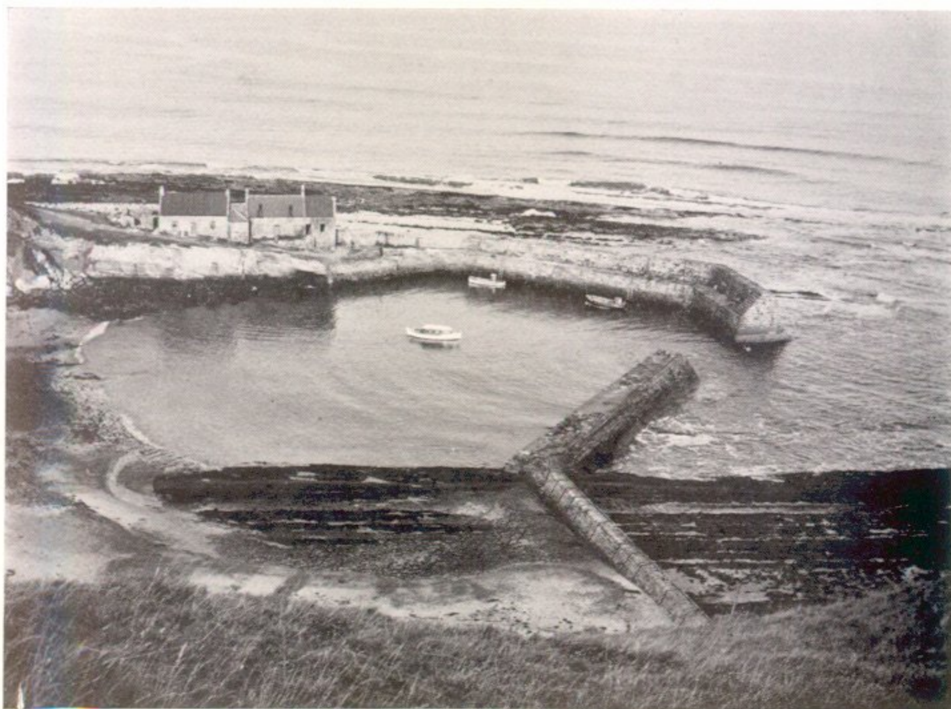
2. General view showing North and South Piers
