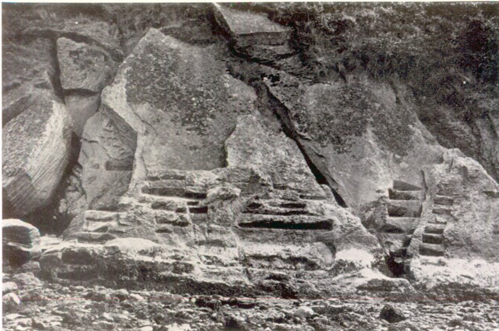
1. Tusking and steps at site of earlier breakwaters
