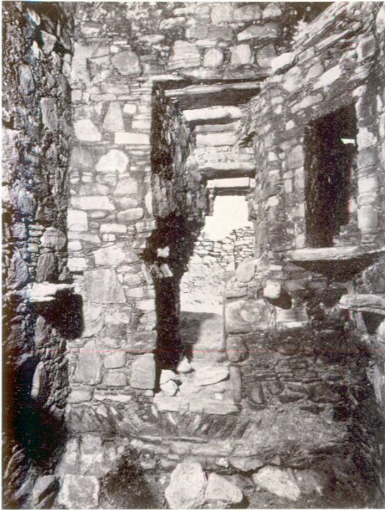
a Interior of tower-house from W showing entrance-doorways
