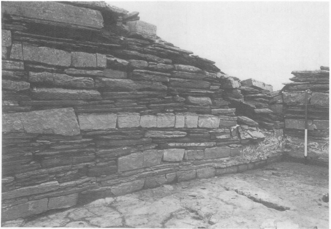
ILLUS 16 North wall of Chapel, from south-west (D Jeffrey)
