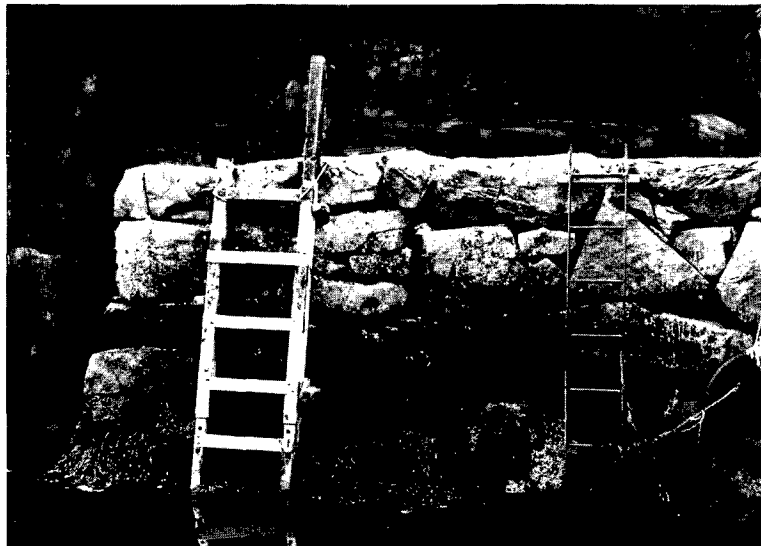
ILLUS 42 Crinan: the head of the quay. Even the rough boulders have been set to flare slightly at the base and are battered on both the seaward faces of this structure. Compare the masonry of the Beilding (Tarbert Loch Fyne)
