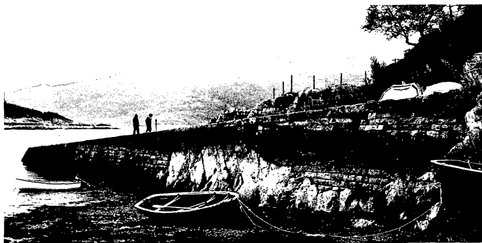
ILLUS 39 Salen, Loch Sunart: the courses of Telford's ferry pier are neatly fitted on to the natural rock foundation, which has not been levelled or stepped. Contrast Portmahomack south pier
