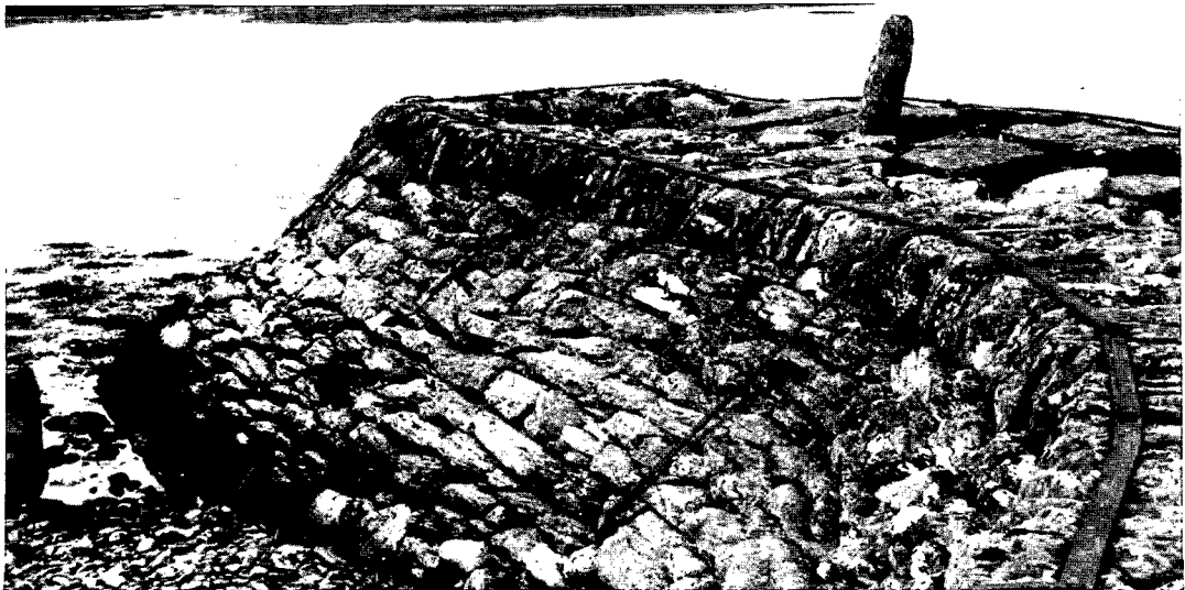
ILLUS 56 Keills: run-bar and straps bolted to pier surfaces, without channels; those on the nearby slipway were set in channels on the seaward sides only
