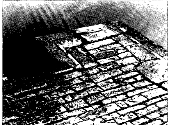
ILLUS 55 Inveraray: run-bar in channel, securing the end of the slipway and the top of the steps
