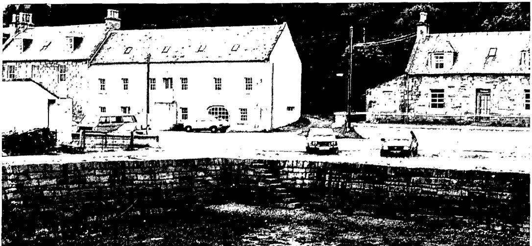
ILLUS 5 Fortrose: courses of red sandstone blocks without mortar. The neatness is characteristic of structures actually supervised by Telford
