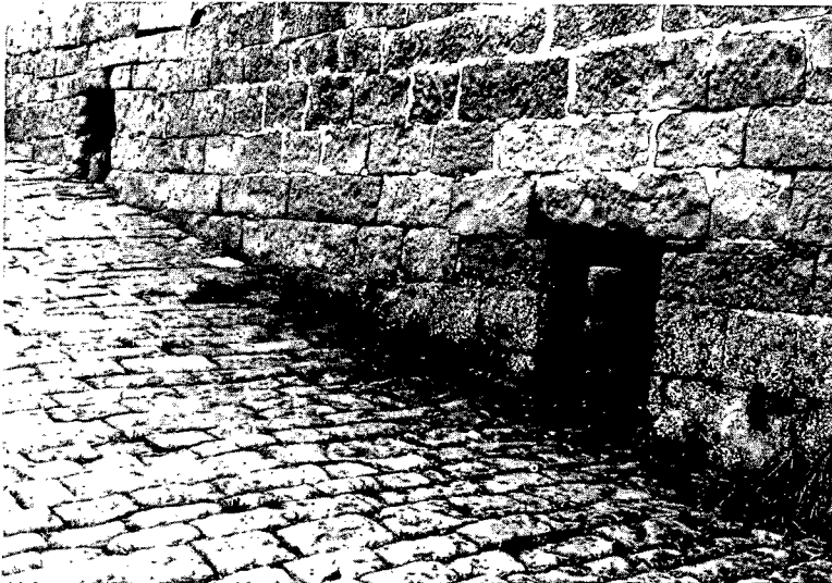
ILLUS 52 Inveraray: pawls in niches beside the slipway used by the ferry to St Catherines, which took carriages
