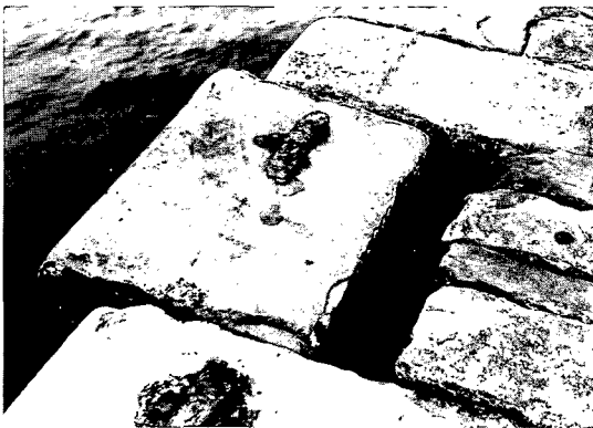
ILLUS 54 Rockfield: kerb block loosened after rusting away of run-bar
