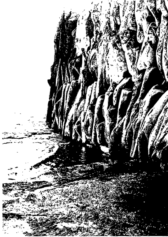
ILLUS 31 Castlehill: sea wear on the tiered vertical flagstones, some five feet high, set by Bremner to form the slightly battered outer face of the north-west pier. The whitish patch (centre top) is repair work in cement to characteristic mid-section damage
