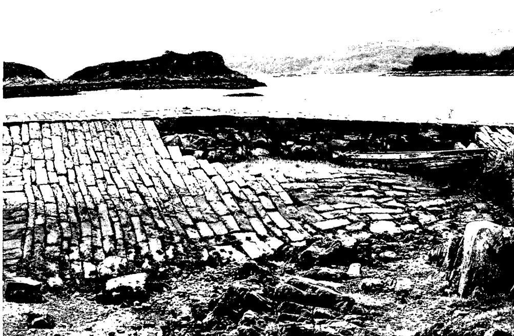
ILLUS 38 Kentra: broken breastwork on the shore side of Telford's ferry pier. The dressed stone has probably been put to other use
