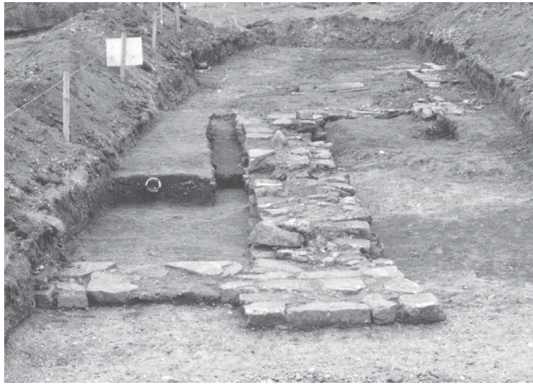
ILLUS 6 Wall [222] during excavation (from NE)
