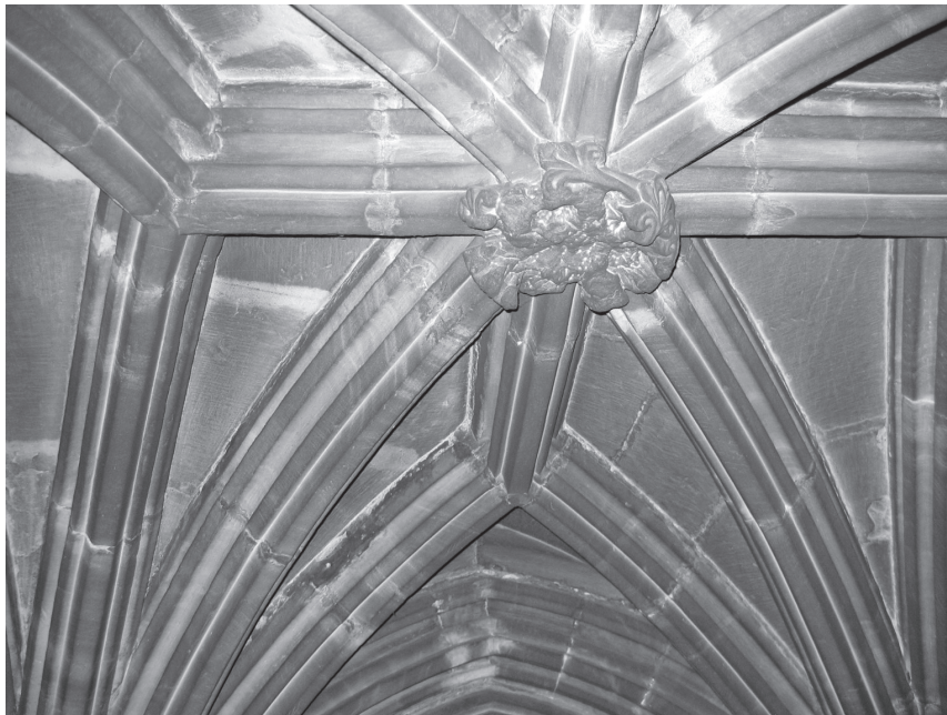
ILLUS 15 Glasgow Cathedral crypt, vault over north staircase landing
