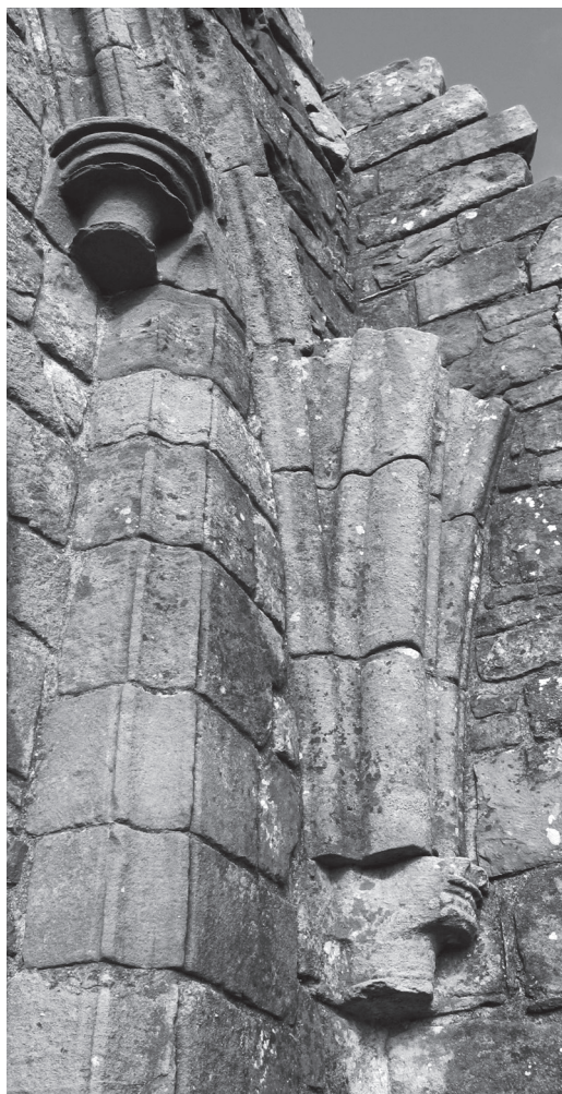
ILLUS 16 Dundrennan Abbey chapterhouse, north-west corner
