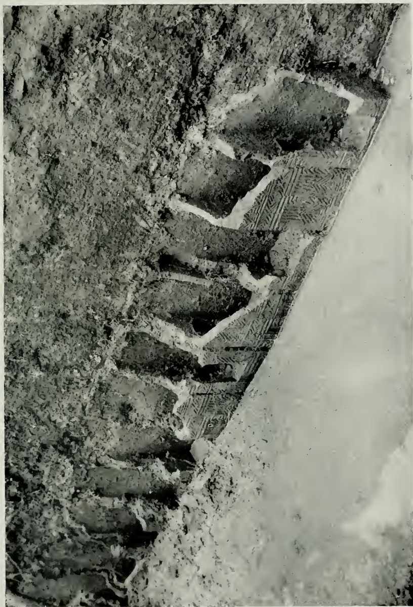
BOX-FLUE TILES OF KEYED VARIETY IN HYPOCAUST OF ROOM 6.
