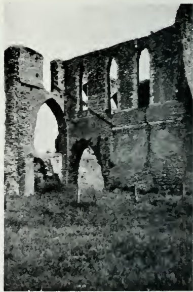
W. wall of S. transept and S. side of retro-choir, showing marks of S. aisle roof.
