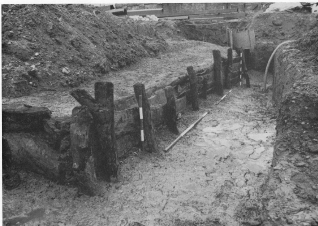
Fig 3. Kingston Horsefair 1987: detail of waterfront of c1300 made up of re-used boat timbers, adjoining the downstream side of the medieval bridge. (Photograph by courtesy of the Museum of London)
