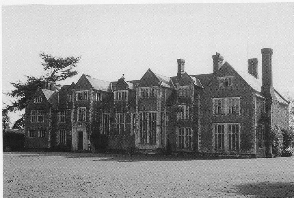
Fig 4 The north (entrance) elevation of Loseley House in 2001 from the north-west. By kind permission of Loseley Park.
