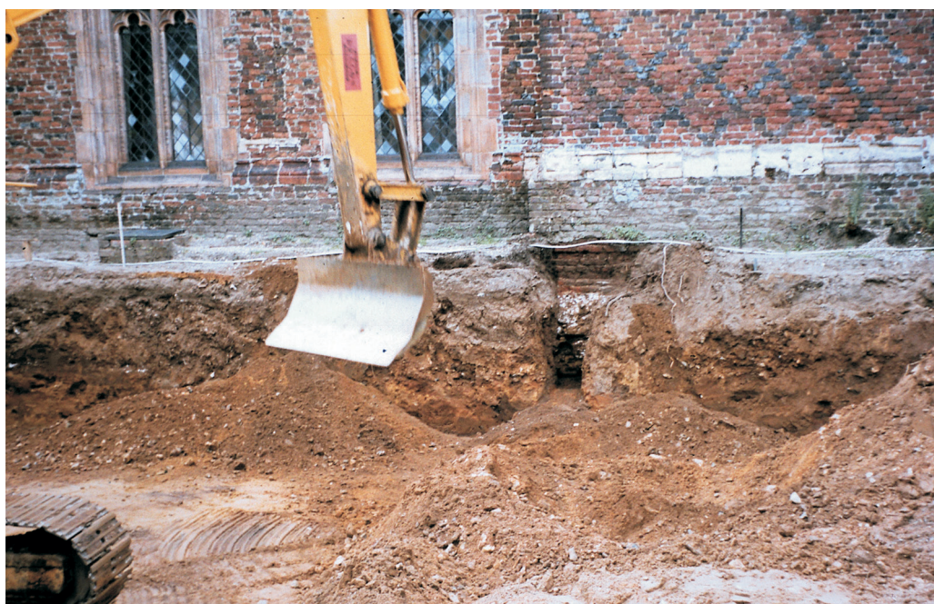
Fig 15 Sutton Place. View of the machine-cut east wall foundation section.
