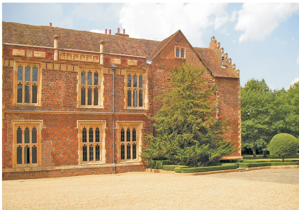
Fig 1 Sutton Place. The northern end of the west wing in 2006 showing the location of its original junction with the north wing (vertical scars either side of the tree below the gable) and in the foreground one of the planting beds marking the outline of the gatehouse wing (in the wrong place). (Photograph: Martin Higgins, © Surrey County Council Heritage Conservation Team)
