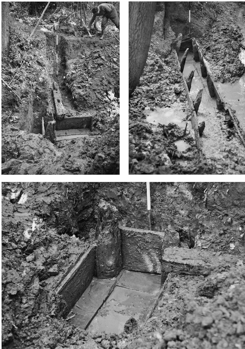
Fig 3 Coneyhurst Gill, Ewhurst. The site during excavation: top left, looking east along the sleeper beam at the base of the dam (NMR AV364); top right, looking north along the covered launder (NMR AV366); bottom, looking east across the end board at the base of the dam (NMR AV374) (photographs by Ken Gravett reproduced by kind permission of the National Monuments Record).
