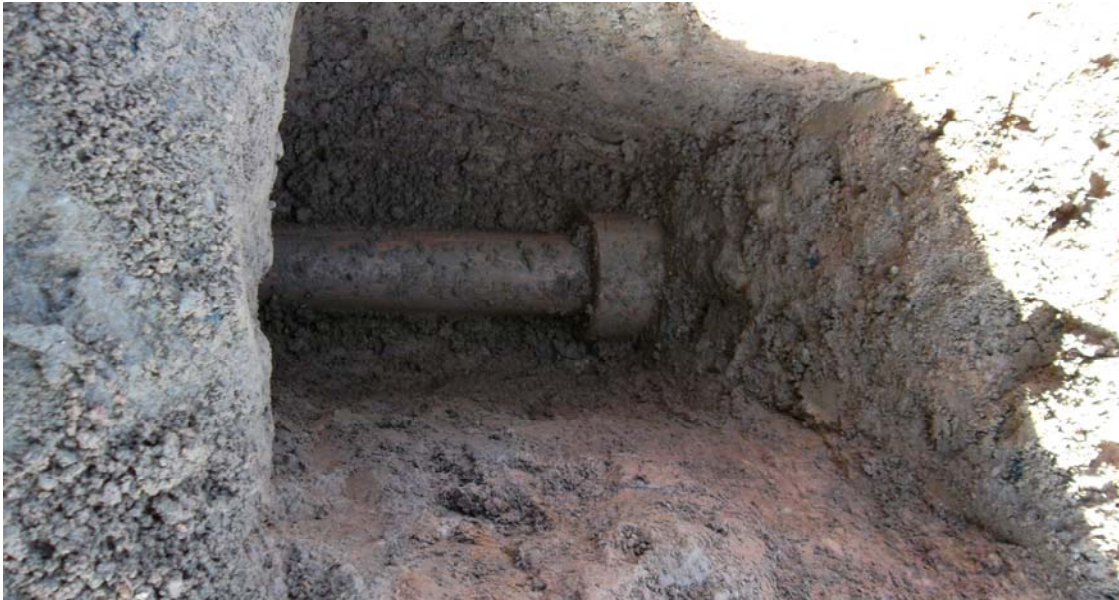
Plate 2: View of ceramic drain, Trench 21
