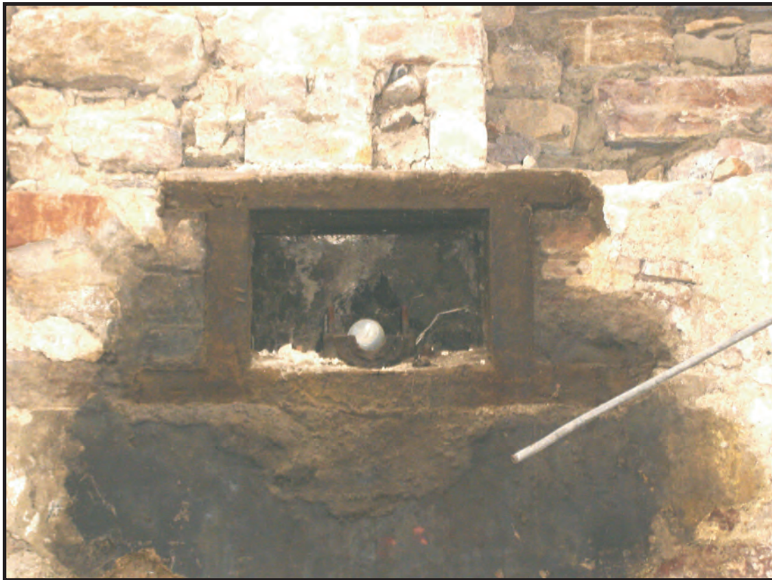
Plate 36: Room A3, detail of the bearing box F45 along the north-west wall
