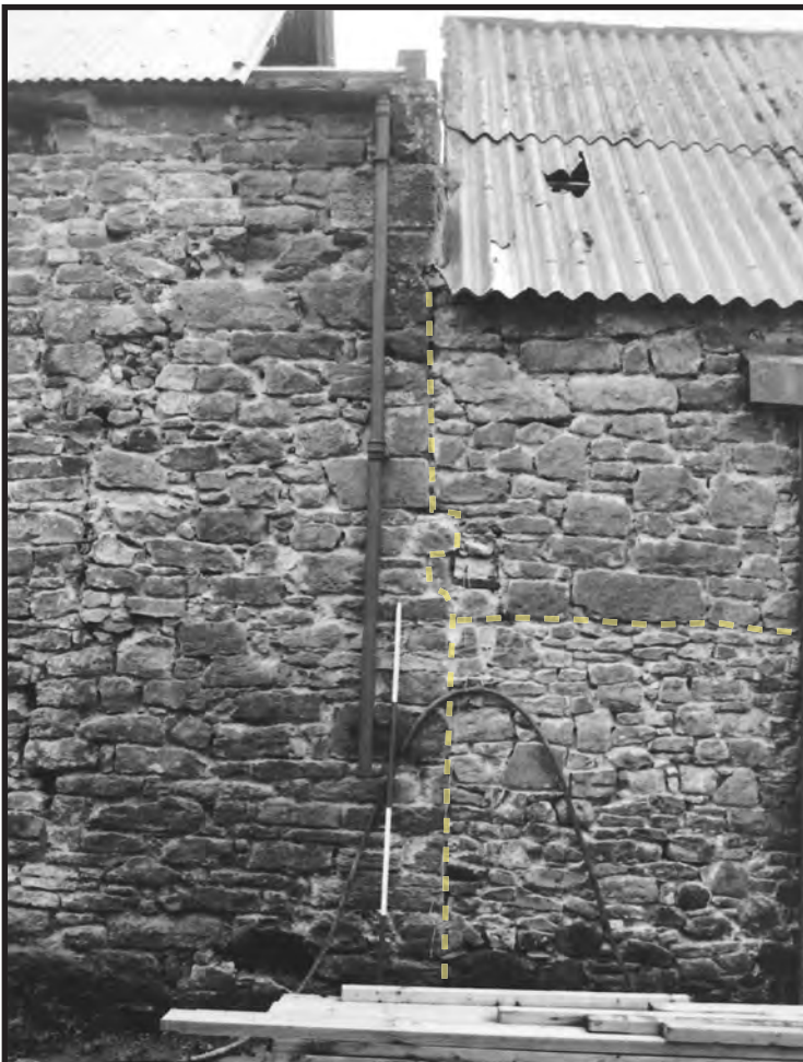
Plate 12: Detail of the phase break between Phases 2b & 2c and Phases 2d & 2e - the yellow dashed line shows the levelling courses associated with the later building to the right showing Phase 2d (below) and Phase 2e (above)
