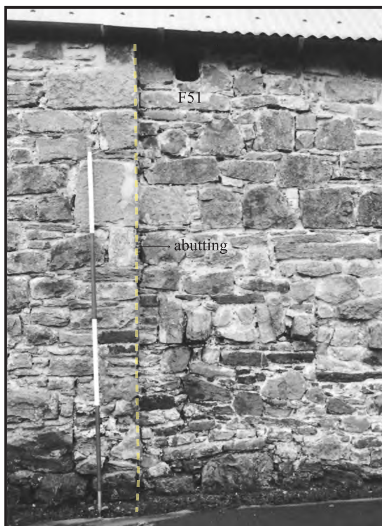
Plate 43: Building B, detail of the possible earlier wall (to the left) on the south-west facing elevation
