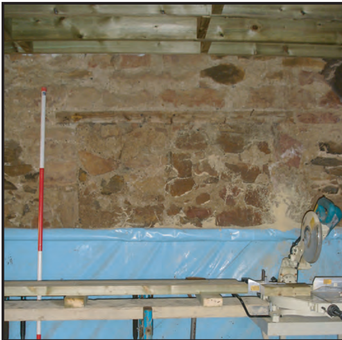
Plate 41: Room A4, detail of blocked window (F47) along the south-east wall
