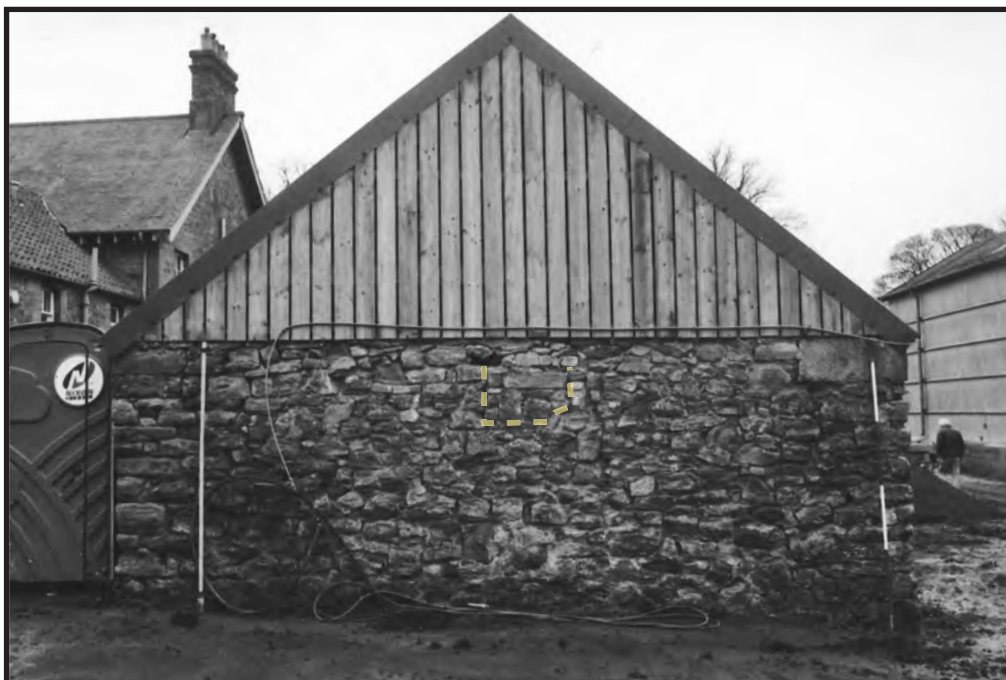
Plate 23: The north-east gable elevation of Building A, with stone-blocked opening (F42) highlighted
