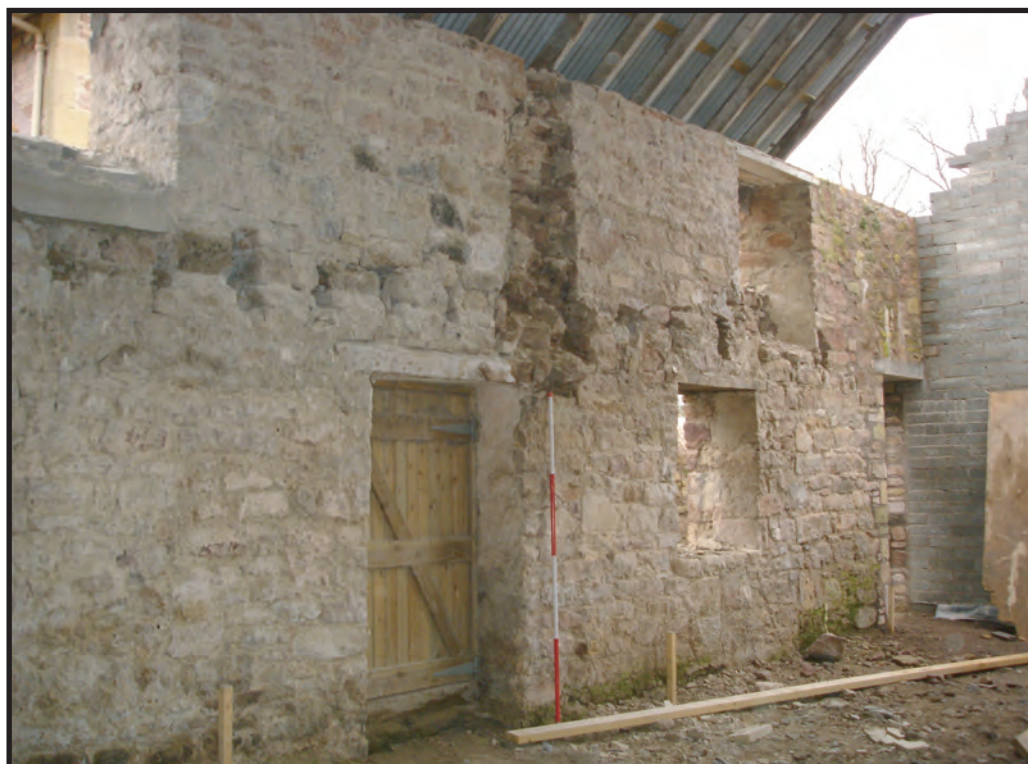
Plate 30: Room A2 from the east - note the now removed stone partition wall (F48a) to the first floor
