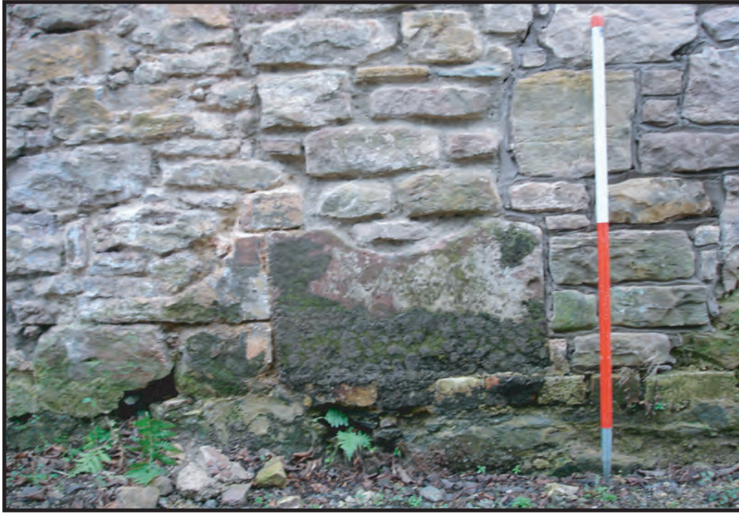
Plate 9: Detail of the machine support (F14) to the base of the north-west facing elevation of the central wing of Building A to the south
