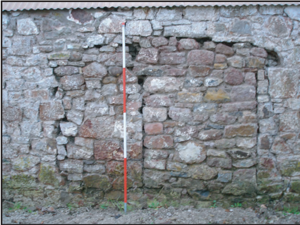
Plate 50: Building B, detail of the central stone-blocked door F58 on the north-east facing elevation
