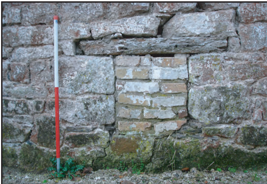
Plate 51: Building B, detail of one of the small bricked-up openings F59 along the north-east facing elevation
