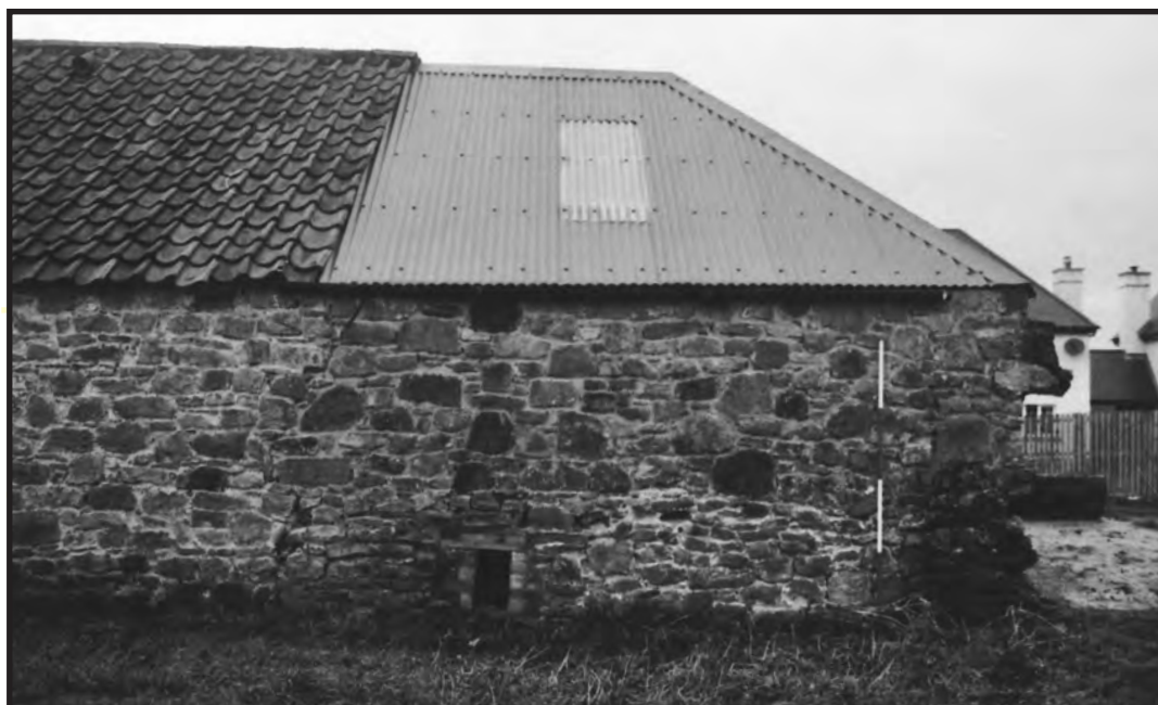
Plate 55: Building B, detail of the north-east side of the south-east facing elevation showing the later inserted opening F61
