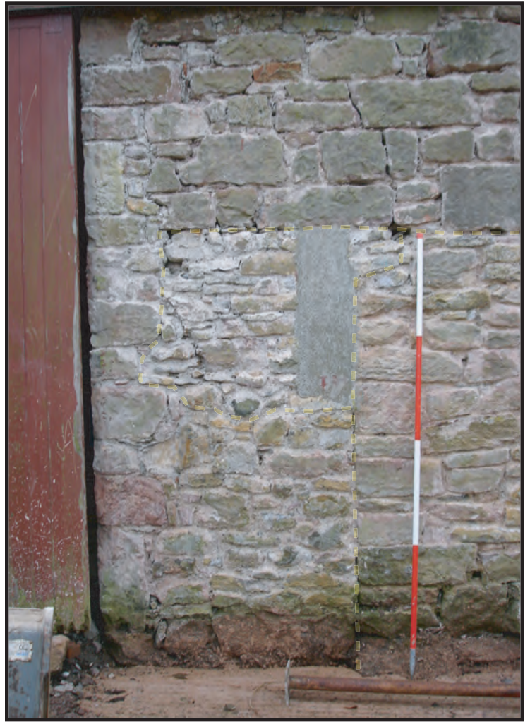
Plate 11: Detail of the stone-blocked doorway (F18) and window (F17) along the north-west facing elevation of the southernmost wing of Building A
