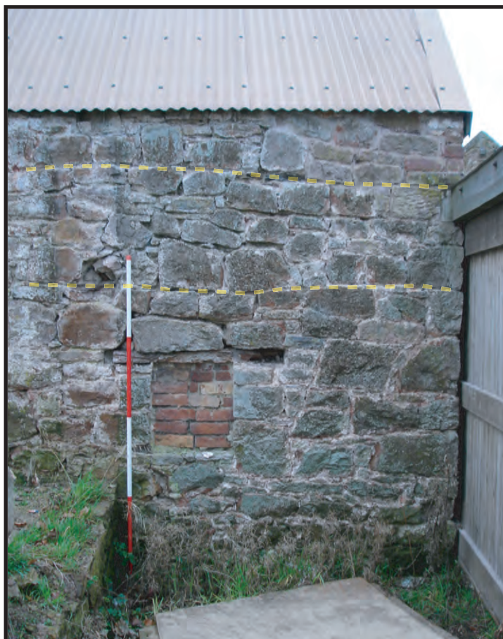
Plate 53: Building B, detail of the bricked-up window F59 and levelling courses along the north-west side of the north-east facing elevation identified by yellow dashed lines
