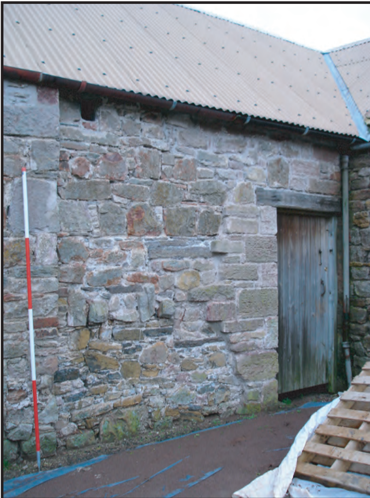
Plate 45: Building B, the south-east facing wall to the south-east showing the reconstructed stonework to doorway F52
