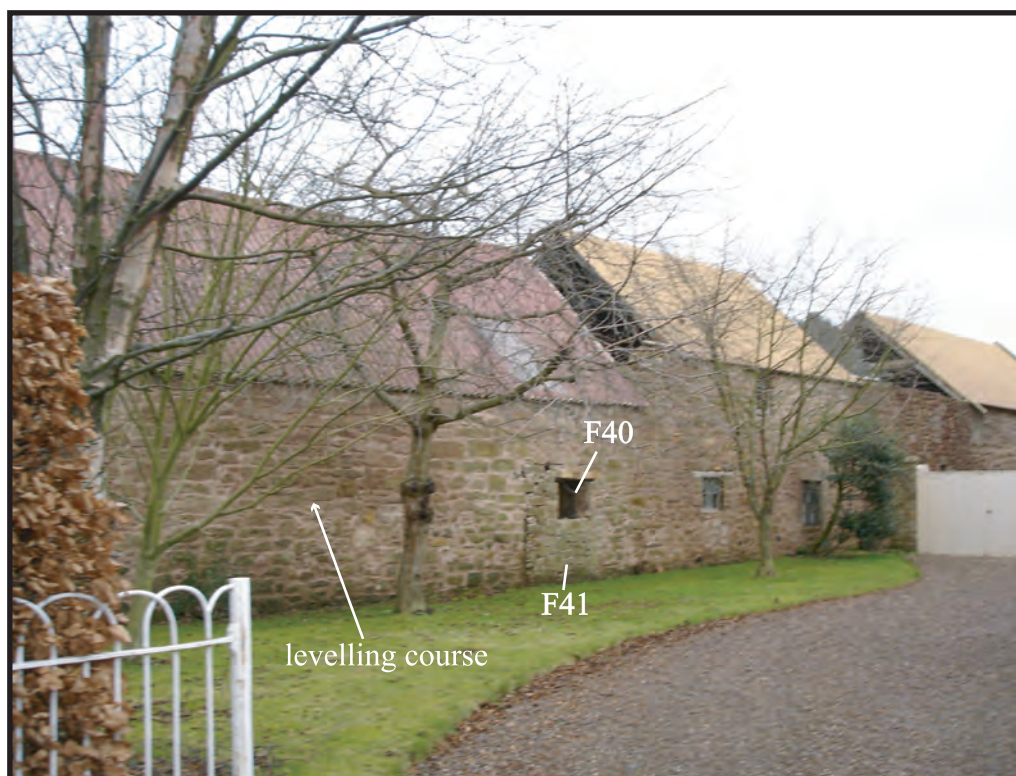
Plate 22: General view of the south-east facing elevation of Building A from the south showing (centre) window F40, a later insertion within the stone blocking of doorway F41
