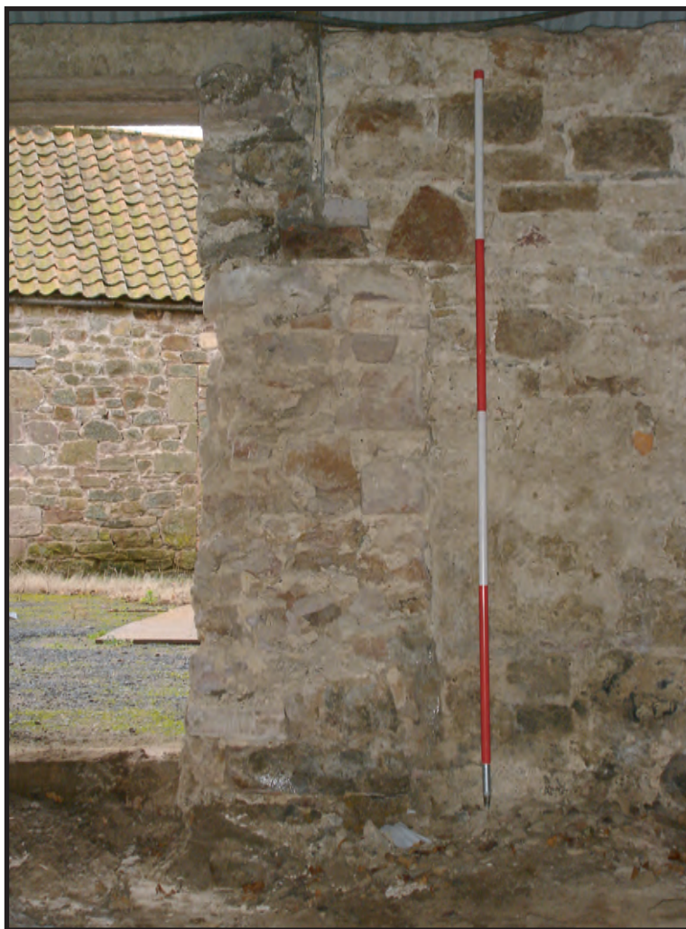
Plate 25: Room A1, detail of the former (possible?) partition wall (F24) on the south-east wall
