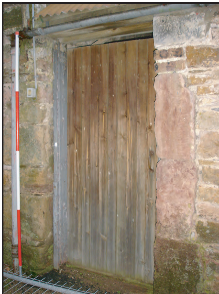
Plate 18: Detail of doorway F26 on the south-east facing elevation of Building A - note the original end of Bay 1 to the left set slightly forward of Bay 2
