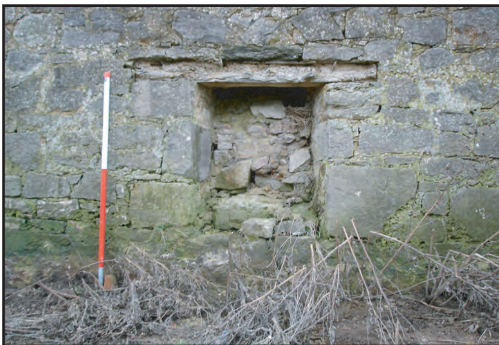
Plate 65: Detail of former window (originally internal window) on the Building D south-east facing boundary wall
