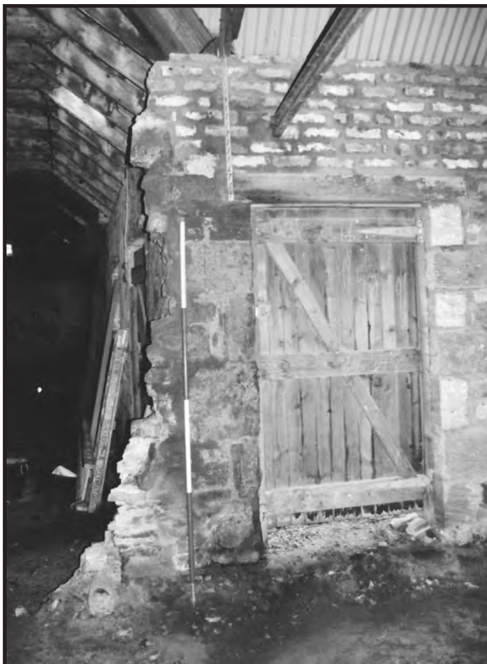
Plate 59: Building B, Area B1, detail of the south-west wall showing the broken away stone partition wall (F62) (to the left)
