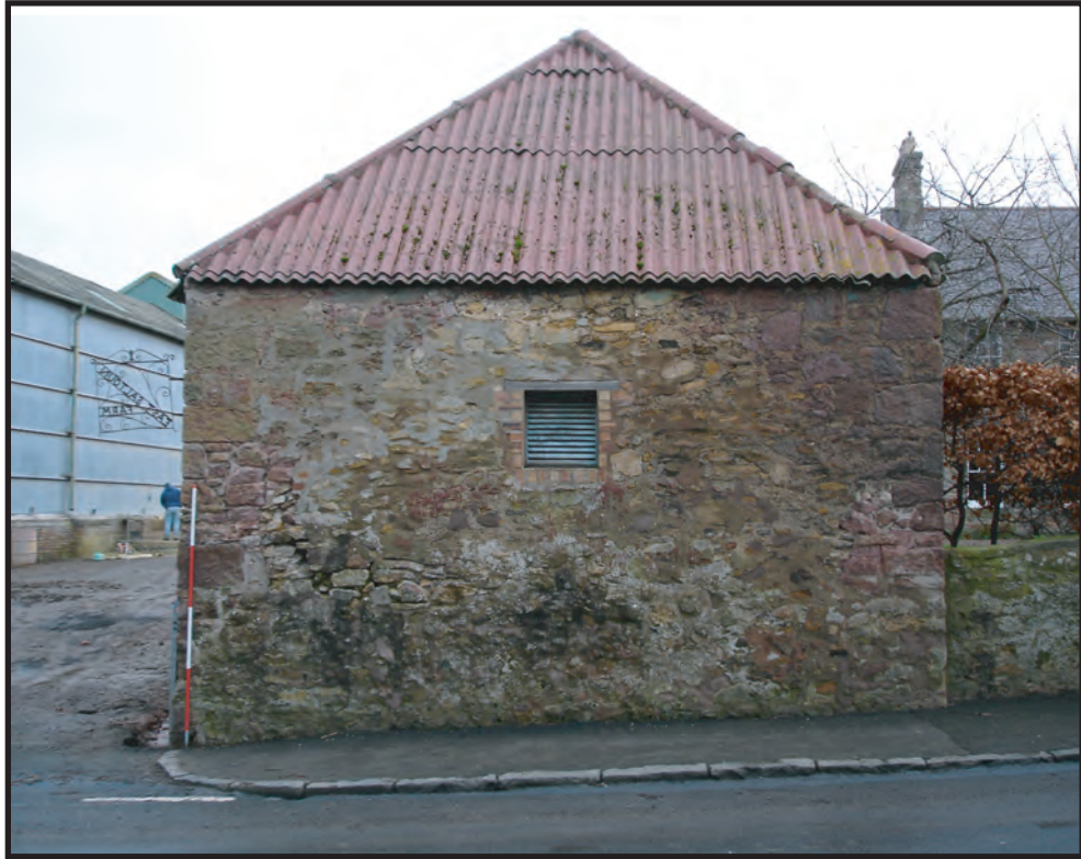
Plate 13: The south-west gable elevation of Building A showing later inserted window F21
