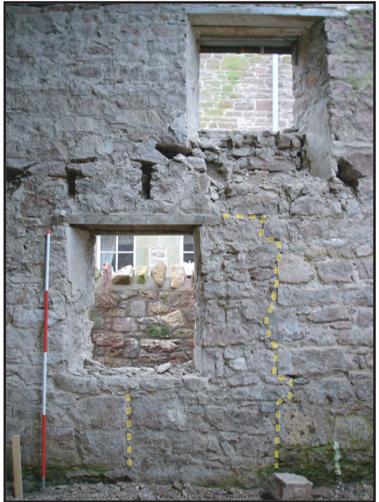
Plate 31: Room A2, detail of the windows F29 in the south-east wall showing the ground floor stone blocked doorway (F31)- yellow dashed lines identify the extent of the blocked feature
