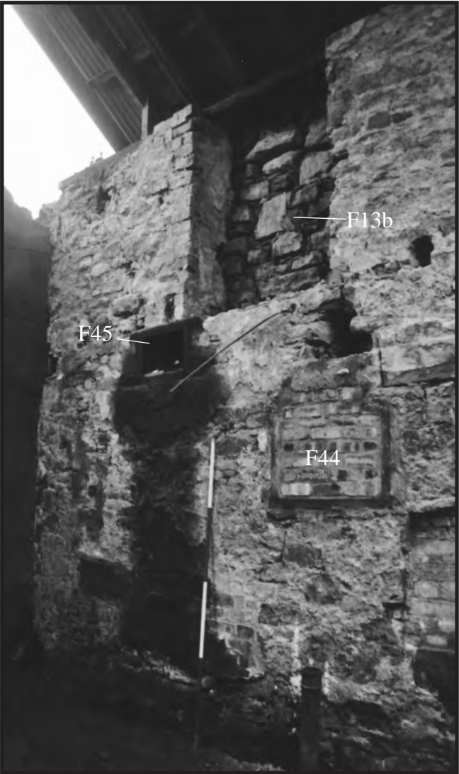
Plate 35: Room A3, detail of the southern end of the north-west wall showing the blocked openings (F44 & F13) and bearing box (F45) associated with the threshing machinery and adjacent engine house (Now demolished)
