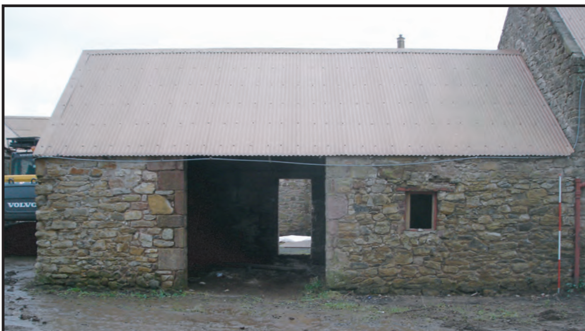
Plate 1: The north-west facing elevation of Building A to the north showing the original Phase 2a building with original cart shed door (F01) and later inserted window (F02)
