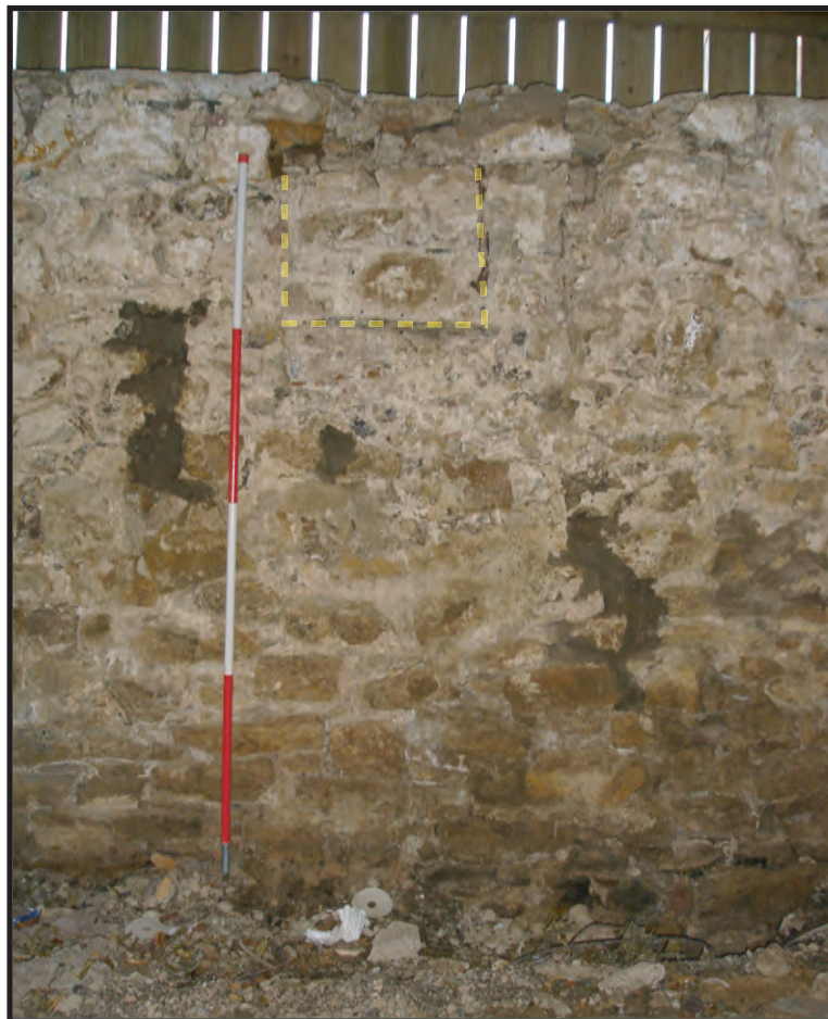
Plate 28: Room A1, detail of the stone-blocked opening (F42) on north-east gable wall (the yellow dashed line outlines the feature)
