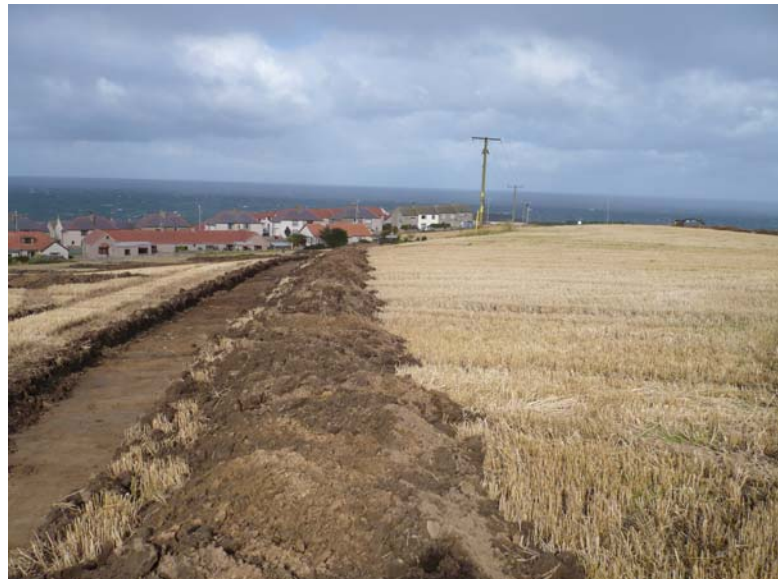
Figure 3: General view of trench, post-excavation
