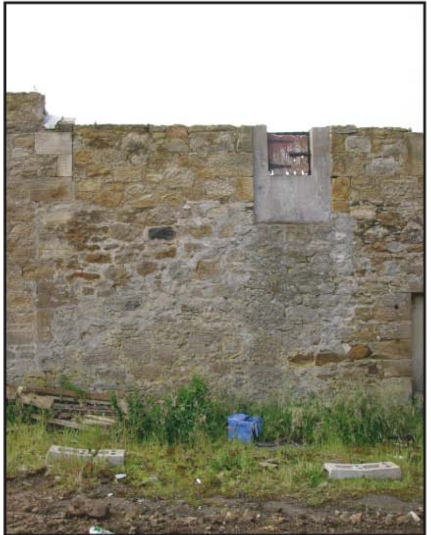
Plate 7: Detail of the scar of the former external stair on the north wall of Building B
