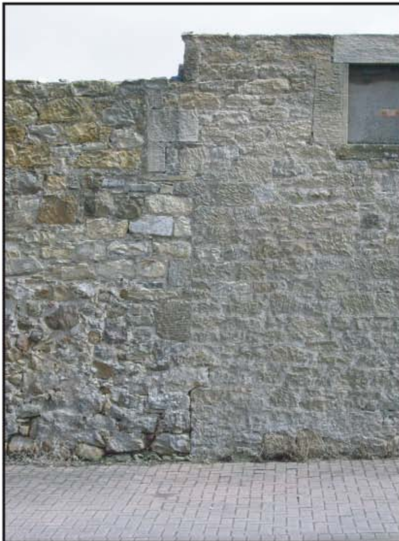
Plate 3: Detail of the phase line between Buildings A & B on the south wall
