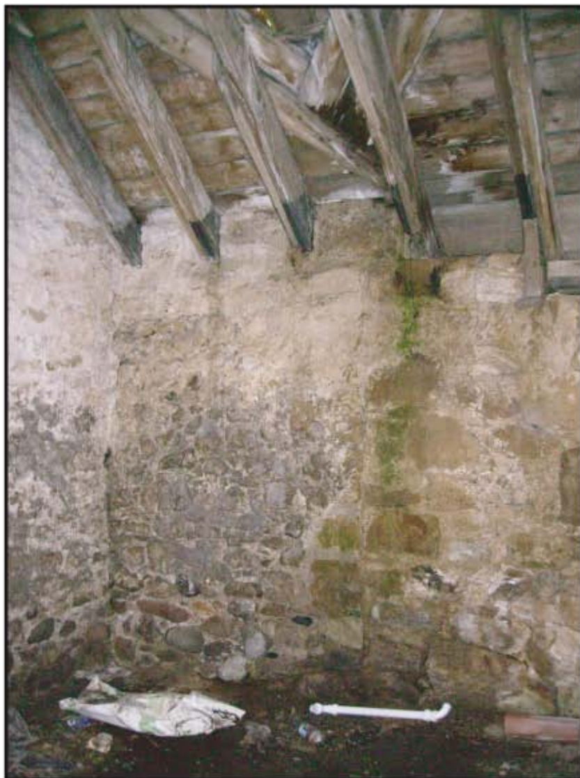
Plate 17: Detail of the stone blocked door in the north wall of the central room of Building E
