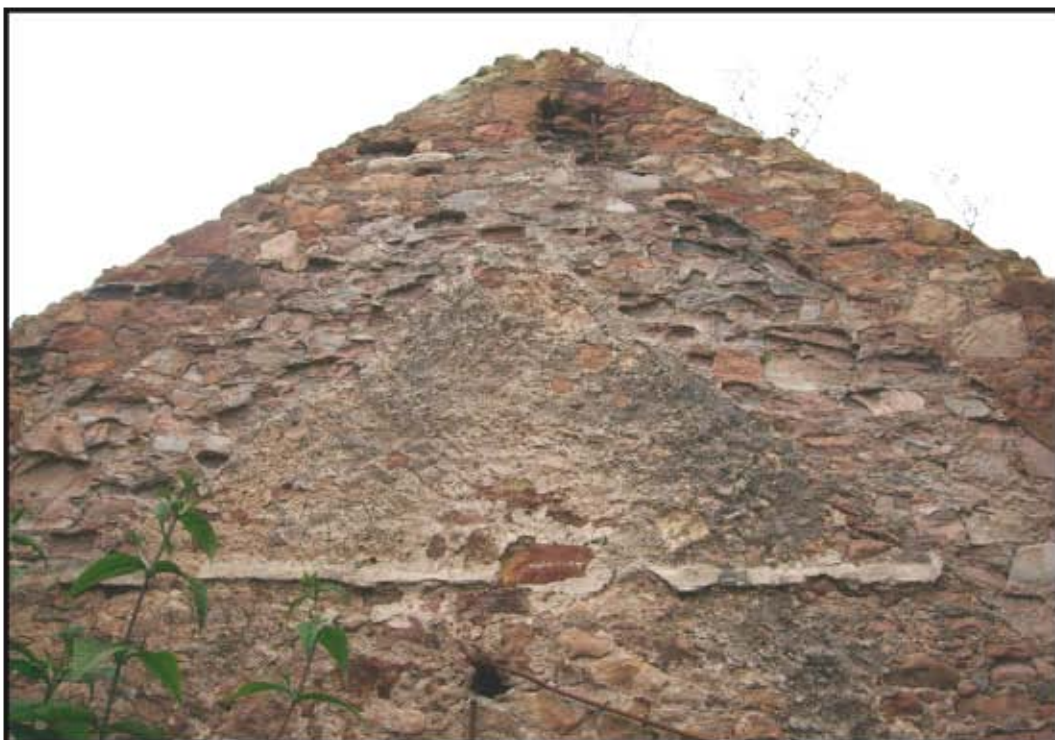
Plate 8: Detail of an earlier roof line on the interior west gable wall of Building B
