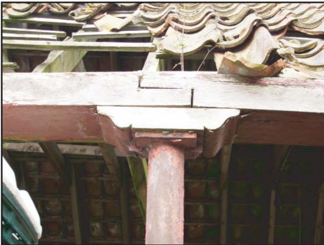
Plate 12: Detail of the cast-iron column head supporting a sill beam for the rafters of Building D from the east
