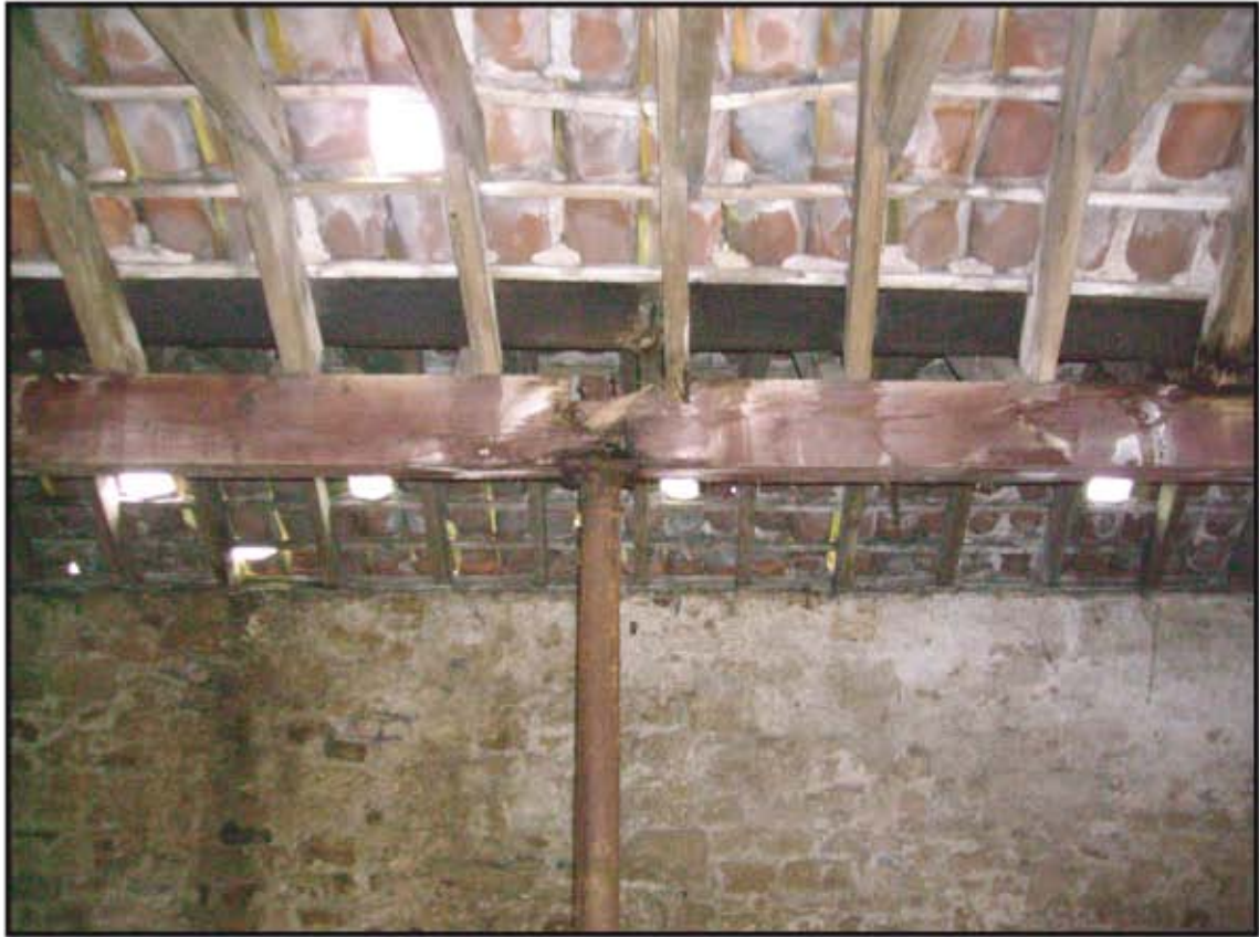
Plate 21: Detail of the cast-iron column supported in the east/west roof beam in Building F from the south
