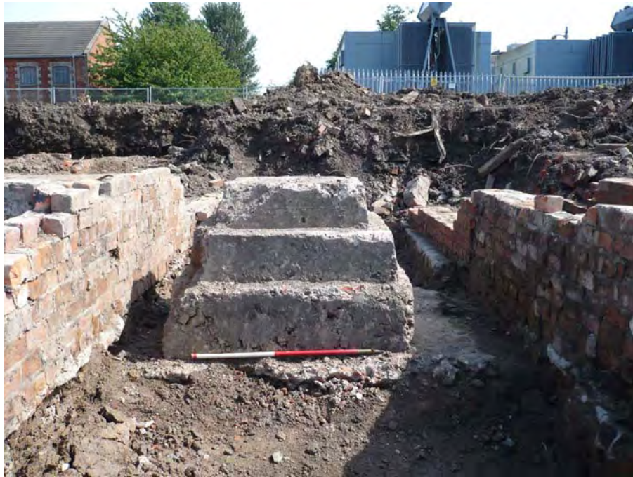
Figure 8: Detail of concrete foundation [003]
