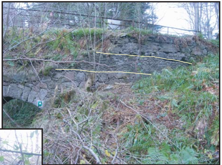
Plate 5: Detail of the stone phasing on the east side of the south elevation (highlighted)
