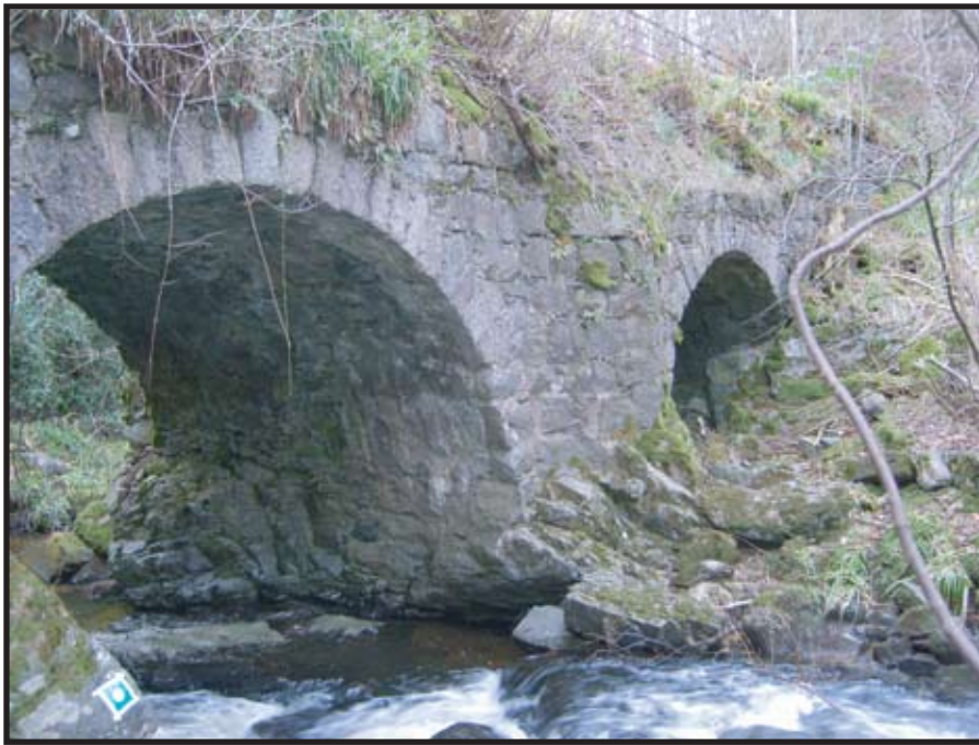
Plate 4: View of south elevation of Sheeoch Bridge showing the projecting buttress between the arches.
