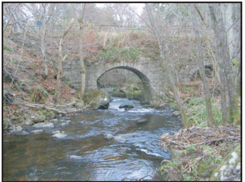
Plate 2: General view of south elevation of Sheeoch Bridge showing the collapsed spandrel
