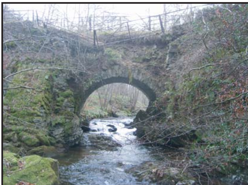
Plate 3: General view of the main arch of the north elevation showing the collapse on this side
