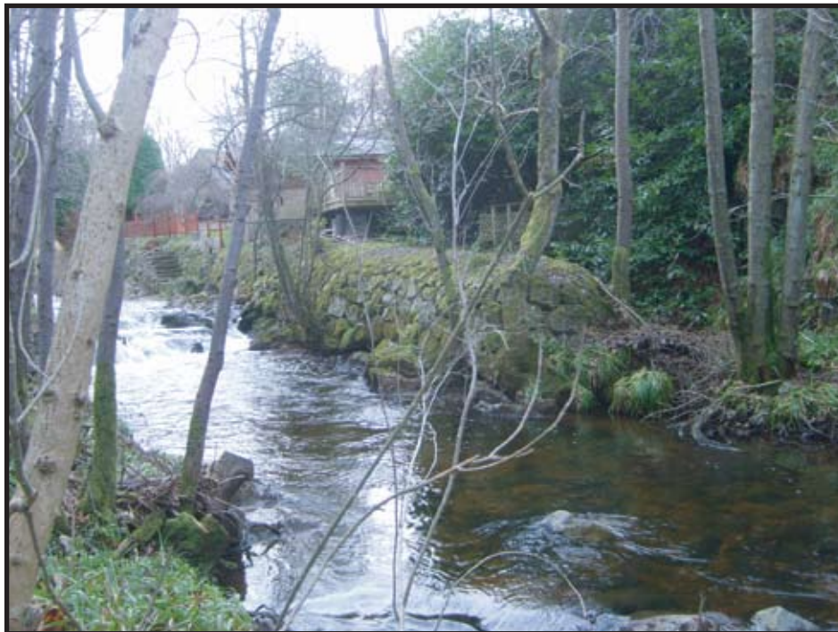
Plate 14: Stone boulder wall of mill lade (F22) to south of bridge
