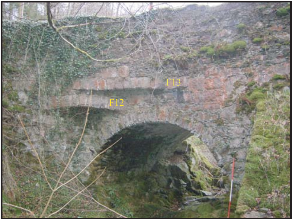
Plate 7: View of storm arch (F9) showing the stone relieving courses (F12 & F13) above plus the stone phasing.
