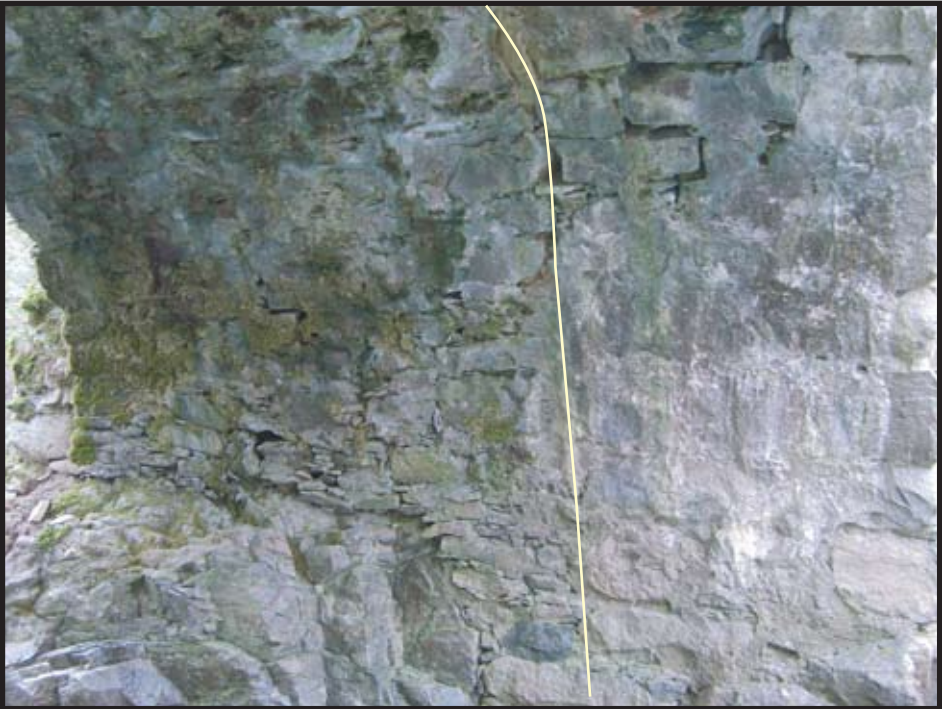
Plate 8: Detail of the construction line in the soffit of the storm arch (shown highlighted)
