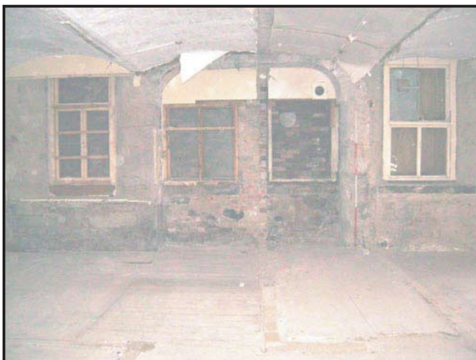
Plate 21: Bricked-up cart entrance F0/6 on the south wall of the ground floor showing the inserted windows
