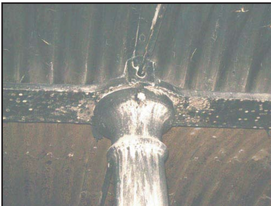
Plate 30: Detail of the top section of the cast-iron column in the second floor
