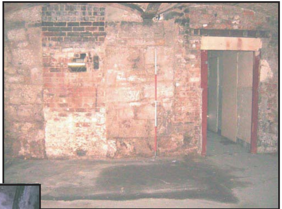
Plate 17: Detail of bricked up wall (F-1/12) on the south wall
