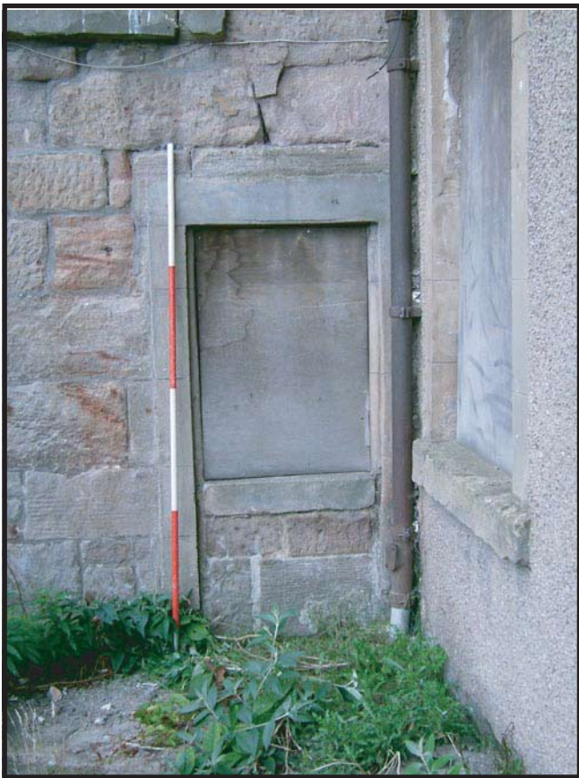
Plate 7: Detail of the modified window on the west side of the main staircase
