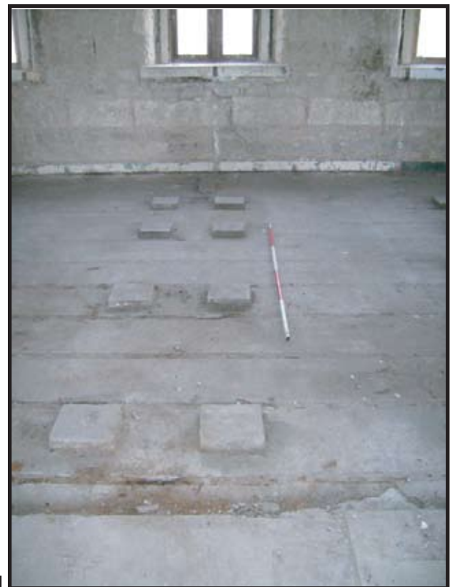
Plate 32: Detail of machine plinths on the third floor
