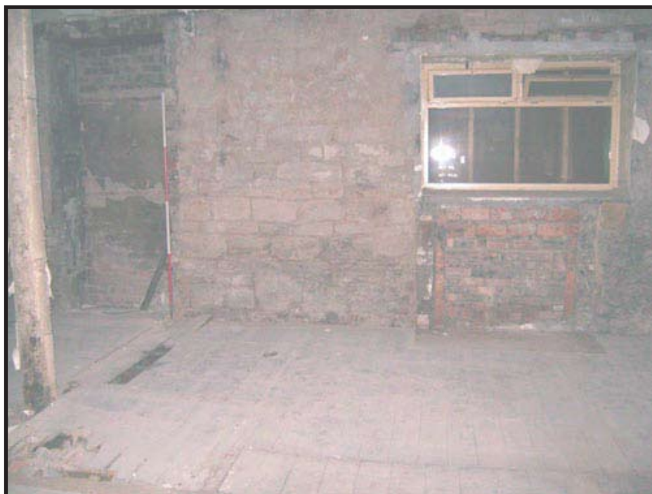
Plate 20: East wall of the ground floor showing features F0/4 window with F0/7 fireplace below and F0/3 doorway
