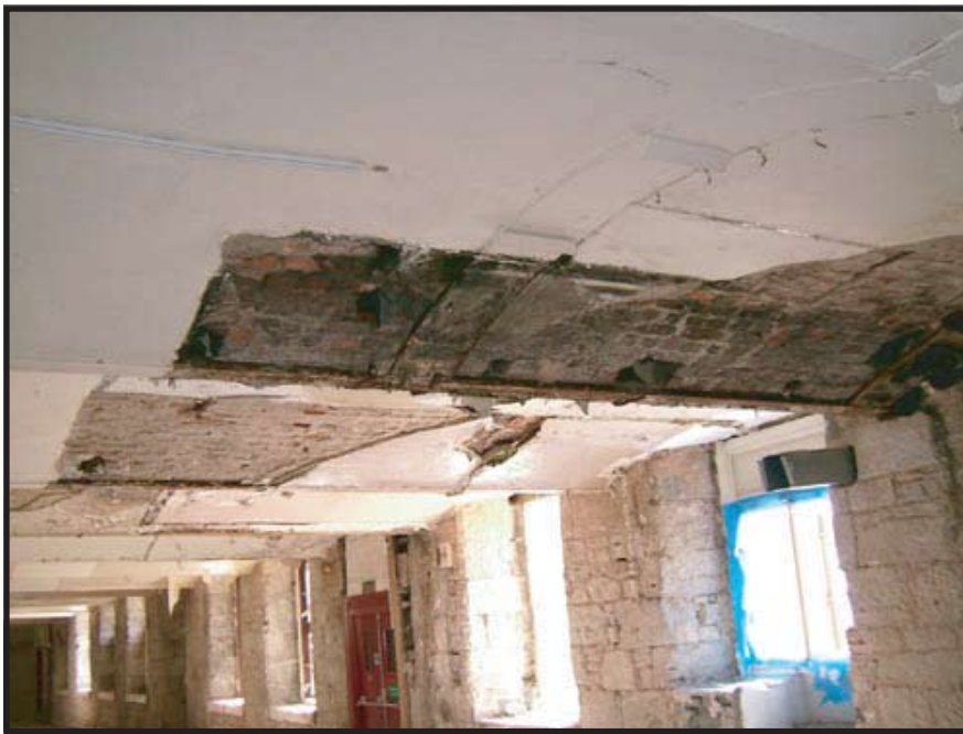
Plate 25: Detail of the brick-vaulting on the ceiling of the first floor
