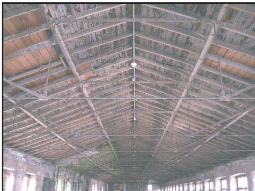
Plate 39: Detail of the steel-framed roof on the fifth floor
