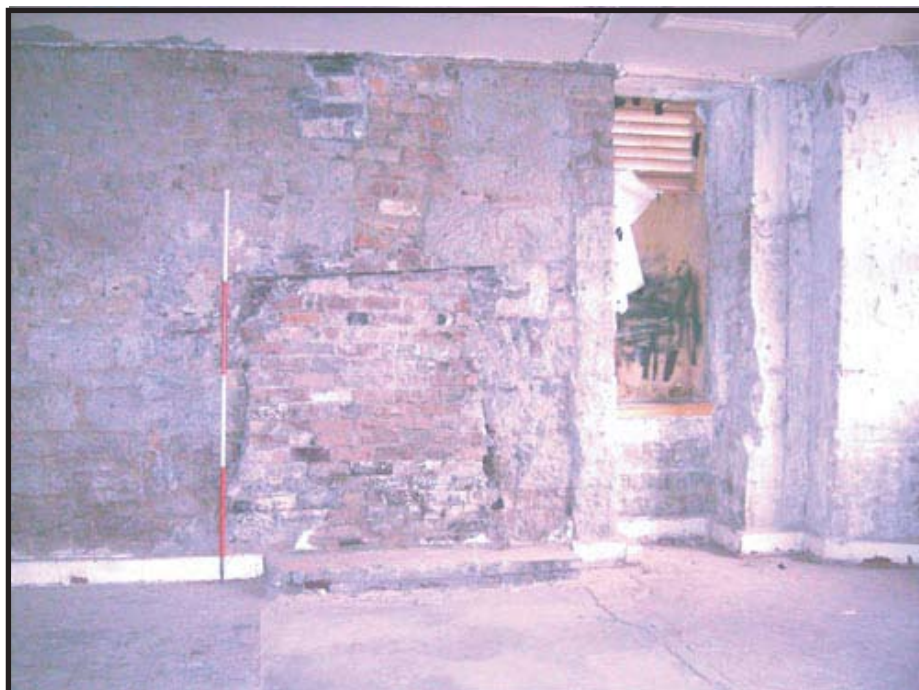
Plate 22: Detail of the north side of the west wall showing features F0/17 (window recess) and F0/18 (fireplace) on the ground floor
