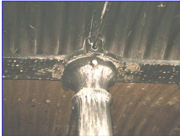
Detail of the top of a cast-iron column on the second floor
