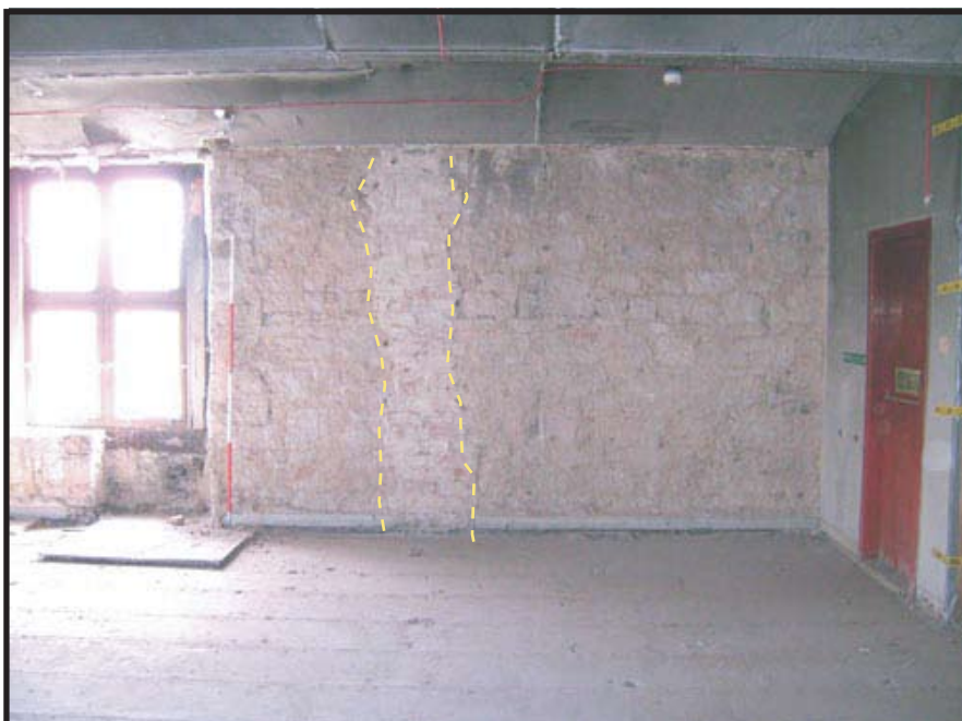
Plate 27: General view of the north side of the west wall showing the brick flue (F1/2)
