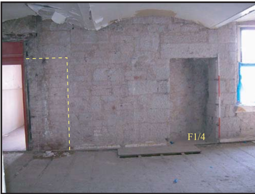
Plate 28: Detail of the bricked-up doorway F1/3 and opening F1/14 on the south wall of the first floor
