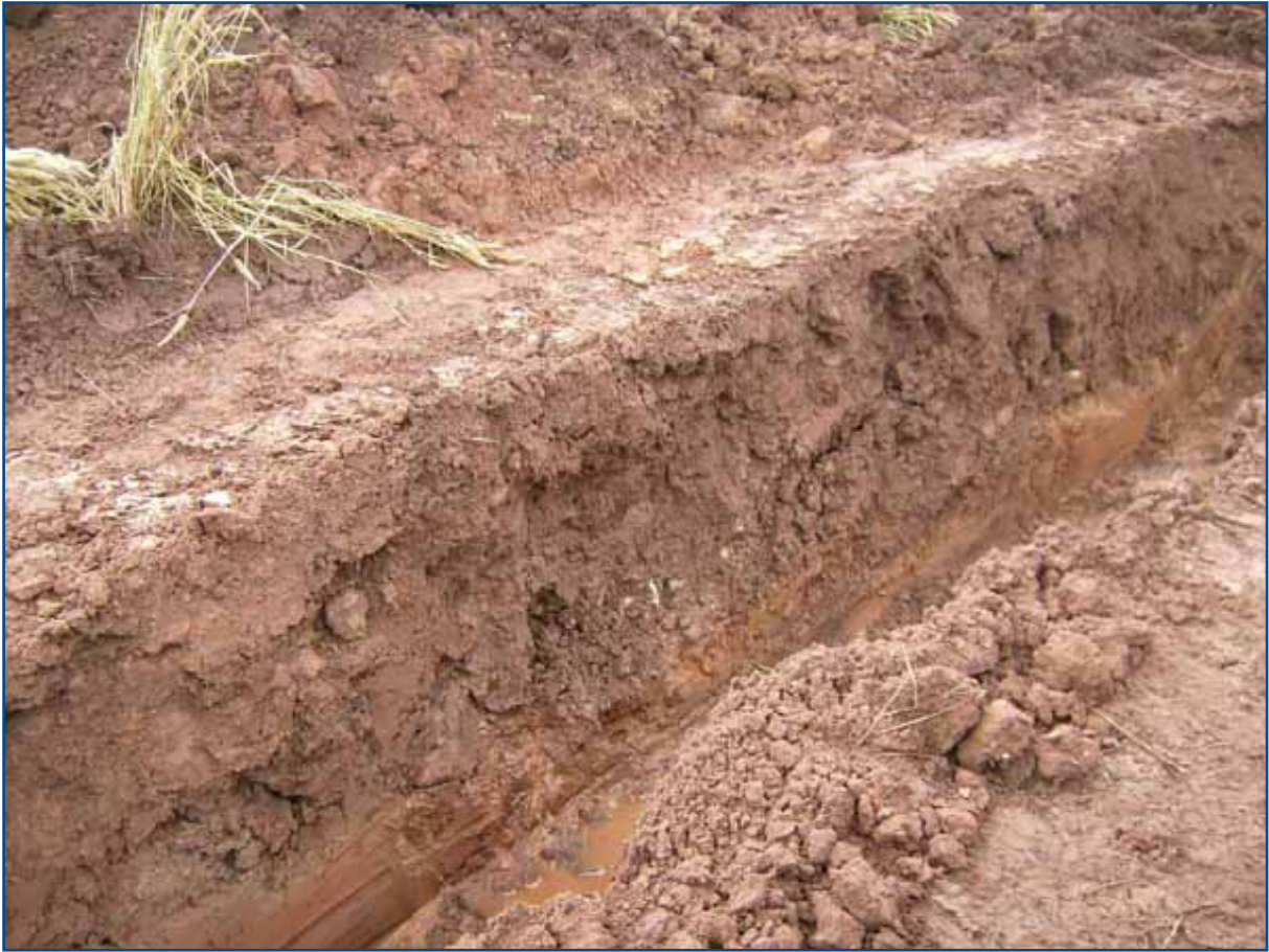
Plate 7: Detail of the cable trench at Site 3 showing the alluvial deposits
