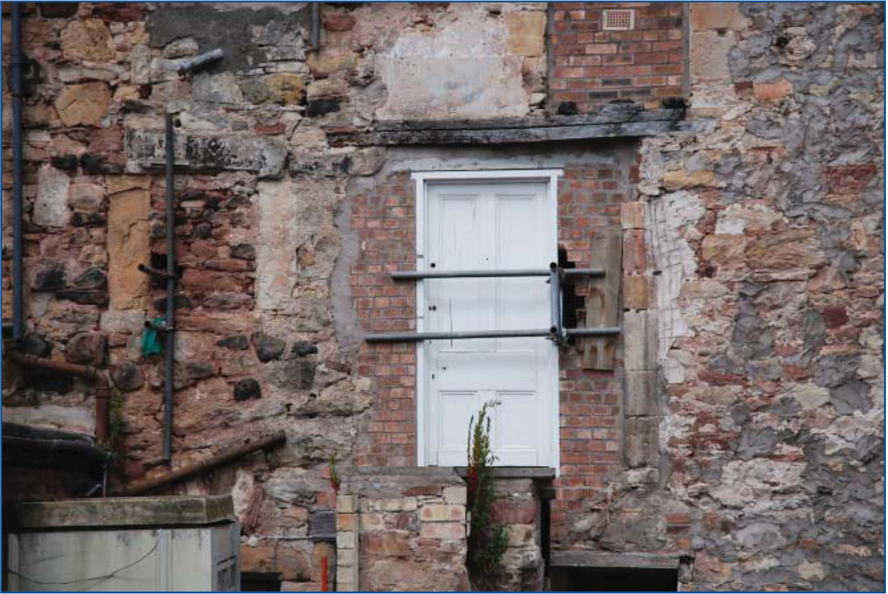
Plate 5: Detail for the first floor altered doorway to the east of the south elevation
