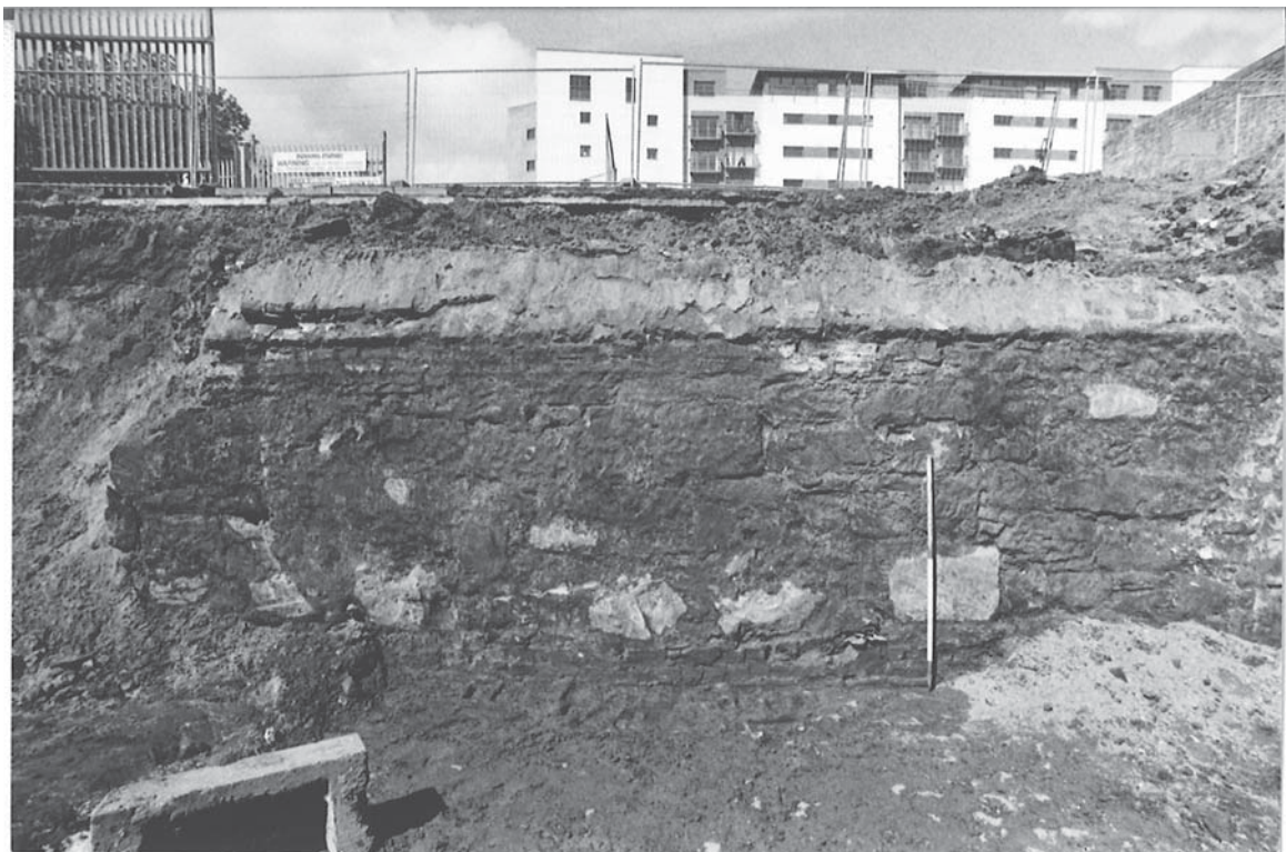
Plate 2 :Brickwork underpinning on north wall
