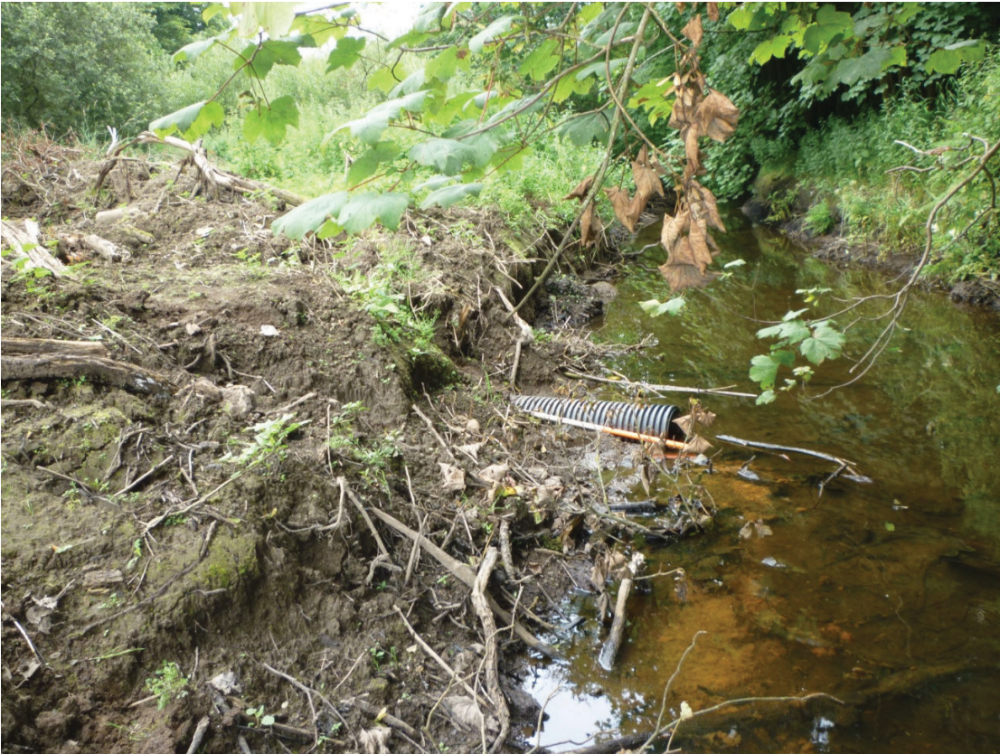
Figure 4: Outflow of the run-off trench
