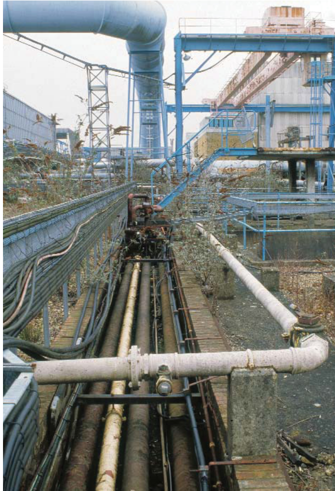
Fig 19 Fuel pipes and other pipes laid in an open conduit forming a 'safety zone', looking west between Cells 3 and 4 (MoLAS 021/05/14)
