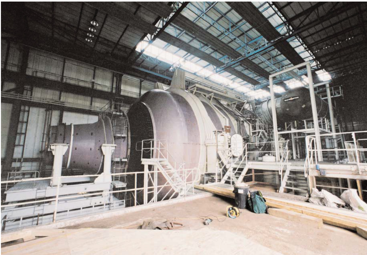
Fig 50 Cell 4 plenum chamber, looking south-west. The intake has been disconnected, to the left (CNV00011-F2-07.jpg)
