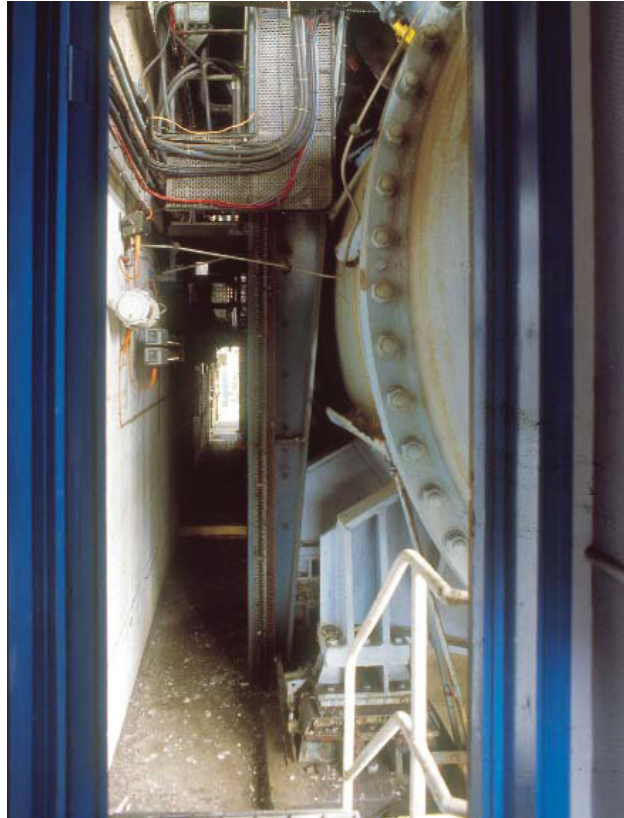
Fig 37 Gap between Cell 2 (right) and control room (left), looking north, showing the mountings for the test cell separate from the steel frame for the shelter overhead (MoLAS 021/05/33)
