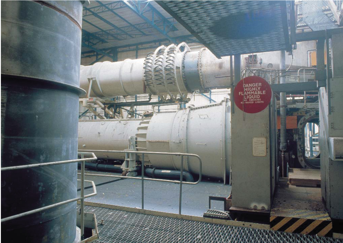
Fig 53 Engine capsule in Cell 4, leading to the main exhaust diffuser (to left), and upper spill duct above, looking north. The diffuser can be unbolted and rolled sideways to install and dismantle engines. Note water spray pipes entering the spill duct (MoLAS 028/05/40)
