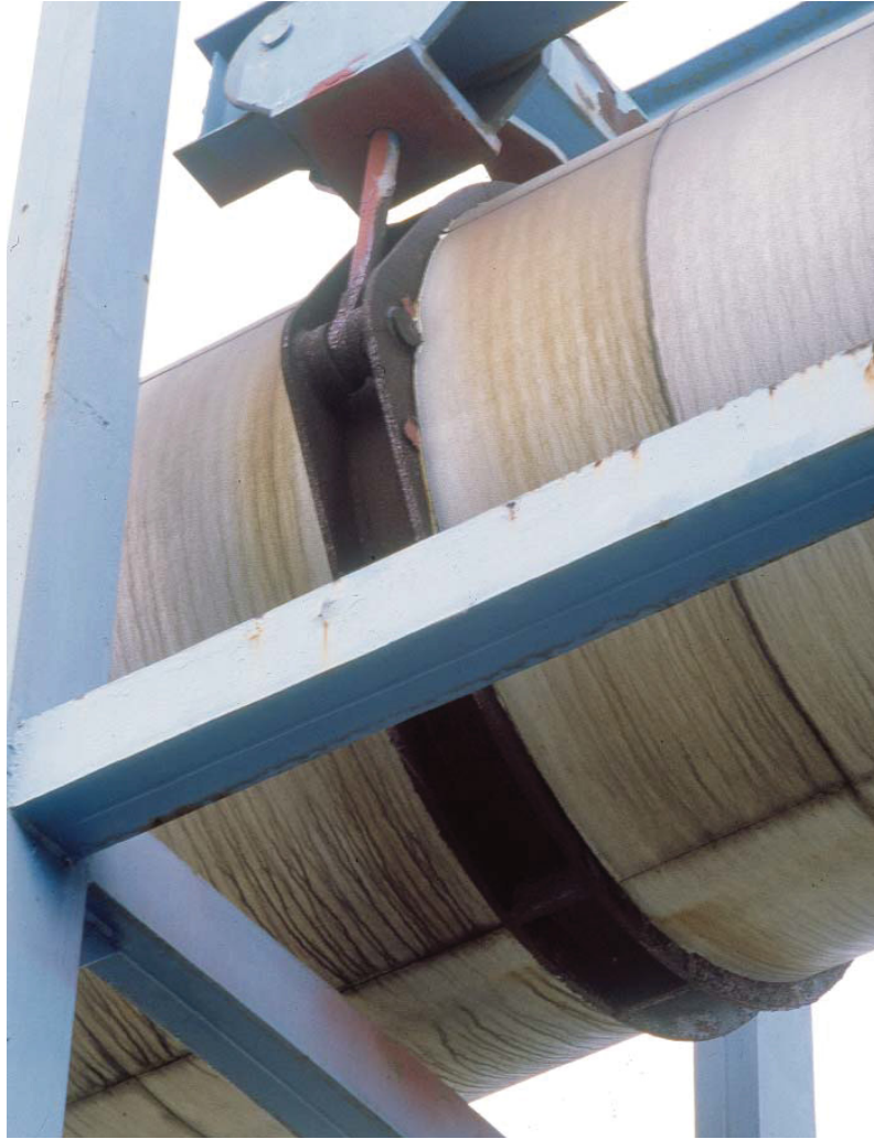
Fig 15 Flexible support for overhead air pipe near Cells 1 and 2 (MoLAS 021/05/20)
