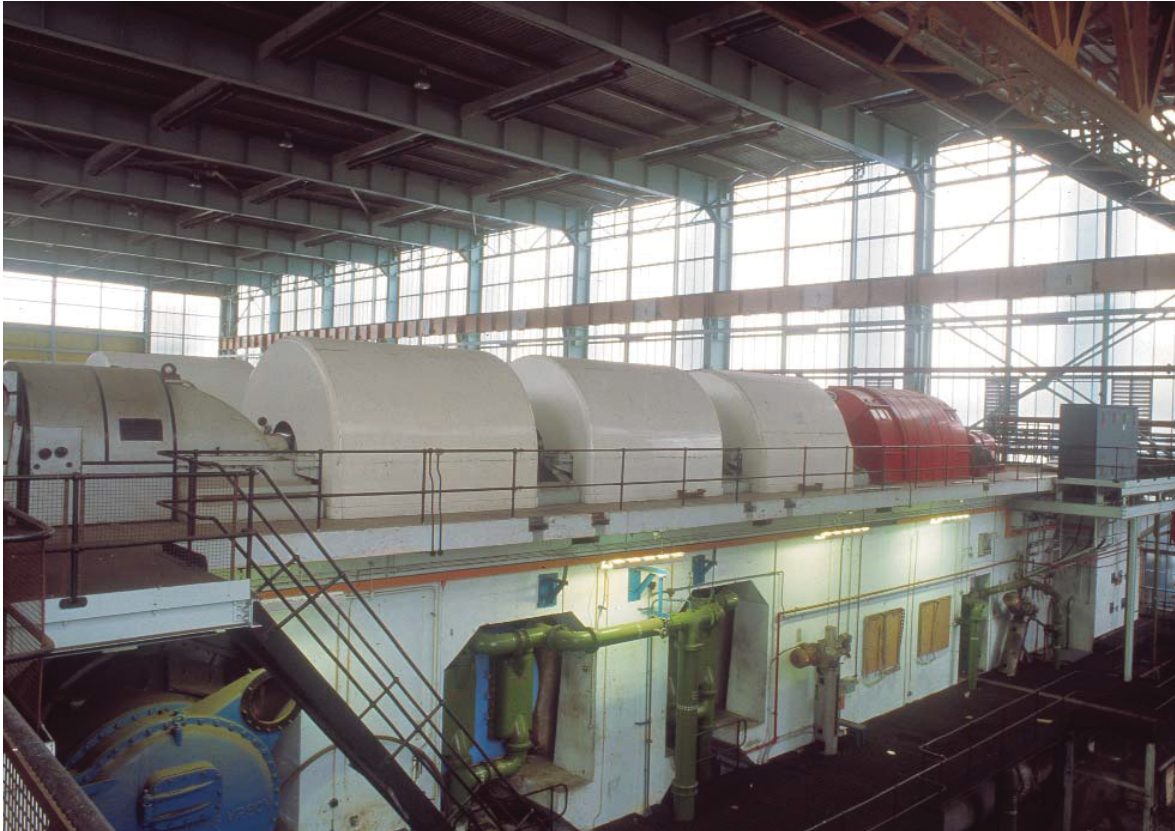
Fig 8 Interior of the Air House, looking north-east, showing the southernmost set of air compressors at an upper level inside the building. Service piping and machinery is underneath at ground level. The space in the foreground is a loading bay (MoLAS 015/05/02)
