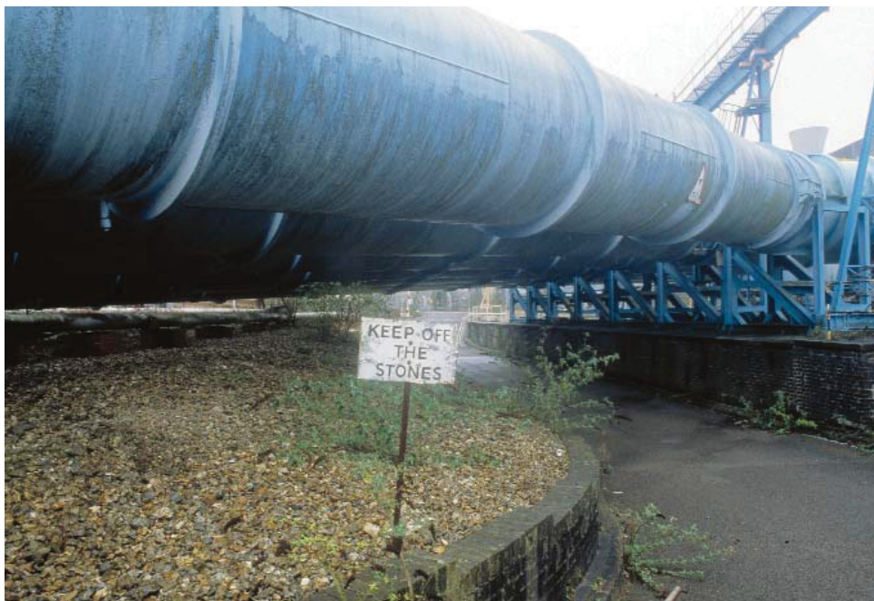
Fig 47 A series of air pipes running overhead from the west end of Cell 4 towards the Air House, looking north-west. Large areas of the site are gravelled and possibly sprayed with weed killer, presumably to minimise maintenance (MoLAS 028/05/26)
