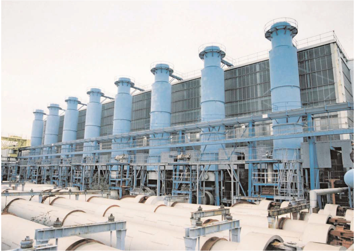
Fig 7 Exterior of the Air House (Bldg 621), looking west. Each of the eight vertical exhaust stacks serves one of the sets of air compressors inside the building (CNV00025-F1-24.jpg)
