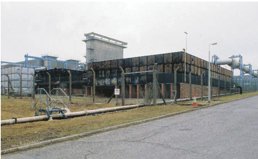
Fig 20 Water tanks north-east of Cells 1 and 2, to store water for cooling; looking south-west. Note water-level gauge on the nearest corner (MoLAS 021/05/10)
