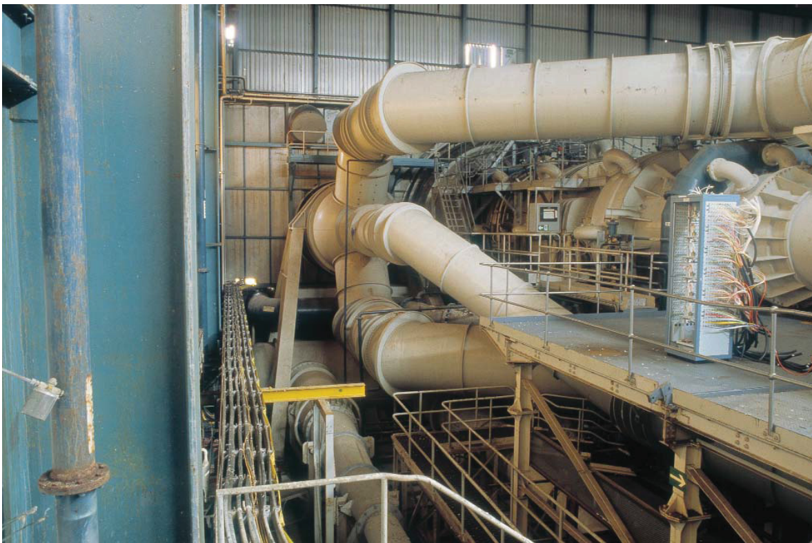
Fig 54 Spill ducts and exhaust diffusers leading to cooling stages in Cell 4, looking north-west (MoLAS 028/05/47)
