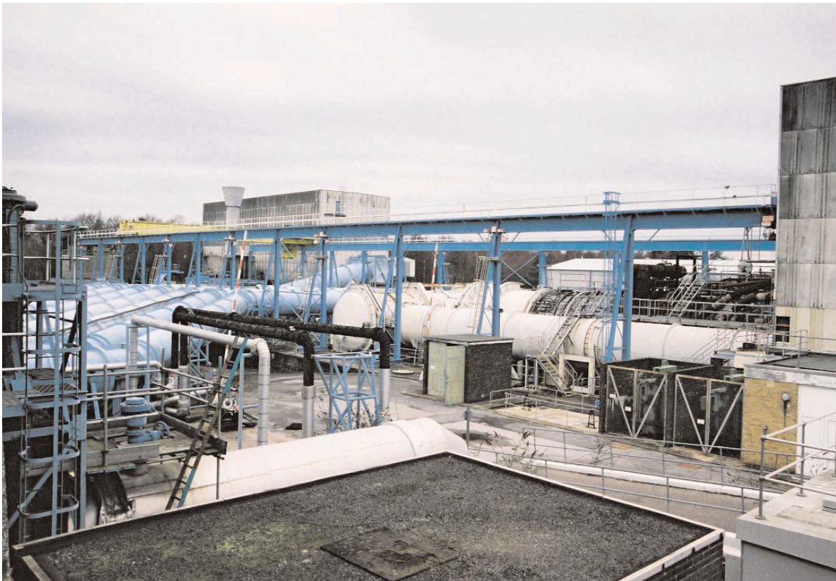
Fig 45 Air pipes at the west end of Cell 4, looking north-west. The cell's outlet pipes (white) are mainly at a low level, connecting with overhead pipes (blue) to the Air House (CNV00008-F5-08)
