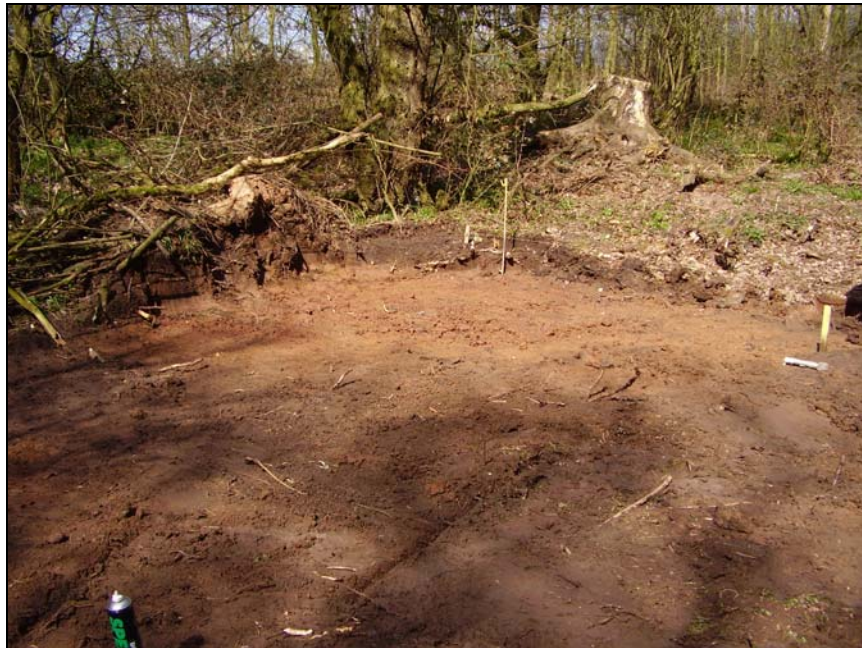
Fig. 3 Northwest corner of the larger 'base' area where the greatest depth of topsoil was stripped to make up the eastern end.
