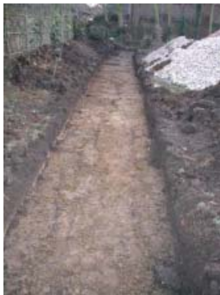
Plate 1 Trench 1 viewed from the north
