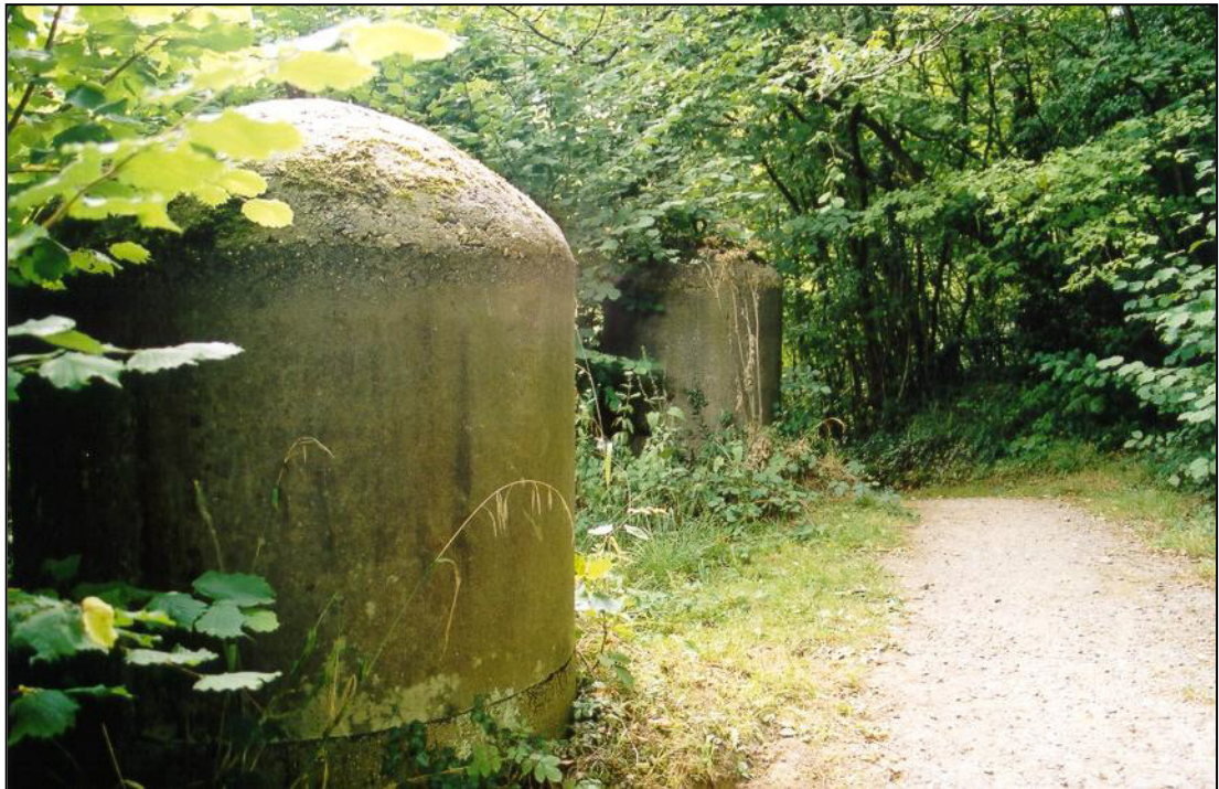
Fig. 16 - UORN 16752: anti-tank cylinders by the towpath of the Basingstoke Canal opposite Coxmoor Wood. They are three feet in diameter and stand five feet high.
