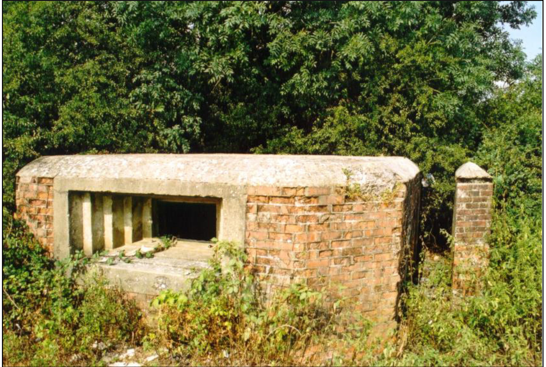
Fig. 13 - UORN 6974: the exterior of the Vickers machine gun emplacement shows its massive main embrasure. Another example of this type of emplacement further north-west has three such embrasures making it probably unique [UORN 16698].
