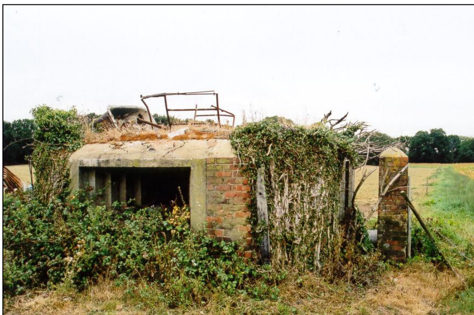
Fig. 7 - UORN 7414: Vickers machine gun emplacement with detached blast wall.
