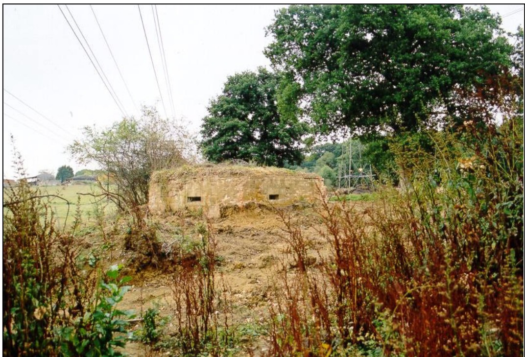
Fig. 10 - UORN 7411: type 24 pillbox with earth piled around, said to be from the spoil of the anti-tank ditch.
