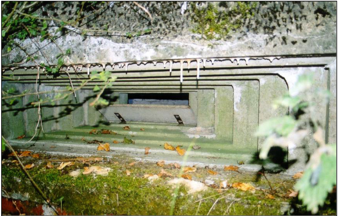
Fig. 14 - UORN 16698: a multi-stepped light machine gun embrasure with hinged asbestos shutter still in place.
