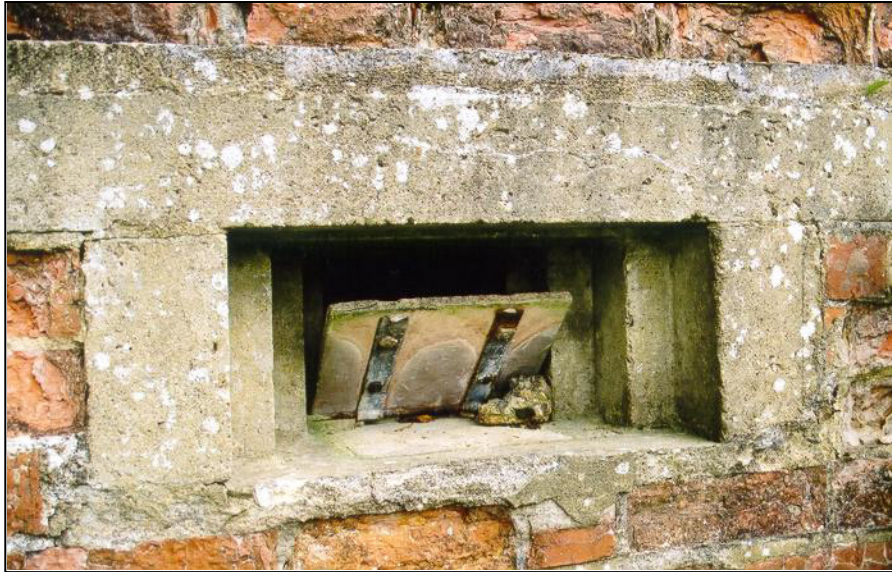
Fig. 11 - UORN 7412: Shutter to a light machine gun embrasure of a type 24 pillbox that can still be opened and shut.
