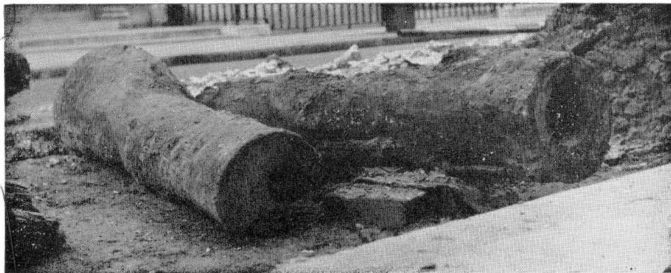
Wooden water pipes in Carlos Place, W.1.
