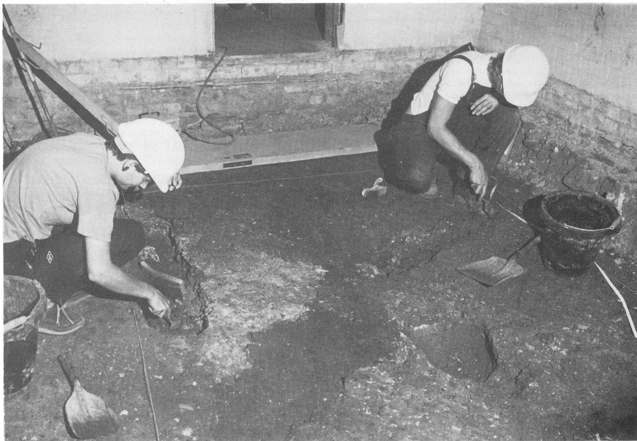
Fig. 2: Excavation in progress beneath the strong room floor in the standing building.
