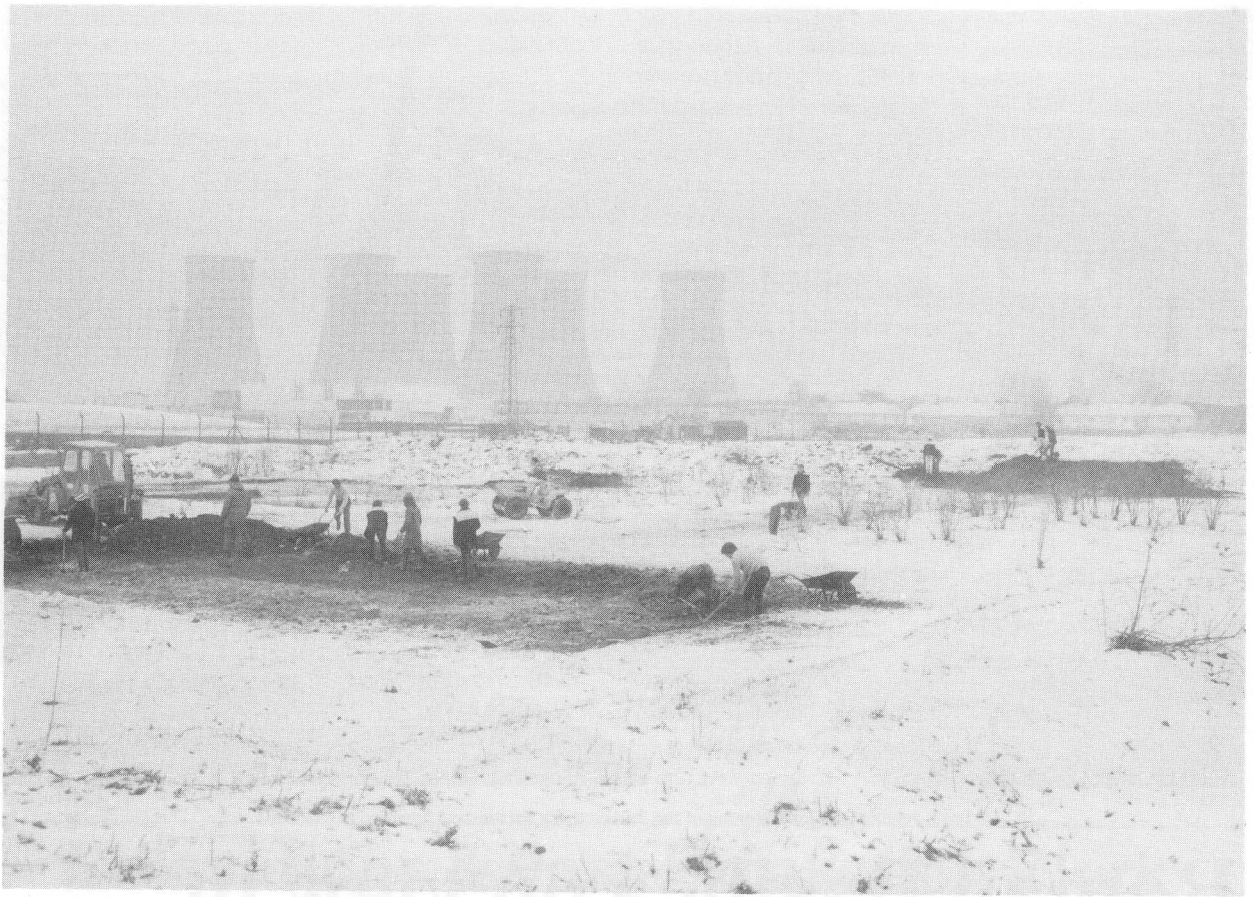
Fig. 1: extending the excavation area, January 1985.
