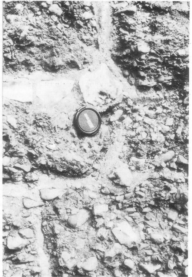
Fig. 3: close-up of ferricrete blocks in St Peter and St Paul, Harlington. Angular flints, gravel-stone blocks of subangular flint pebbles bonded in a rusty-red matrix. Gravel-stone variety of ferricrete. (Lens cap is 50mm in diameter).
