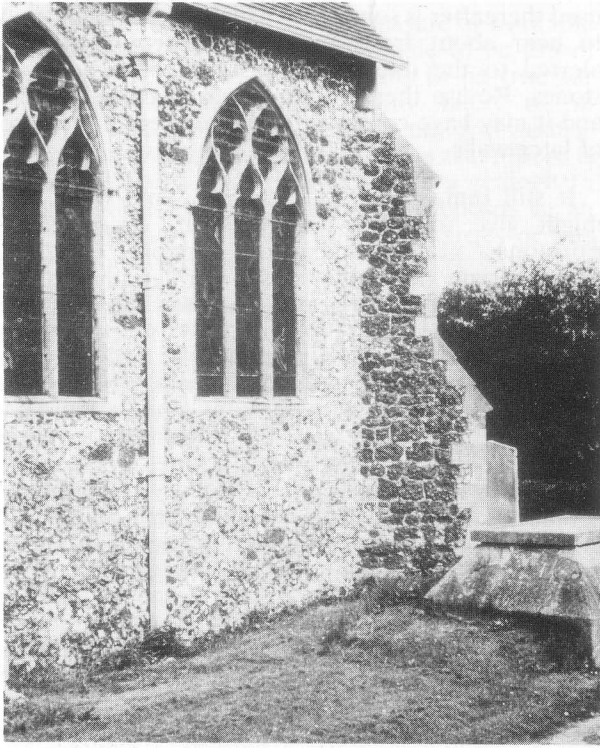
Fig. 2: south-east buttress, St Peter and St Paul, Harlington, showing blocks or ferricrete (the dark blocks).
